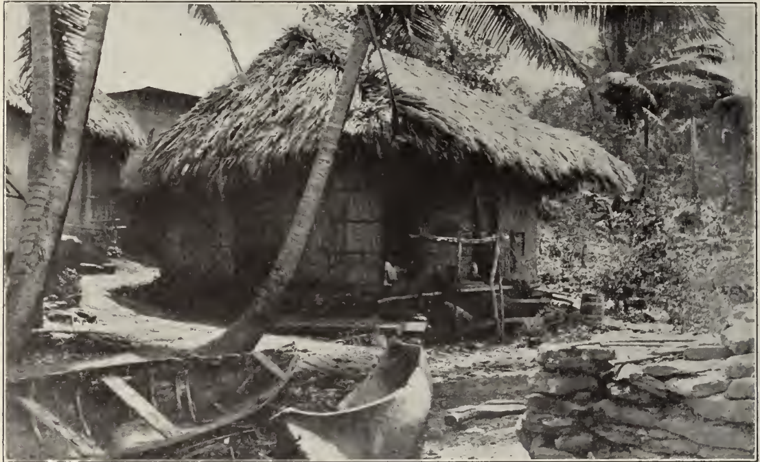
The usual type of house of the average interior Panamanian. They are constructed of bamboo, tied by means of withes and have a thatch roof.
