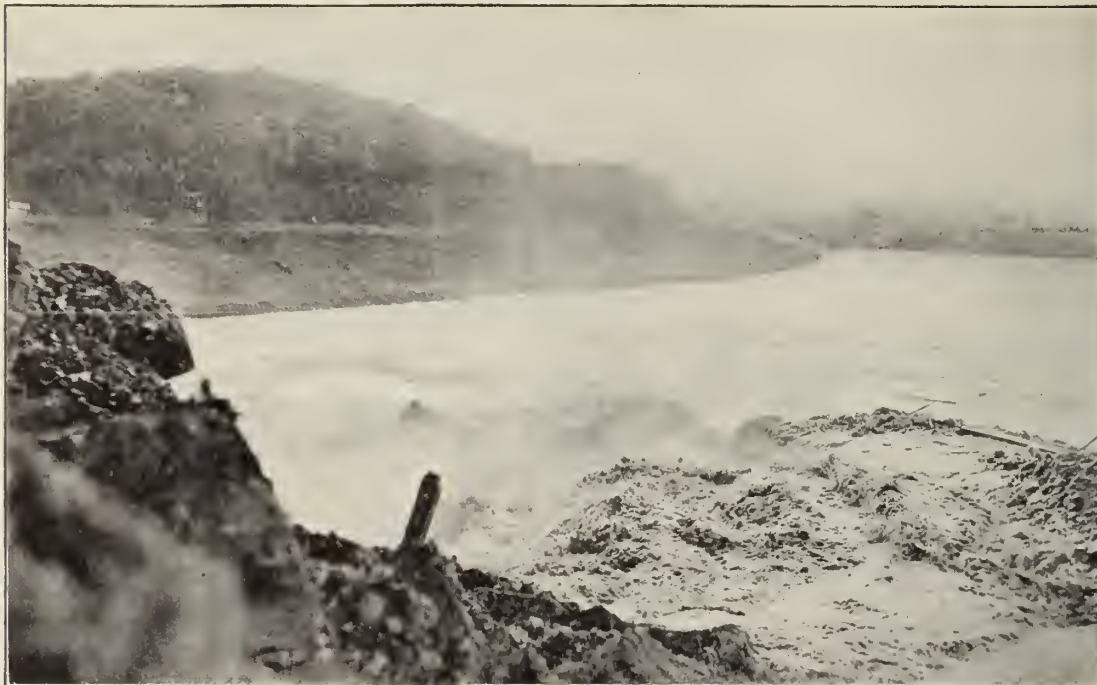
View looking into the pit toward Miraflores Locks.
