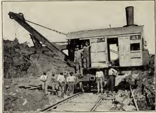
Revolving steam shovel. A few of these machines were used to advantage, but larger ones were used for the heavy work.
