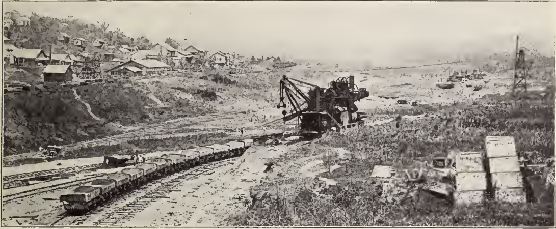
Canal between Empire and Culebra, showing the French method of excavation, in 1888.
