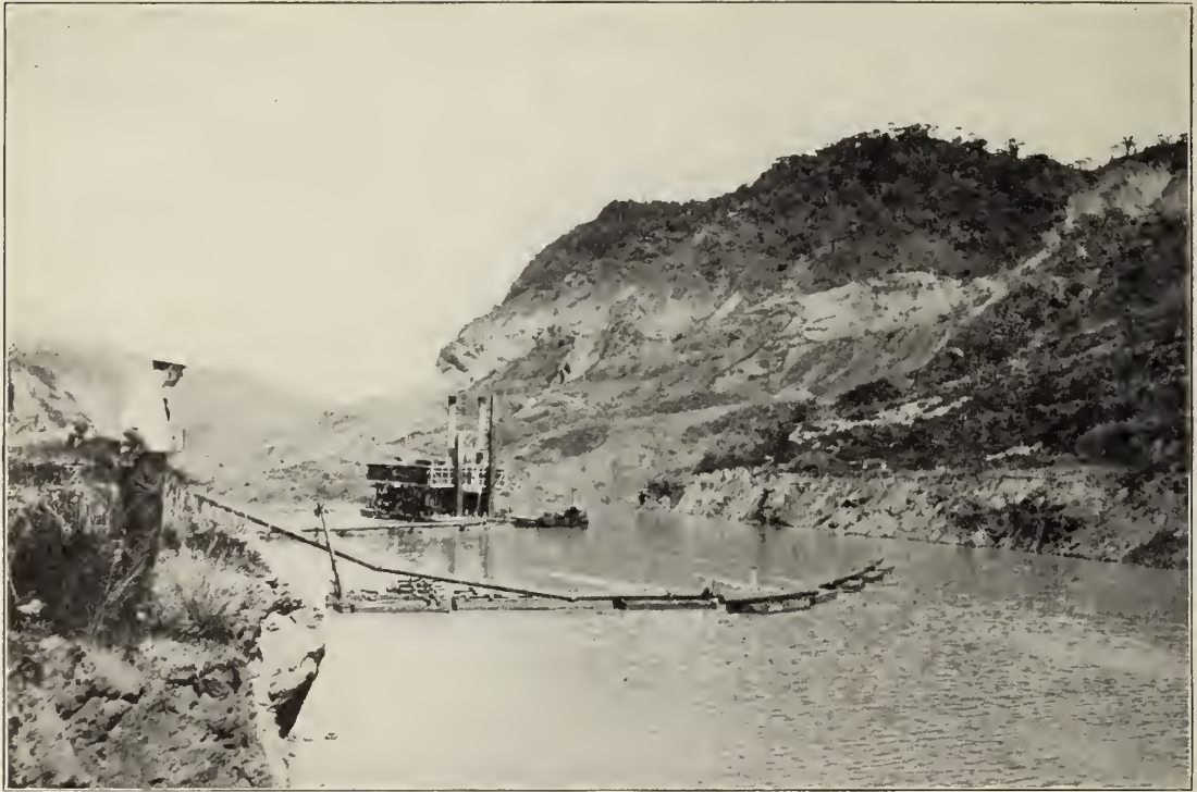
Dredge No. 85 working at the south toe of Cucaracha slide.
