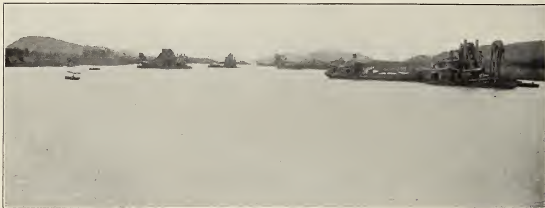
Dredges excavating in the Pacific Channel from Miraflores to the sea.
