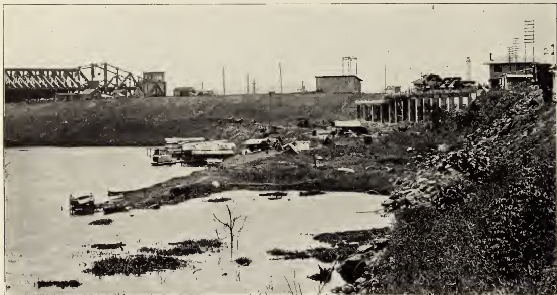
Boat landing at Gatun. The structure on concrete piles to the right is a wharf where small boats that ply the lake may land their cargoes, when the lake is to its full height.
