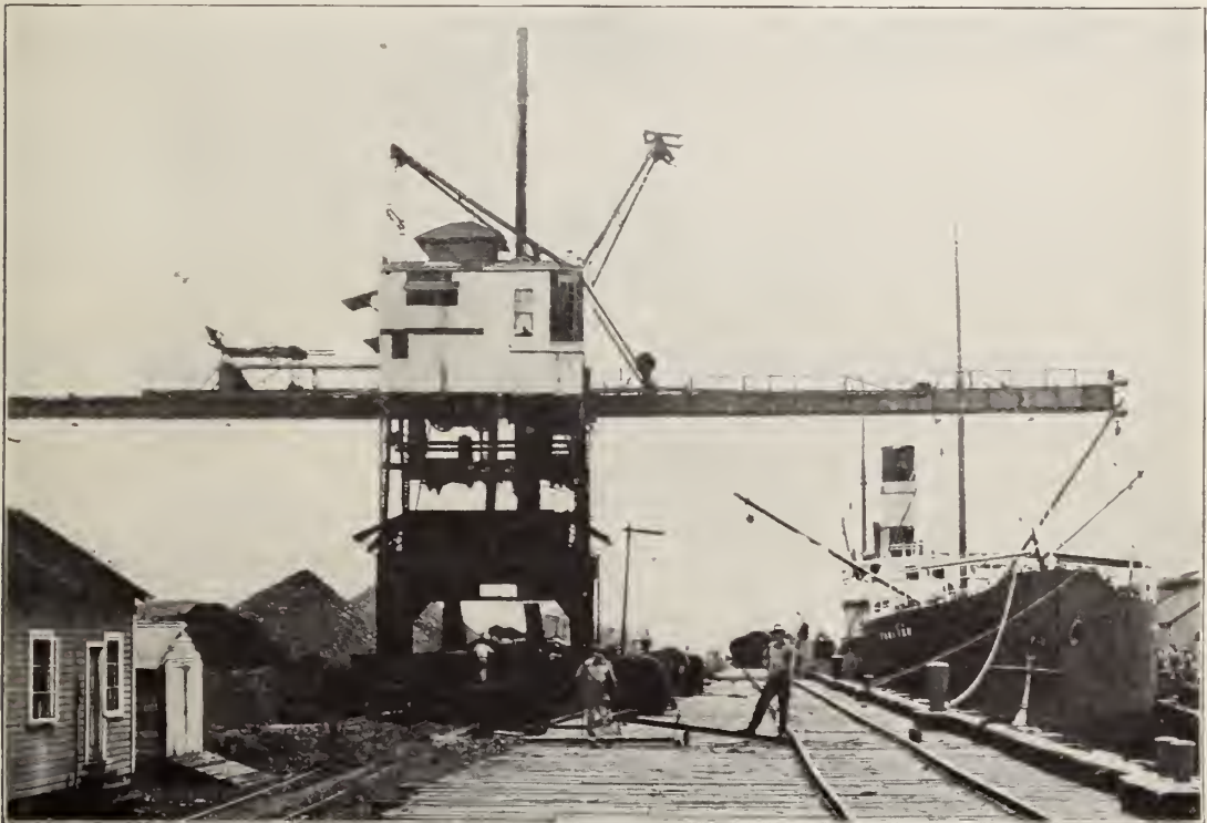
Telpher plant, which has handled practically all of the coal used in the Canal work.
