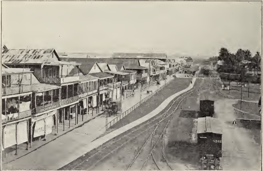
Front Street, Colon, as it appears to-day. Before the Americans started work on the Canal, many of the streets were in an unsightly and consequently unhealthy condition. In the past few years a large amount of street improvements have been made and much land has been filled in and reclaimed east of the city. All of the streets, both residential and business, are now macadamized.
