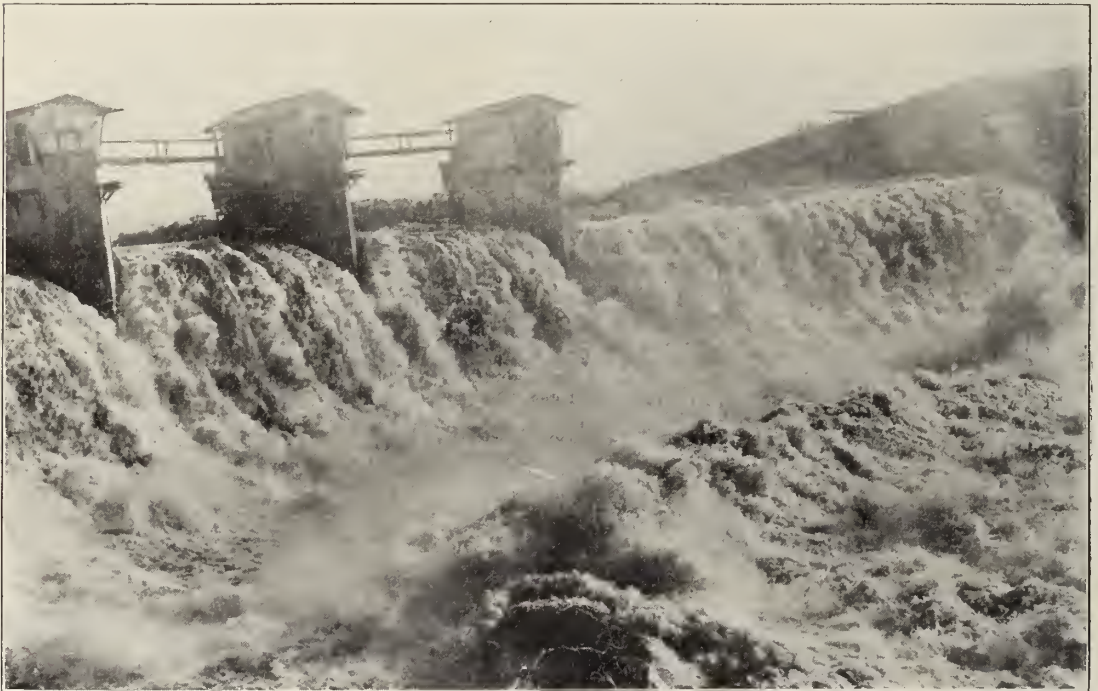
Water from the lake flowing over the spillway, during the rainy season, before it was completed. The spillway will control the rise and fall of Gatun Lake.
