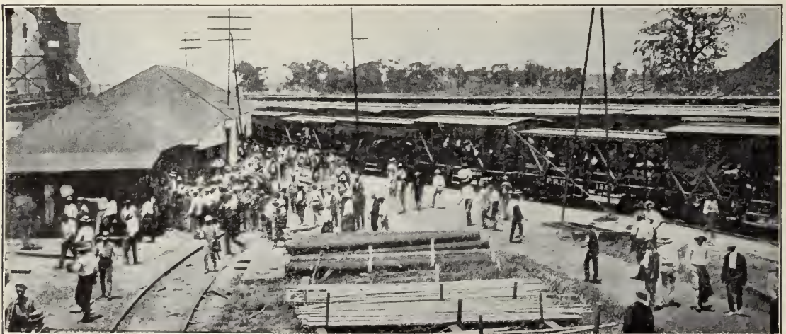
Labor train arriving at dry dock, Cristobal. A great many employes live at a distance from their work, and are transported to and from their homes in labor trains.
