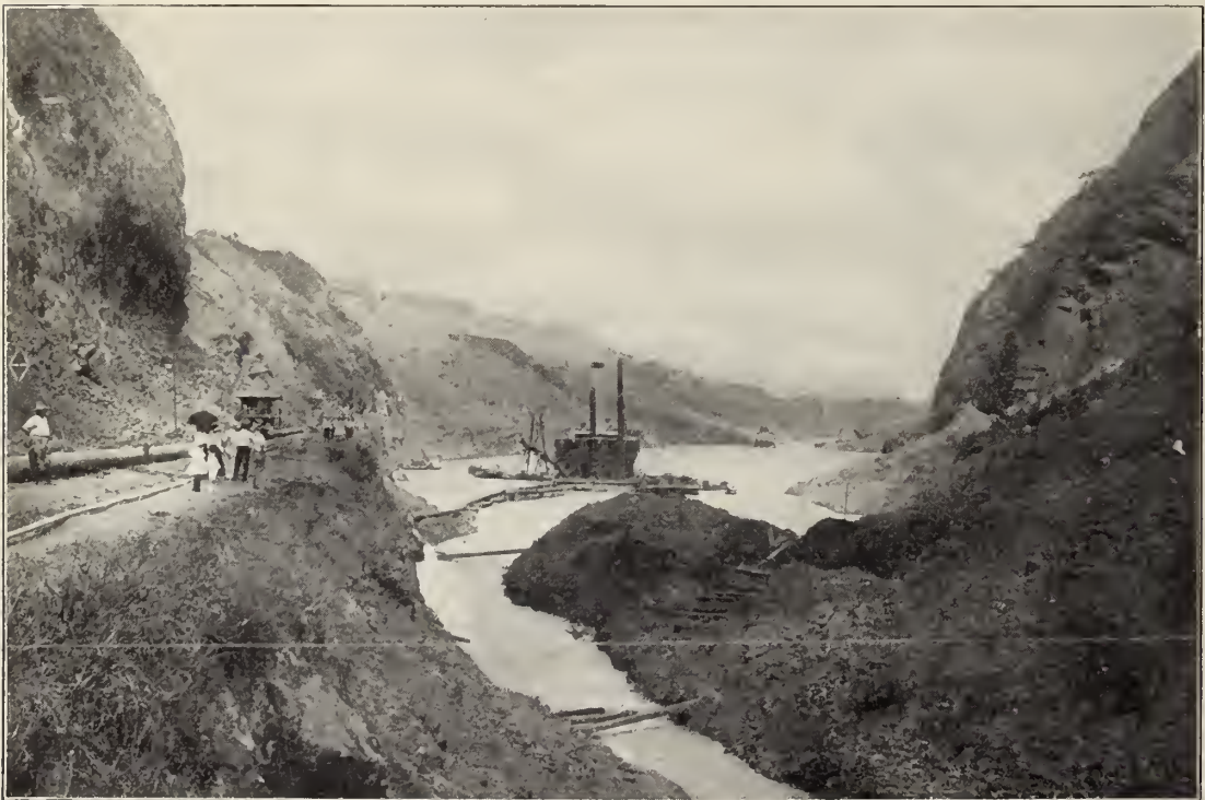
Looking north at a point about opposite the middle of Cucaracha slide, showing dredge No. 86 at work on the north toe of the slide.
