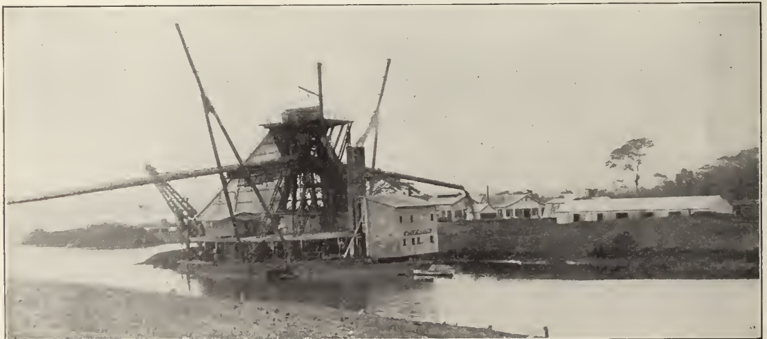
The French suction dredges with the carrying pipes, were effective in excavating, but like their cableways, did not carry the spoil far enough.
