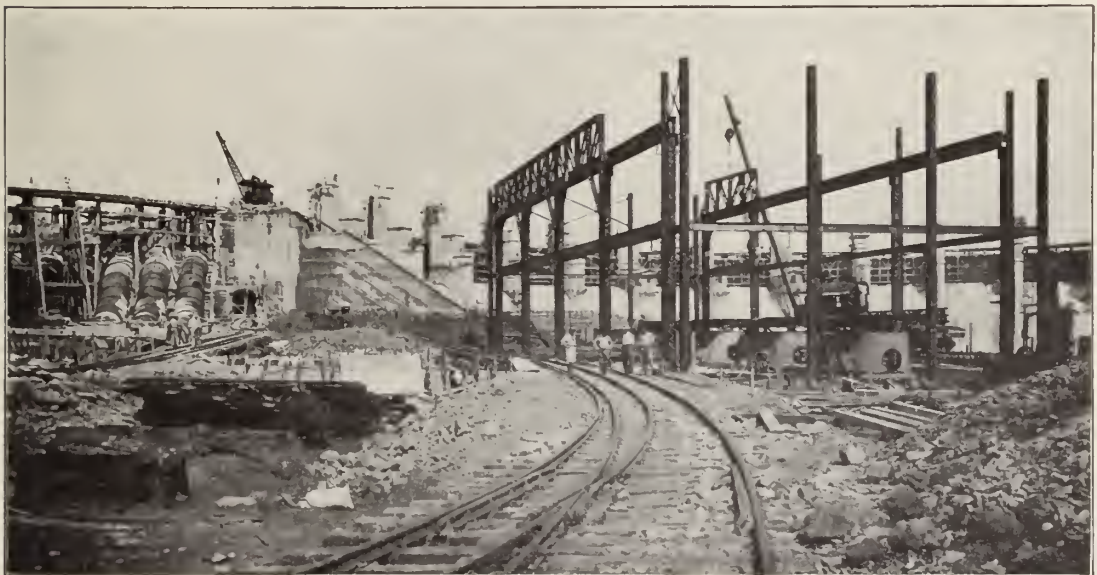
Hydroelectric station, Gatun spillway, under construction, showing location of penstocks.
