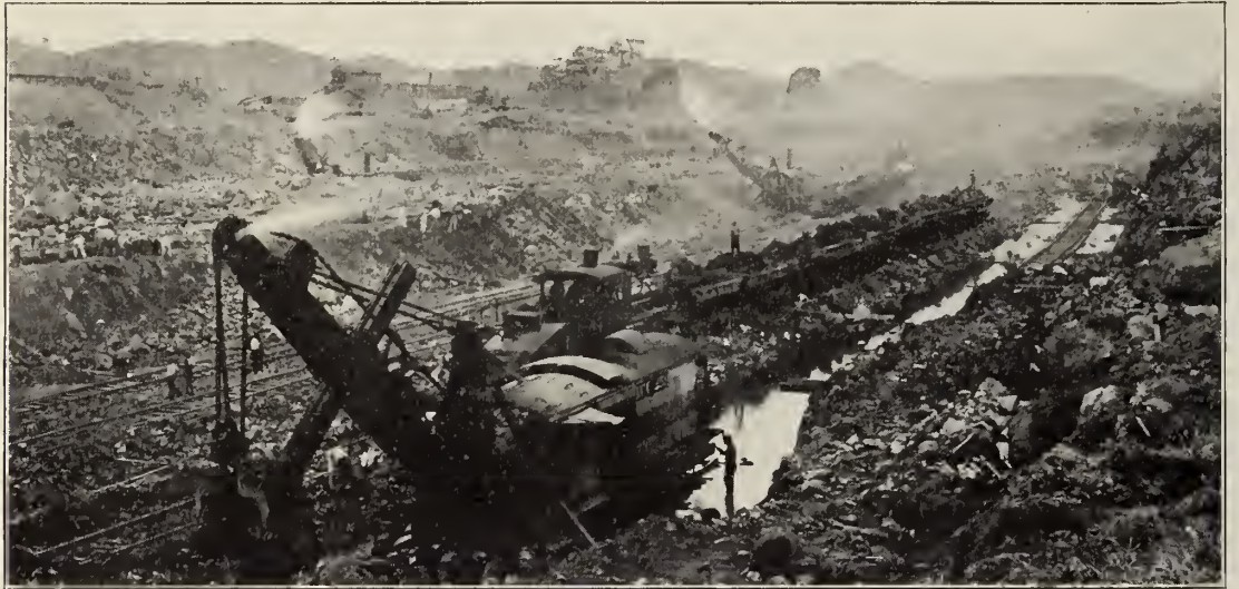
Excavating for lock site, Pedro Miguel.
