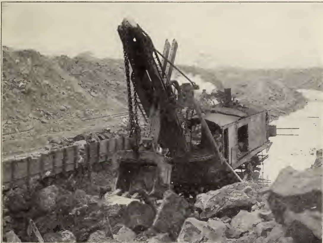
The American machine which moves mountains. One of the 100 steam shovels engaged in the Canal work, holding in its dipper a rock of many tons' weight. With the advent of these machines King Yardage became a household word in the Canal Zone. The American operators take a personal pride in their work, and the world's record for steam shovel excavation is said to be held on the Isthmus.
