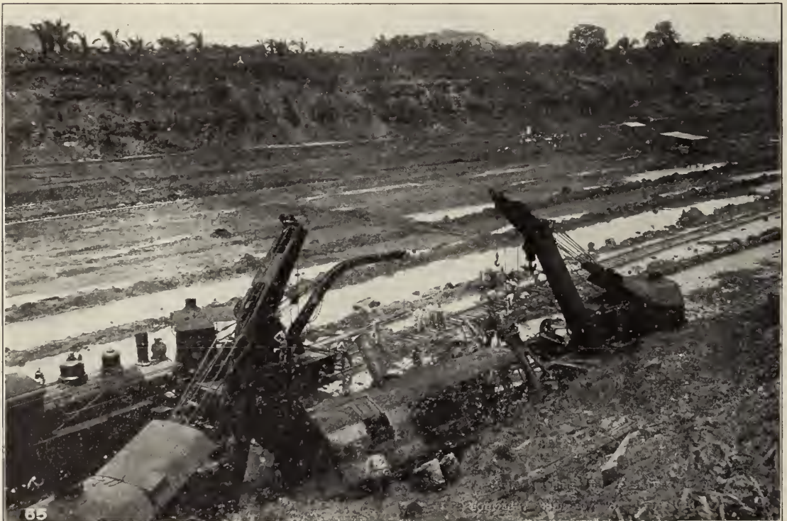
Two wrecking cranes picking up a steam shovel. These machines range in capacity from 15 to 100 tons, and are kept under steam day and night, ready for any emergency in the transportation service.
