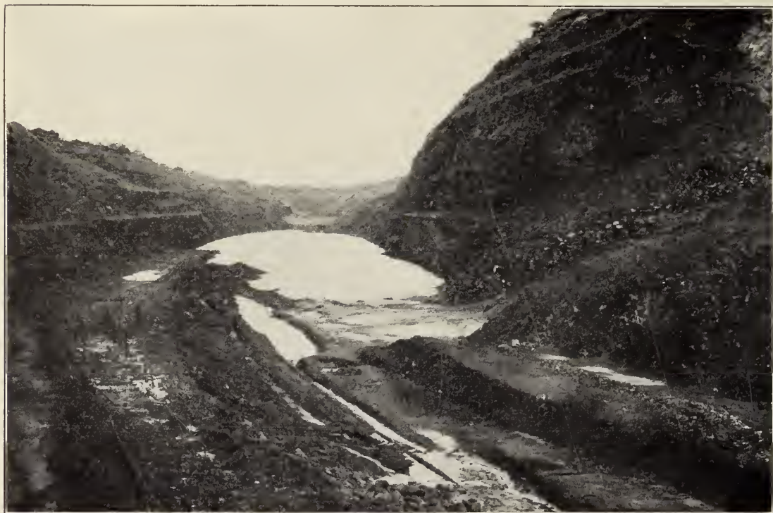
Culebra Cut between Gold and Contractor's Hills after the removal of construction tracks.
