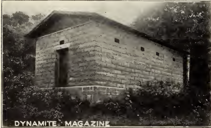
Twelve of these magazines for storing dynamite are located at convenient points along the Canal.
