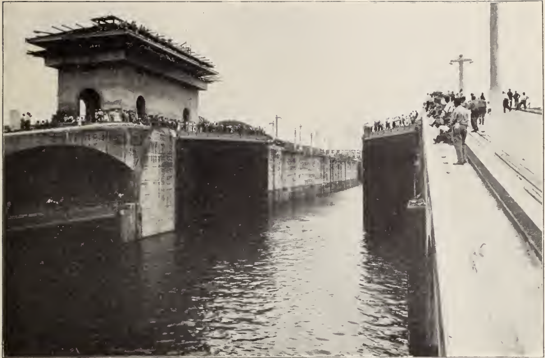
Opening the lower guard gate to admit the floating equipment.
