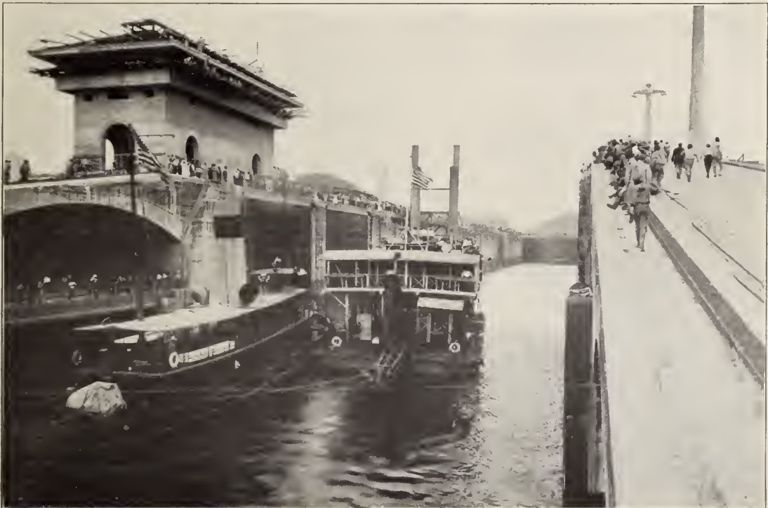
Tug Miraflores and dredge No. 85 entering the east lock chamber.
