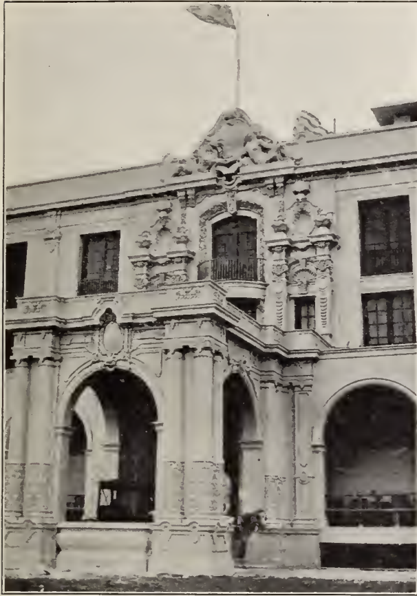
Main entrance to the new Hotel Washington, Colon.
