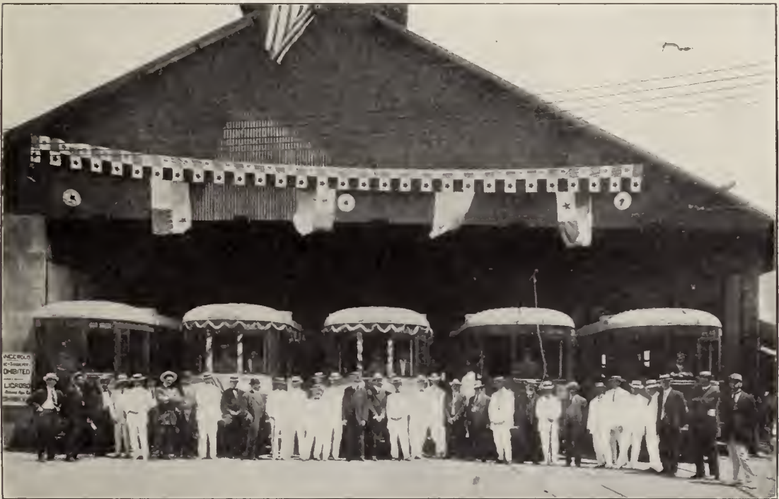
Celebration of the opening of the Panama tramways. Picture taken at the company's car barn.
