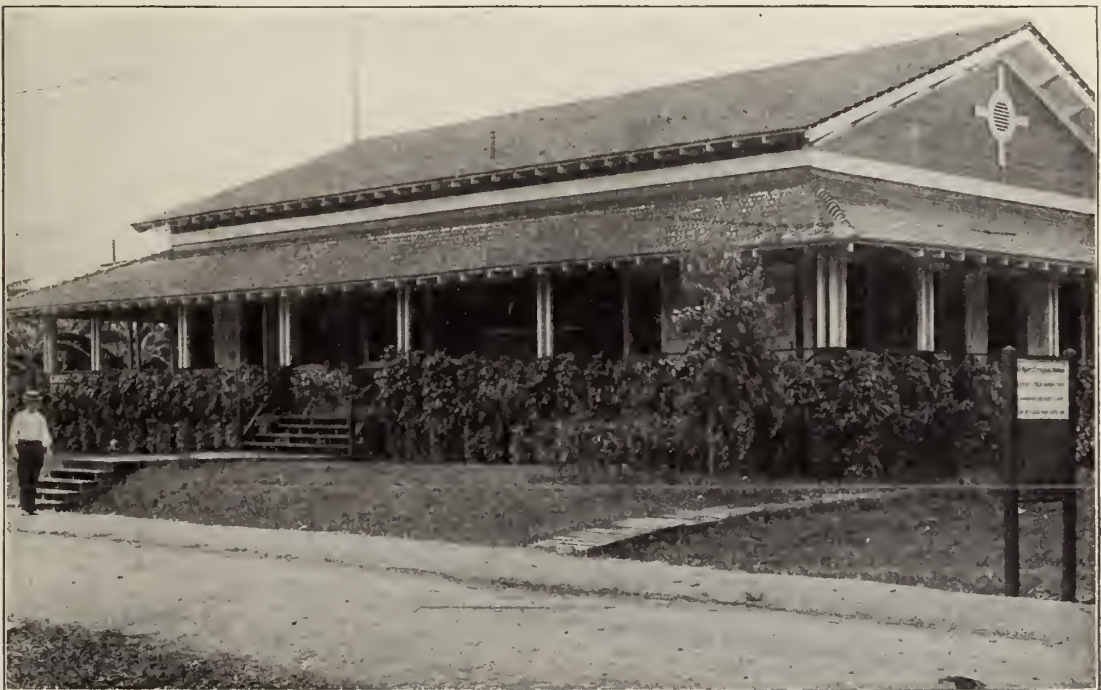
Present Court House at Empire. The United States possesses all authority over the Canal Zone, policing the territory and holding complete judicial power.
