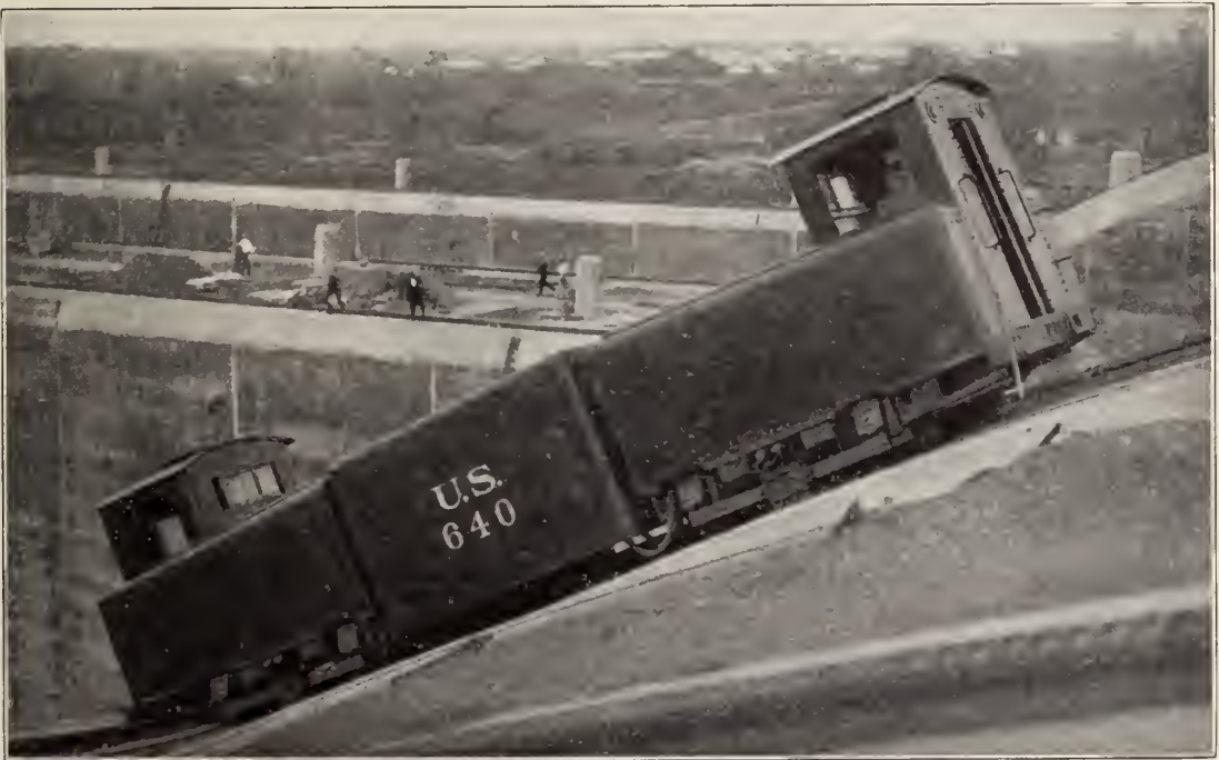
Towing locomotive in operation at Gatun Locks. These machines are designed to tow vessels through the locks. There will be two locomotives ahead towing, and two astern to retard the vessel's progress if required. In towing, they will not move faster than two miles an hour, but a second or return track, permits them to go back at greater speed.
