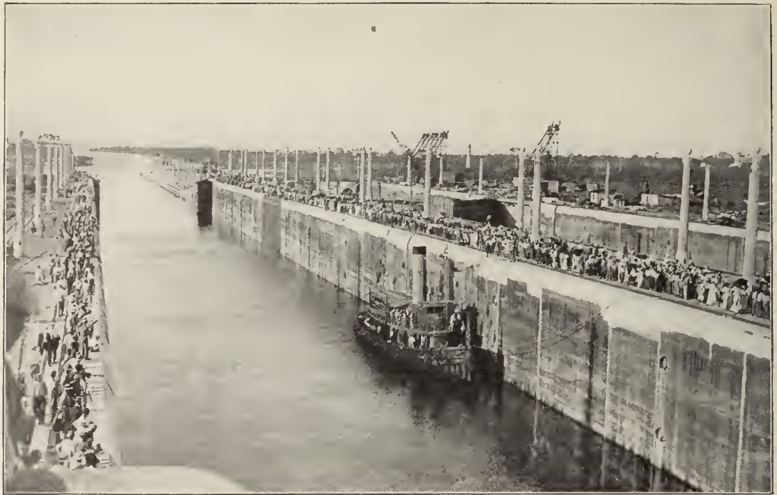
Tug comes to a stop alongside the center wall in the lower lock chamber.
