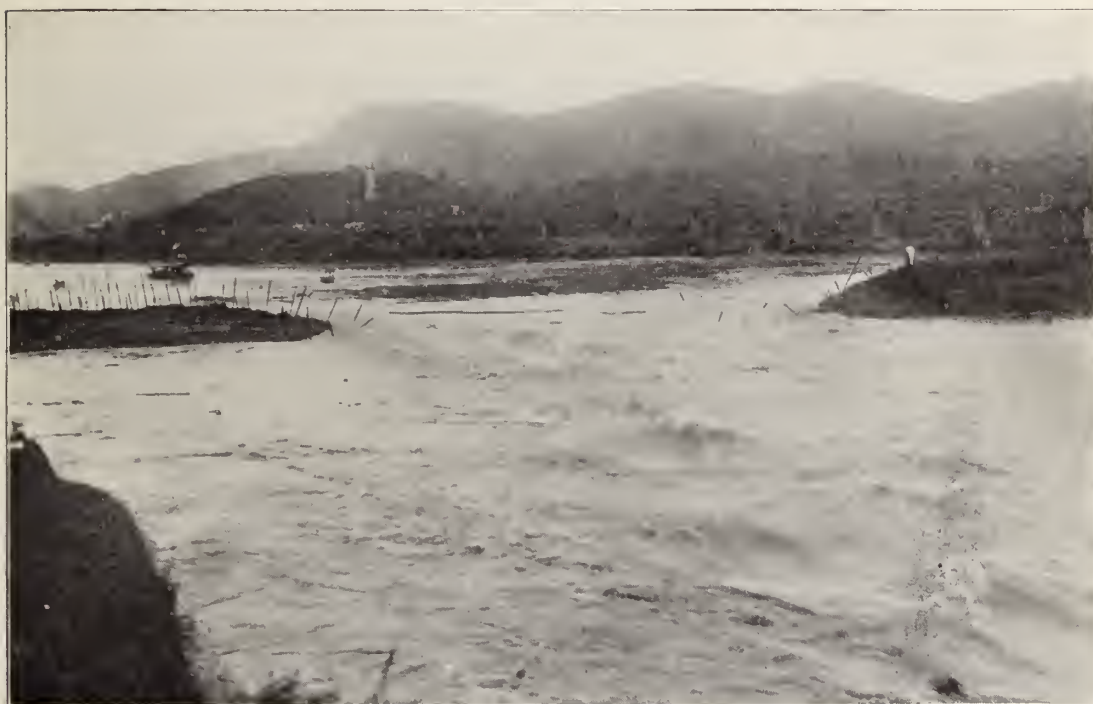
Water from Gatun Lake flowing into the Cut through the opening in the dike after the explosion. The first boat to pass into the Cut from the lake was a canoe containing two men.
