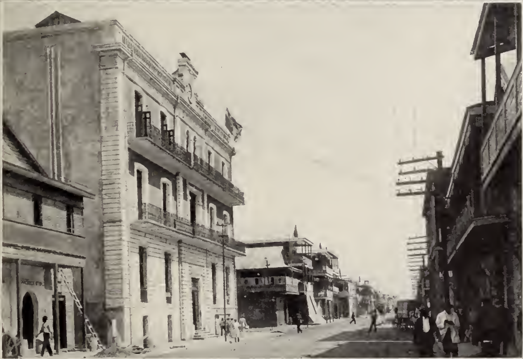
The above comparison of—before and after paving—is not exaggerated. When the Americans took charge of the work many of the streets in Colon and Panama City were veritable bogs in the rainy season. Now, both cities compare favorably in clean, well paved streets, with others of their size.
