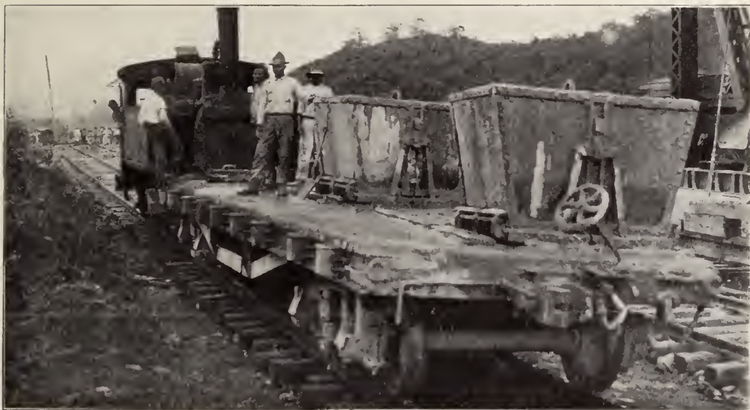
The finished product was carried by these trains into the lock chambers. Many of the old French locomotives were repaired and used for this work.
