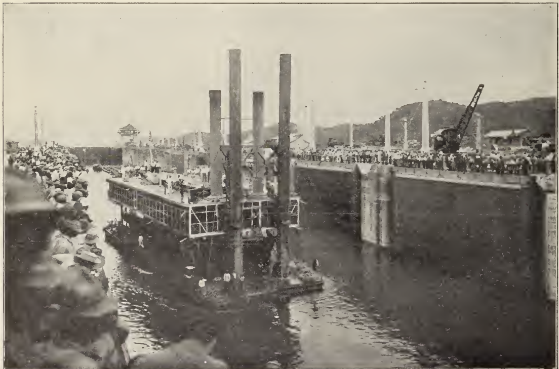
The Lock filled. Ready to pass out into the Culebra Cut channel.
