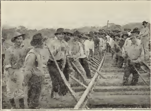
Men shifting track. The old way before the track shifting machine was invented, and put into use.
