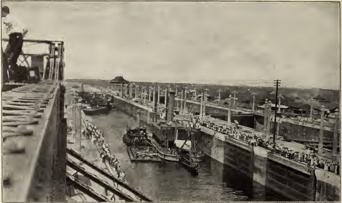
The vessels pass into the middle lock chamber.
