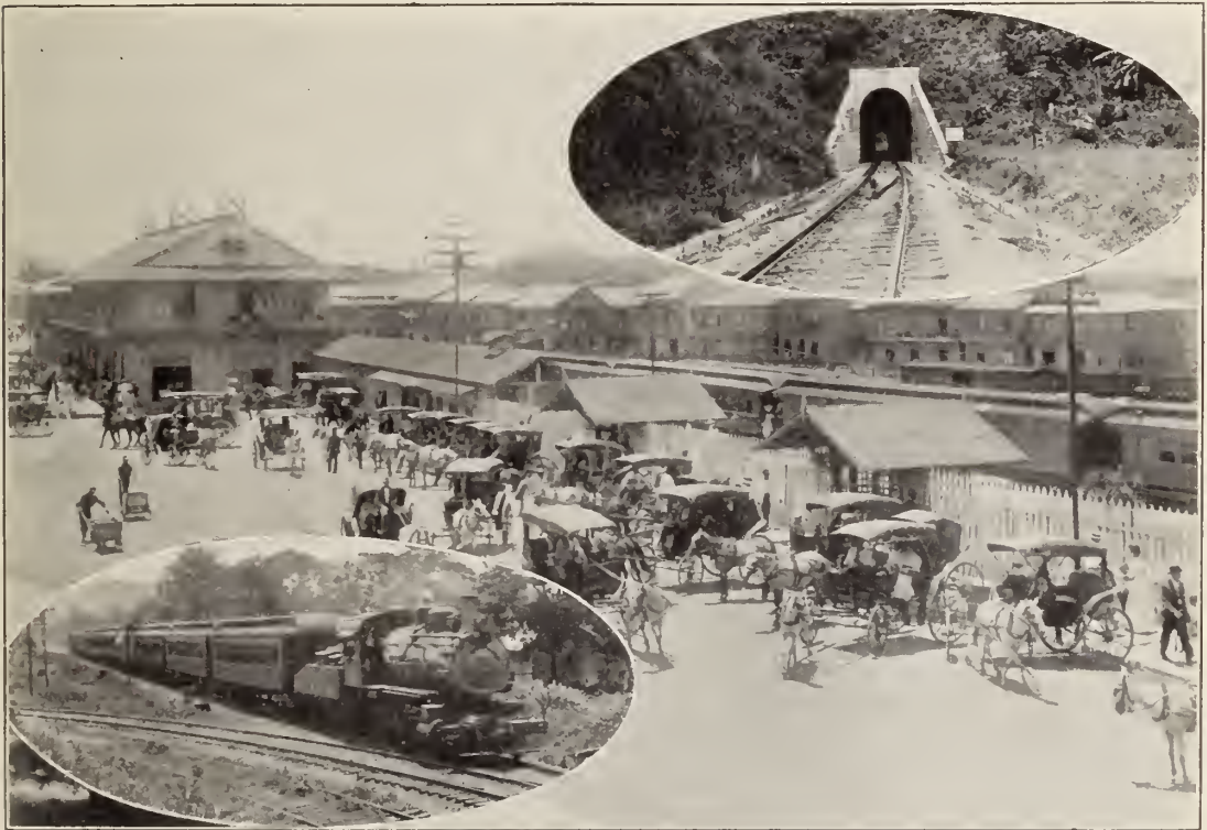
The station of the Panama Railroad at Panama City always presents an active scene at train time. A new first class station has taken the place of the old one shown here. All passenger locomotives are oil-burning and the coaches are thoroughly up-to-date, having first and second class accommodations. The tunnel at Miraflores is 736 feet long.
