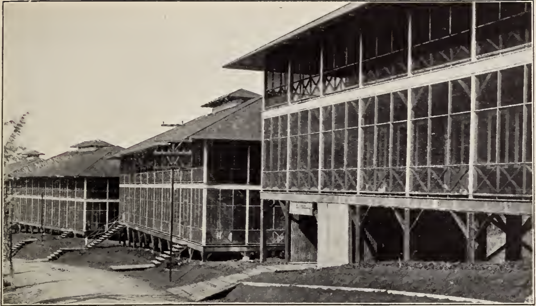
Each Zone settlement has buildings for bachelors commensurate with the force quartered there, furnished free by the Government. This type of quarters contains 24 rooms, with two men assigned to each.
