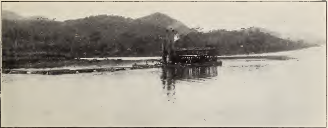
Suction dredge No. 82, removing silt from the channel north of Gamboa dike. This was the first dredge put to work in the Gatun Lake section.
