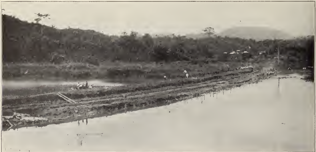
Gamboa Dike before it was dynamited.
