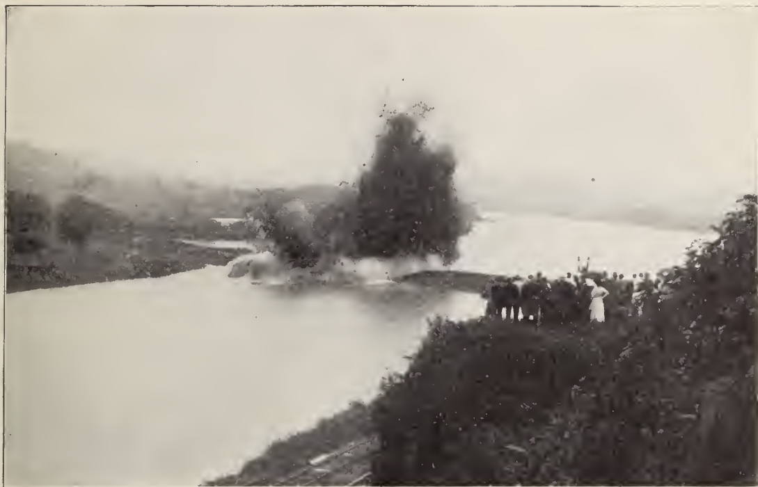
Blast that destroyed Gamboa Dike on October 10, 1913. The Cut had been filled to within a few feet of the level of the lake before the Dike was blown up.
