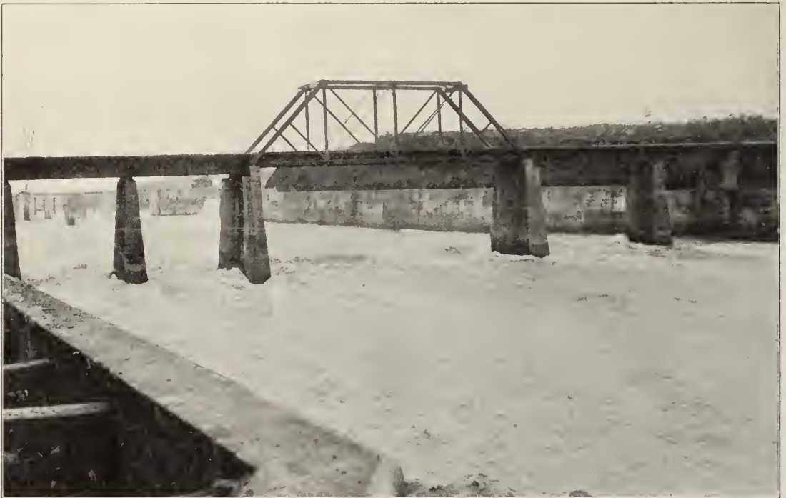
The overflow from the spillway passing out through the old bed of the Chagres River into the Atlantic Ocean. With the lake at its maximum elevation of 87 feet, the regulating gates in the spillway will permit of the discharge of a greater volume of water than the known maximum discharge of the Chagres River during a flood.
