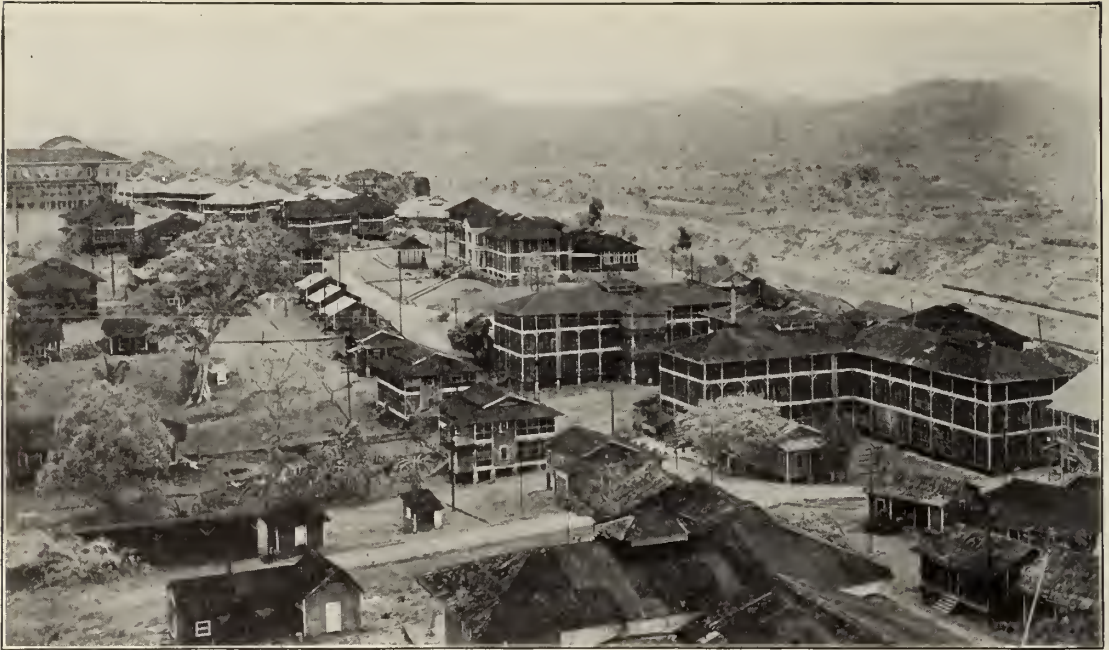
A view of the town of Culebra from Mount Zion as it appeared several years ago. The buildings to the right along the edge of the Canal, have all been removed on account of the slides at this point.
