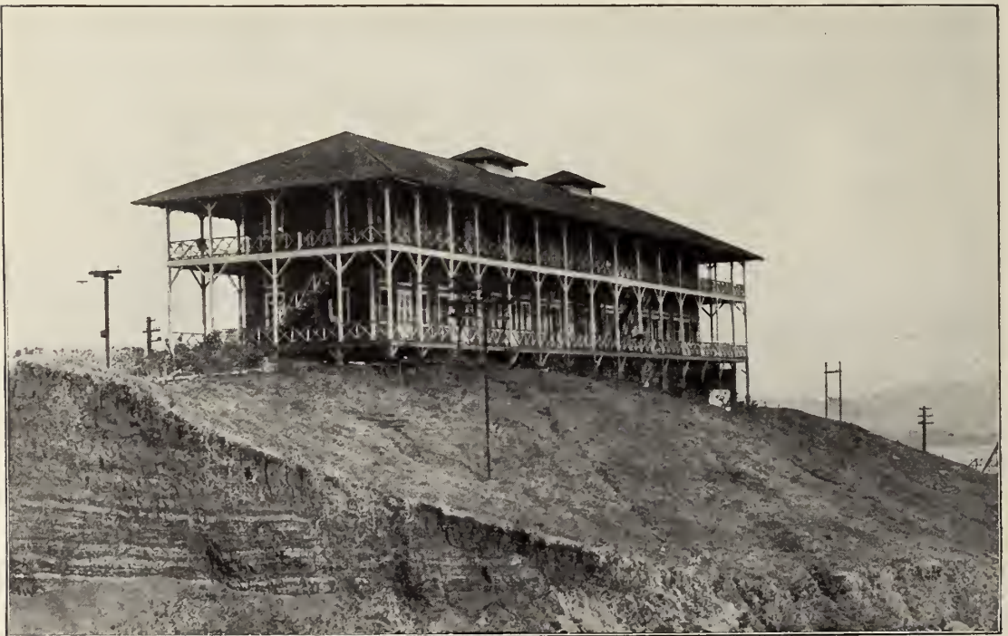
The Division Engineer's office at Gatun. Gatun is the engineering headquarters for the Atlantic Division, which embraces the construction from deep water in the Caribbean Sea to include the Gatun Locks and Dam.
