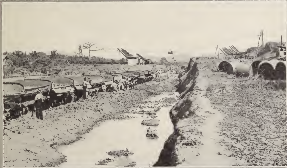
The top picture shows Bas Obispo in the first French Company's days, at the northern end of their proposed lock. The center picture shows French cranes at work. The French using laborers to fill cars is shown in the lower picture. Cableways, in the distance, were also used for handling spoil.
