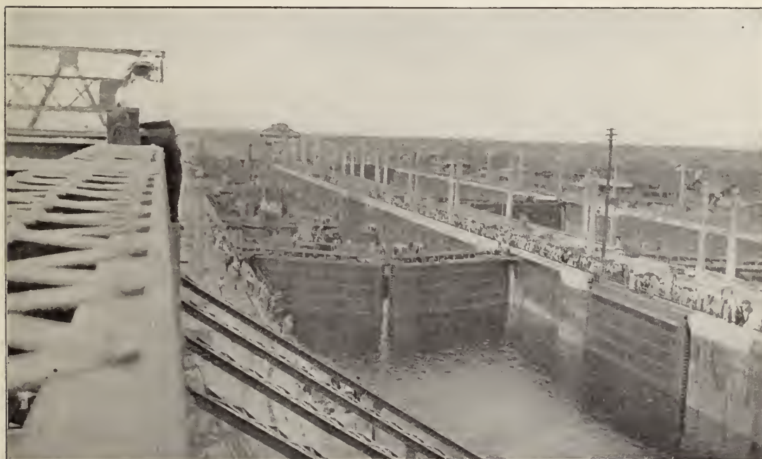
Opening the middle gate. The fleet, 13 vessels in all, nearly fill the lower lock chamber.
