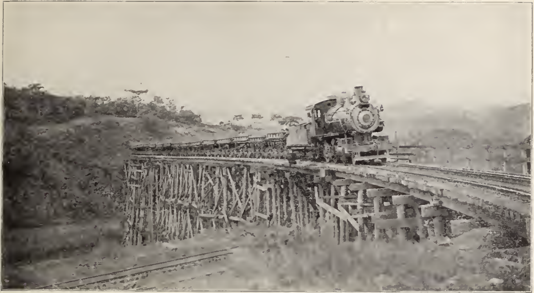
Loaded work train crossing the high trestle over the Canal at Paraiso. This bridge, known as No. 57½, is to be taken down as soon as the pontoon bridge a little above this point is constructed, as it obstructs navigation of the Canal.
