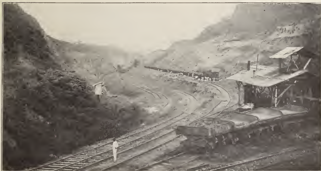
Culebra Cut at Gold Hill in 1887, during the French canal times. The space between the shed in the foreground and the first French locomotive is the zone of activity of the Cucaracha slide.
