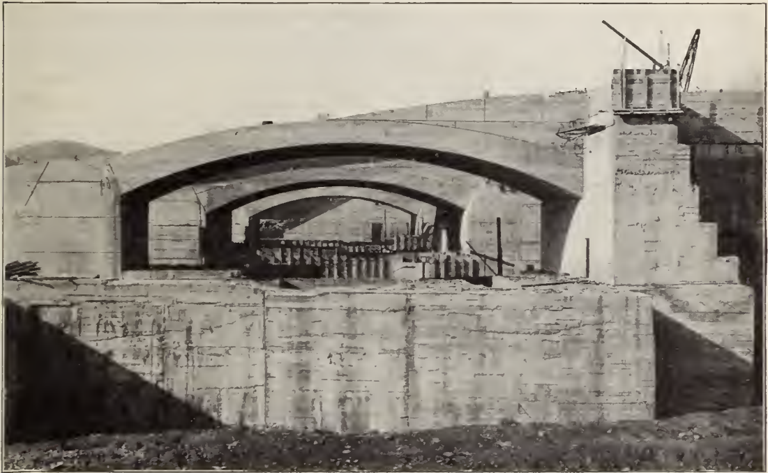
The lock walls as a whole give the visitor an idea of massive construction only. The arched sections, shown in the picture, connecting the main walls with the wing and guide walls, effect a saving in concrete and also give a symmetrical touch to the structures.
