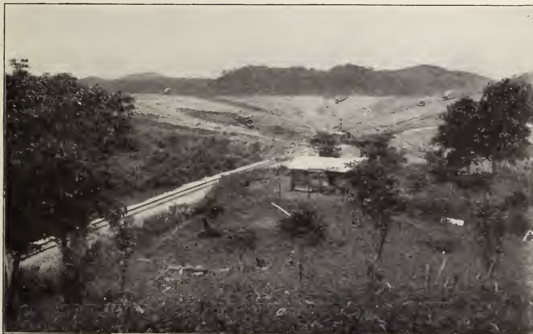
In order to dispose of the material from the Cut, large dumps had to be established. The site of this one, known as Miraflores dump, was formerly a swamp, but it has now been built up to a height of more than 40 feet. A large amount of the excavated material was used in building the Dam at Gatun and the Naos Island breakwater on the Pacific side. The spoil from Culebra Cut has been carried all the way from five to twenty-four miles.
