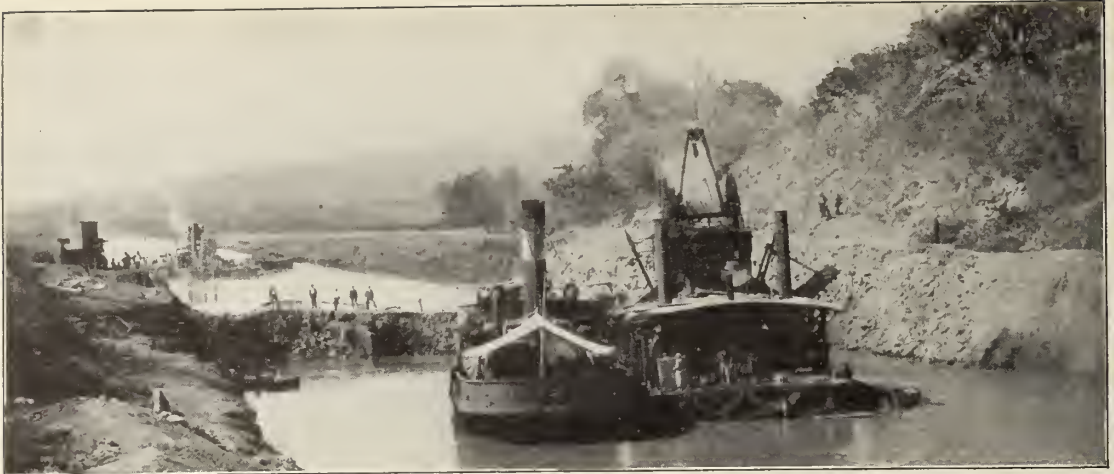
First French Company's days. Dredges working in the canal at Mindi.
