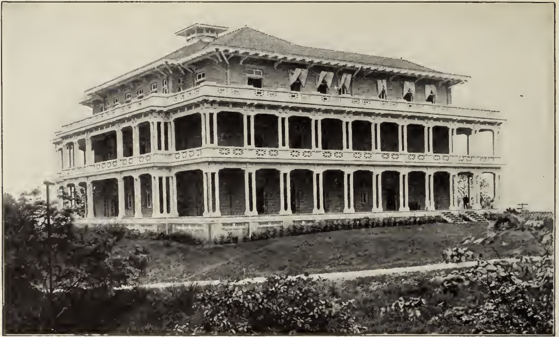
The Administration Building at Ancon, containing various offices, including those of the Secretary of the Commission, and the heads of the Departments of Civil Administration, Sanitation and Law.
