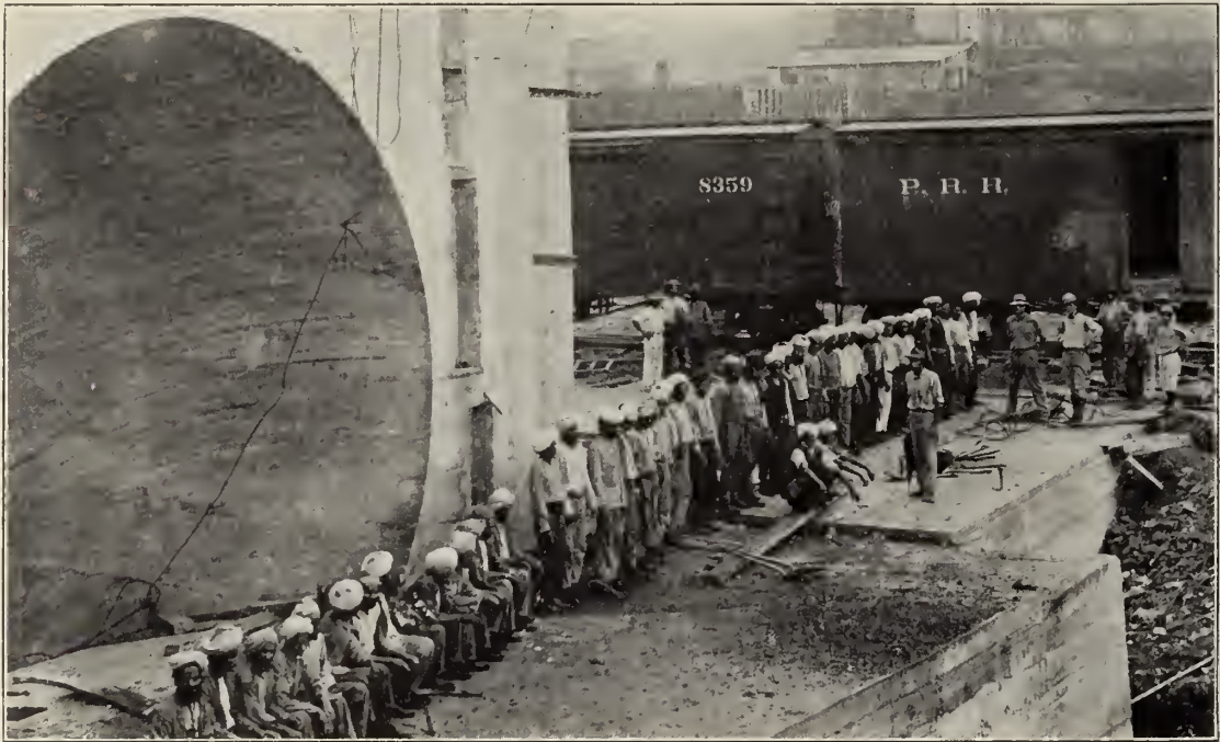
A group of East Indian laborers in the Canal service. Those sitting, are directly in front of an elbow in one of the great lock wall culverts.
