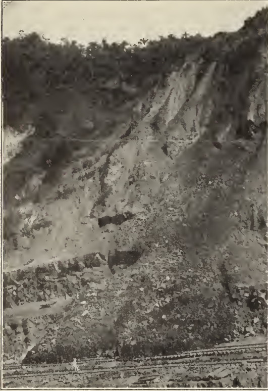
Close view of a slide in Culebra Cut.
