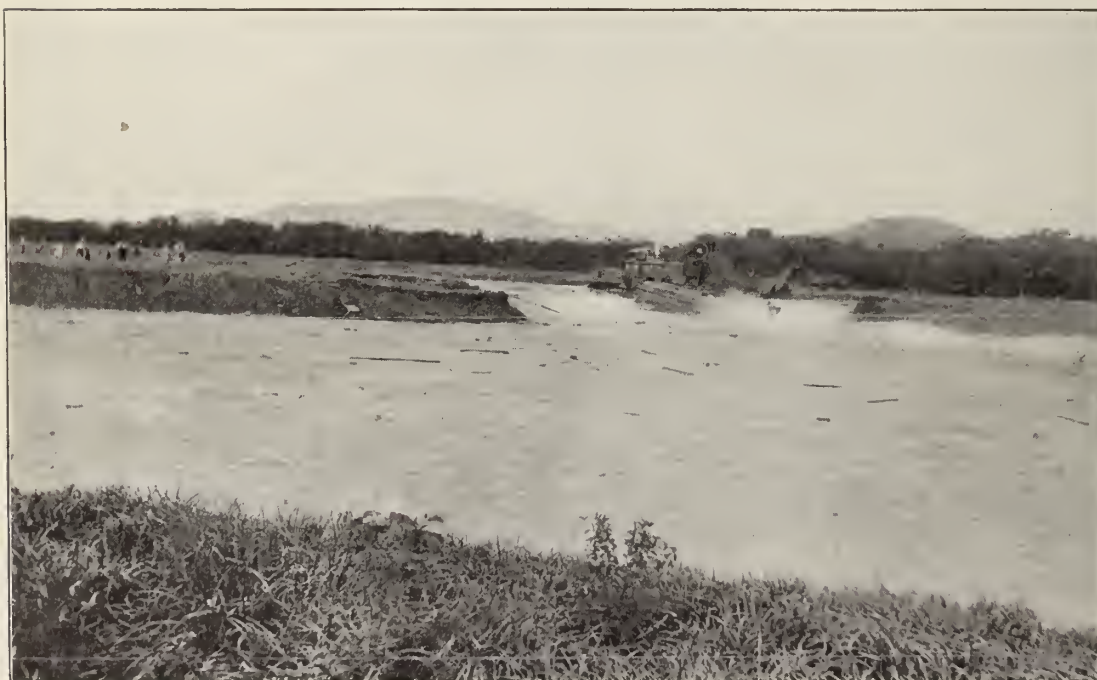
When the pit was nearly full, the suction caused a barge to break loose and to pass through the opening, snapping the steel cable in its progress like a piece of thread.
