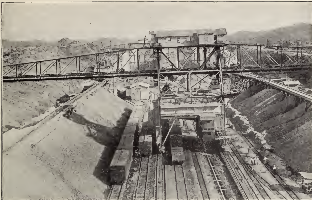
The handling equipment used at Pedro Miguel and Miraflores locks was entirely different from that at Gatun. At Pedro Miguel, Berm cranes, containing the mixing machinery, were stationed at the head of the lock, with arms extending on either side, from which grab buckets were lowered to pick up sand and rock, as the case might be.
