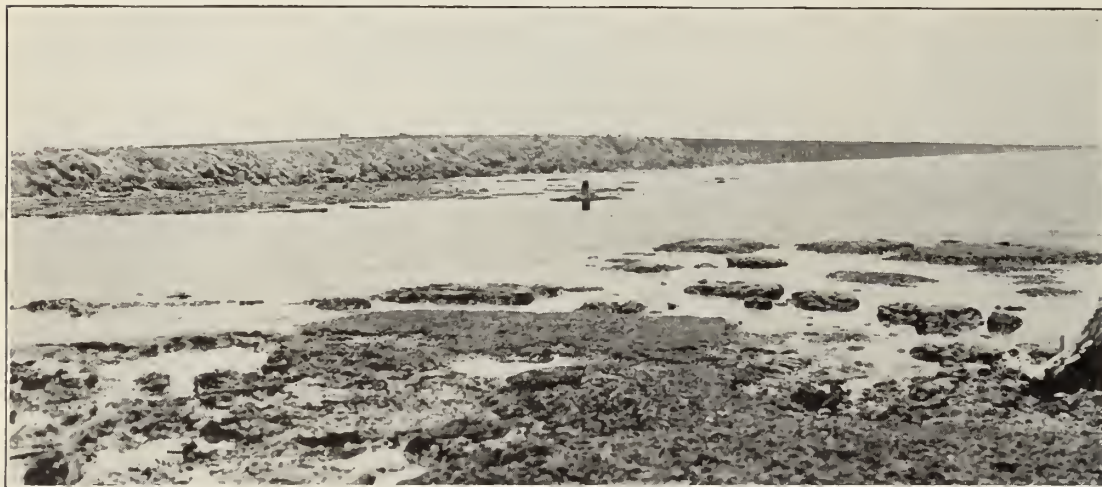
Toro Point breakwater. In order to protect the Cristobal docks and the Atlantic entrance to the Canal from heavy seas, a breakwater has been built out from Toro Point, on the opposite side of Limon Bay. It is over two miles long, and is armored with large rock brought from Porto Bello.
