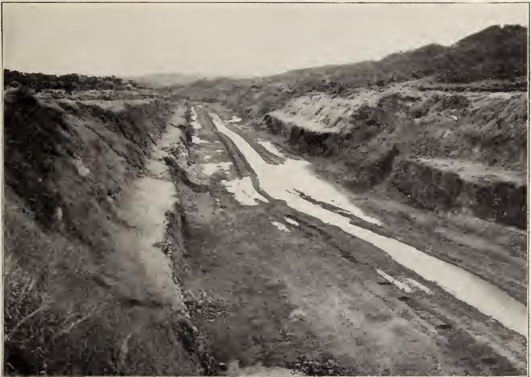
Section of Culebra Cut in the vicinity of Las Cascadas after completion. Various small slides have occurred all along the banks in this part of the Canal.
