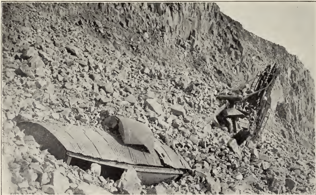
This graphically portrays the result of a slide which has nearly buried a steam shovel. Colonel Gaillard, the Division Engineer, in charge of operations in Culebra Cut said: "I know of no single thing that has done so much to complicate the engineering problems of our work or to hinder and curtail the yardage output as the slides." Colonel George W. Goethals, Chairman and Chief Engineer, said: "The only way to overcome the slides is by unremitting excavation."
