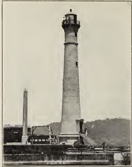
Close view of lighthouse on Gatun Locks. The Locks will be brilliantly lighted at night.
