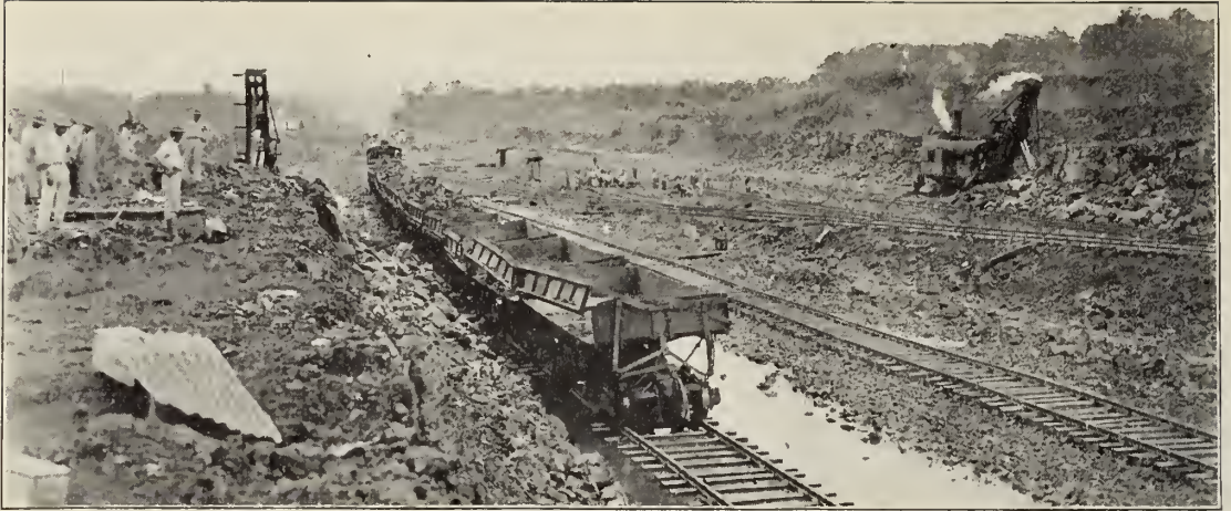
Excavating for lock site, Gatun.
