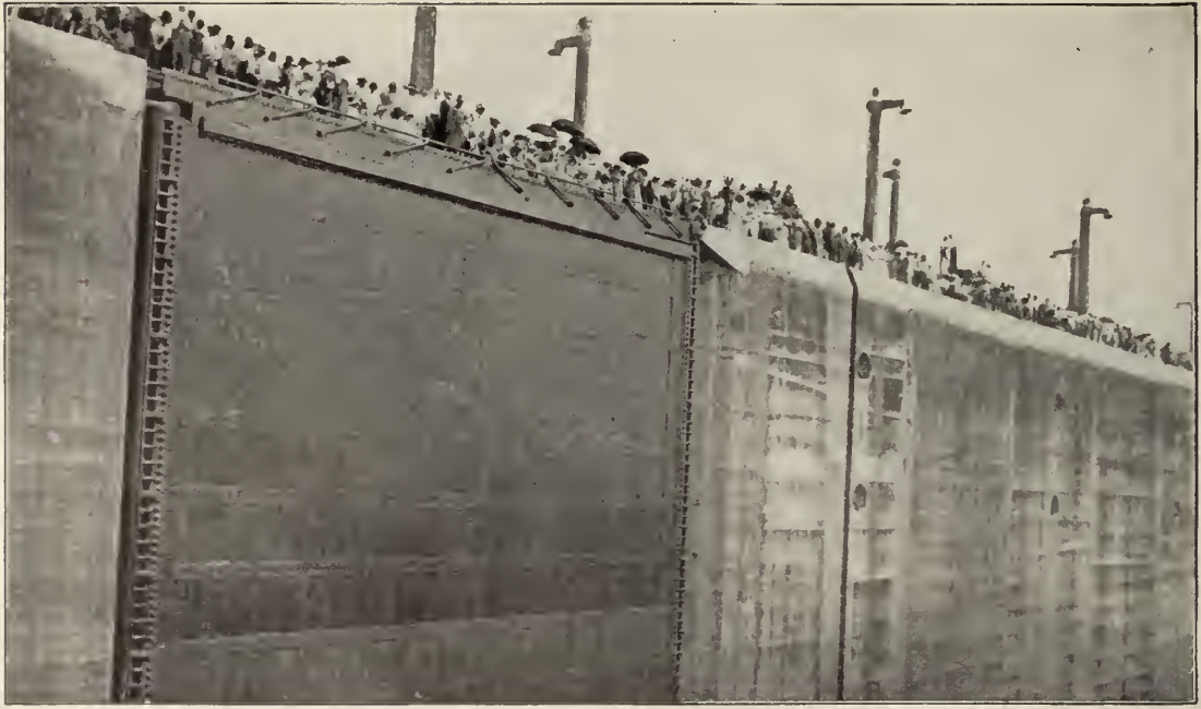
Gates in open position have appearance of being part of lock wall.
