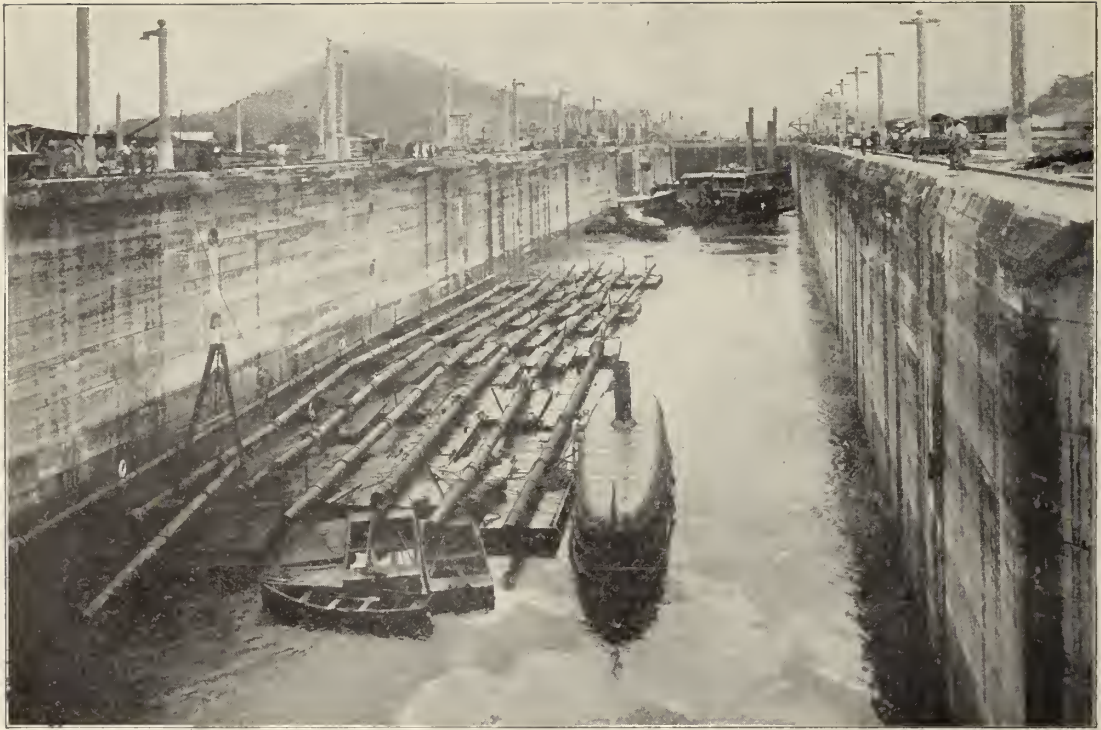
Waiting for the Lock to fill. The pipe on the barges was part of the outfit of dredge No. 85, for use at Cucaracha slide.
