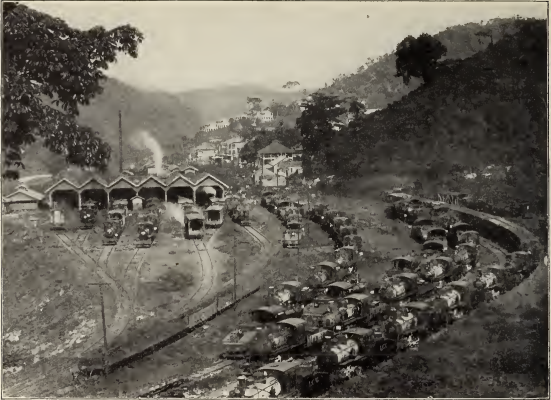
General view of engine house and yard at Paraiso in 1906. This yard was dismantled several years ago, and yards were established at Pedro Miguel and Las Cascadas.
