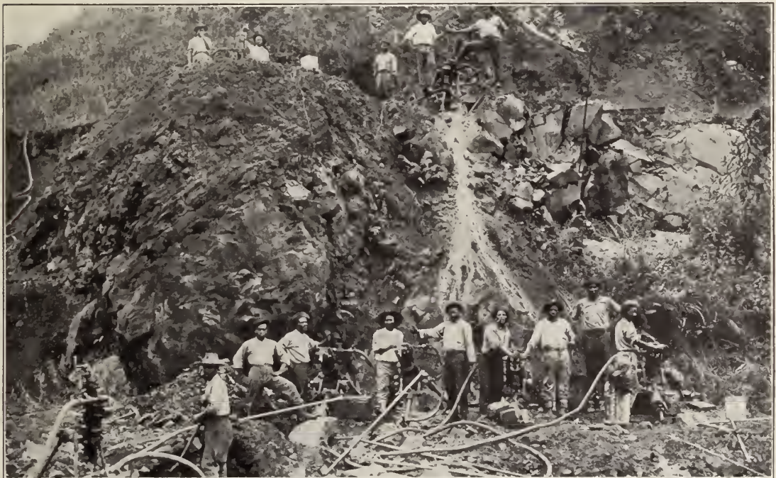
A group of tripod drills at work. Churn drills are used also. All drills are operated by compressed air supplied through mains, and an average of 75 miles of drill holes is sunk each month.
