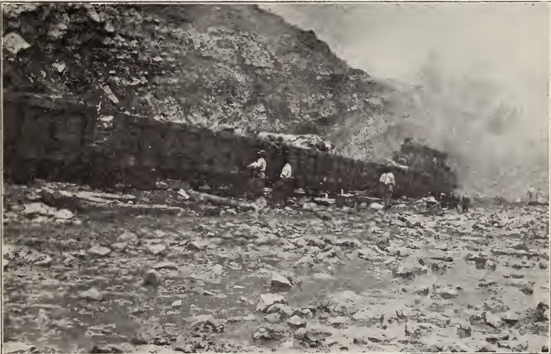
Last train of material out of bottom of the Cut.
