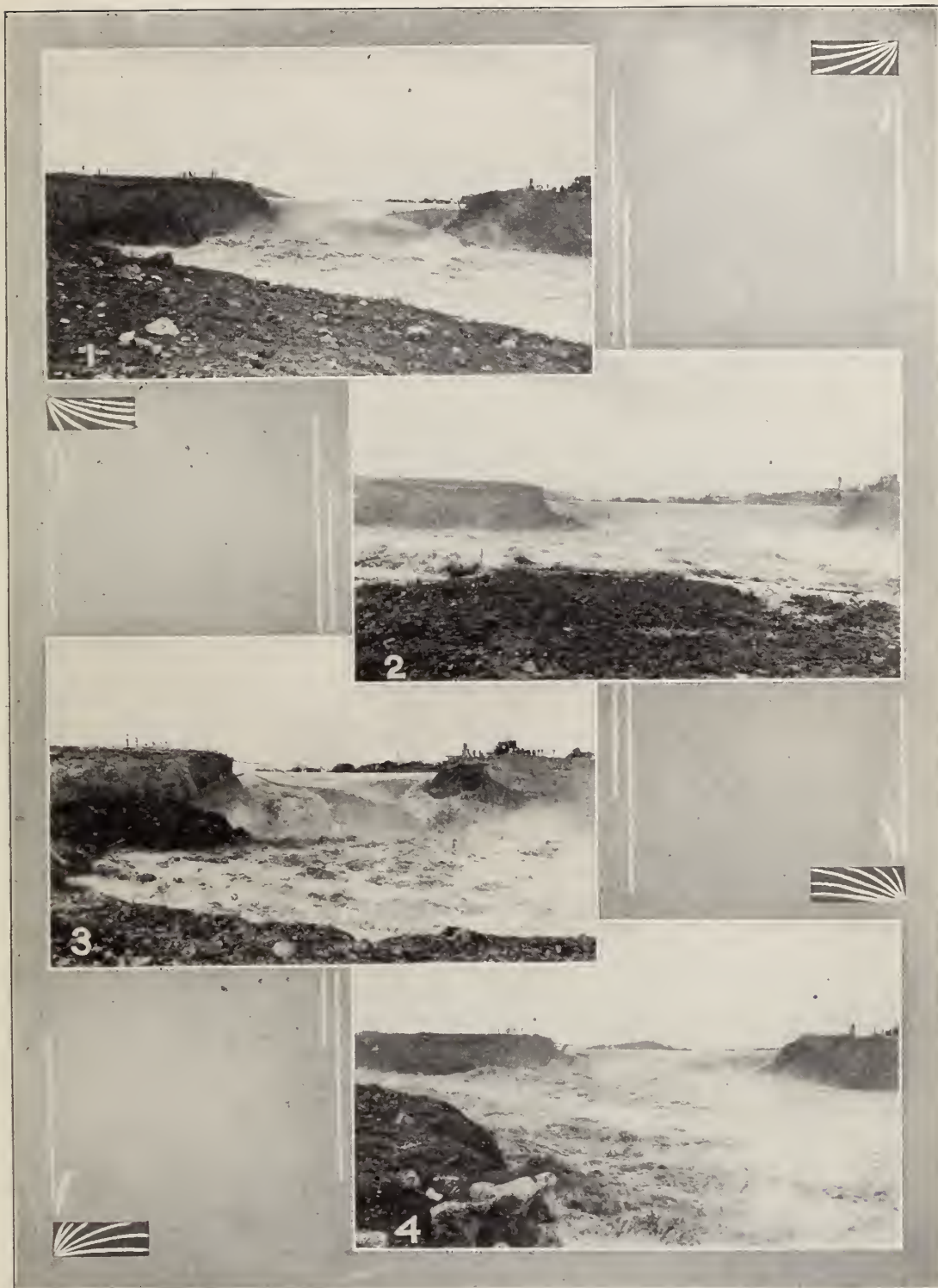
While the water was surging into the pit, the phenomenon of the tide being held stationary for three-quarters of an hour was observed at Balboa eight miles away. 1. The rush of water continues. 2. The opening about one hour after the water first went through. 3. A steel cable hung across the fall, which the rush of water thrashed back and forth. 4. The pit is gradually filling.
