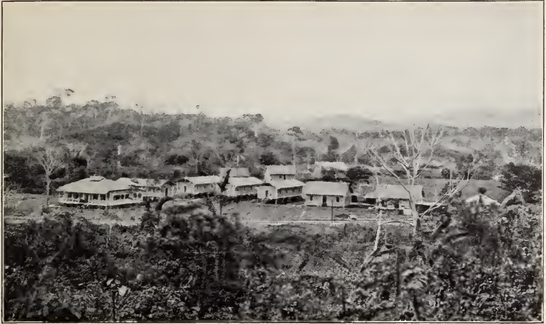
Typical camp for European laborers. There are separate camps for each class of employes, and the American section of a Canal Zone town is entirely by itself.
