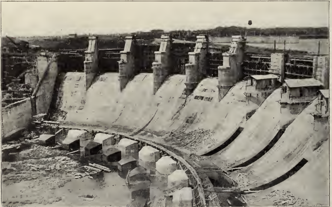
The spillway Gatun with the sluice gates closed. Locks and village of Gatun in the distance.
