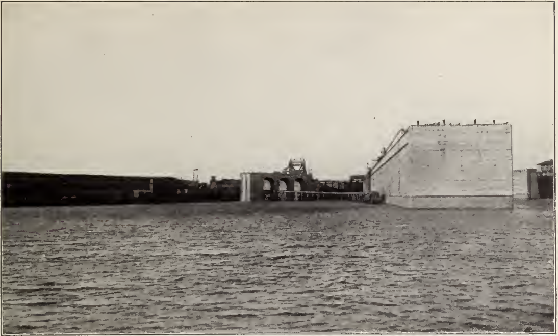
Entrance to Gatun Locks from the lake. Gatun Dam on the left and approach wall in the foreground. Approach walls 1,000 feet long, have been built at each end of all the locks, and as the name indicates, they serve as a guide to ships coming up the approach channel. Ships must come to a stop at these walls, until the locomotives which tow them through the locks make fast their lines.
