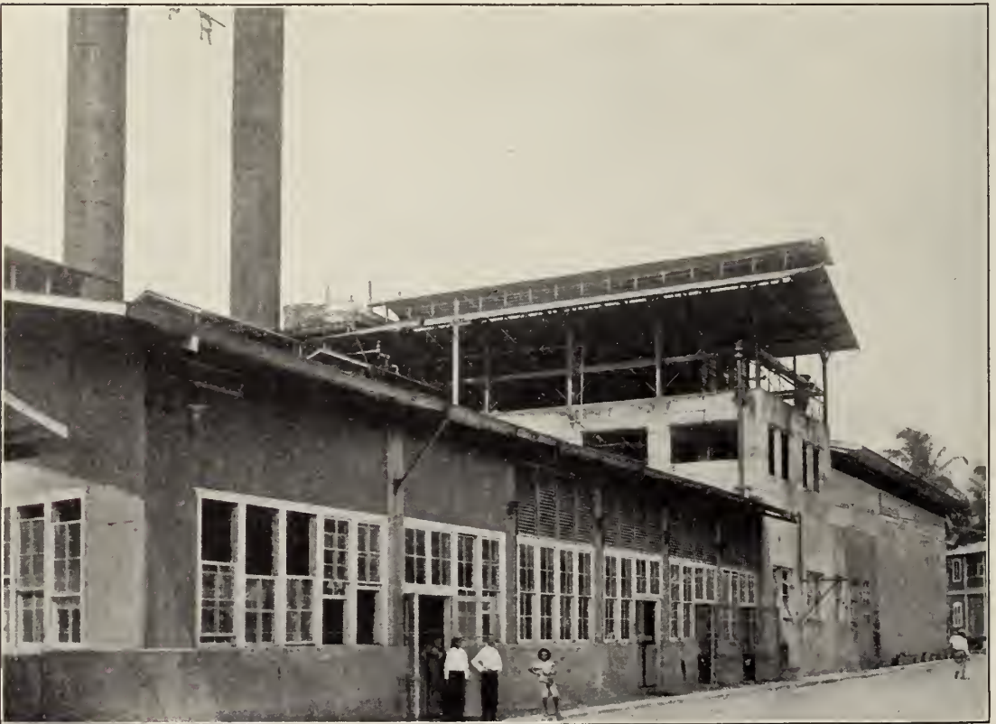
Ice and cold storage plant, Cristobal. Ice is sold at 40 cents per 100 pounds, and cold storage articles are cheaper, in many instances, than they are in this country from which they are imported. This is largely due to the system of buying in bulk and, in the case of meats, to the placing of contracts.
