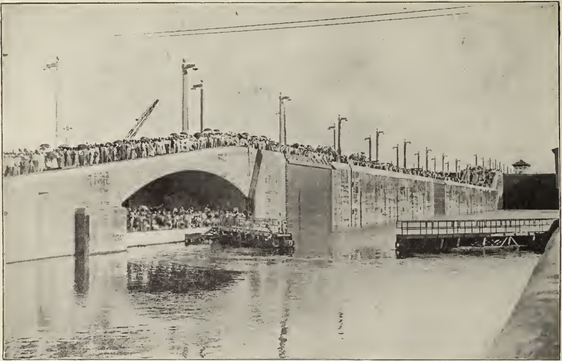
Water in the lower lock and sea level channel equalized. Opening the lower guard gate.
