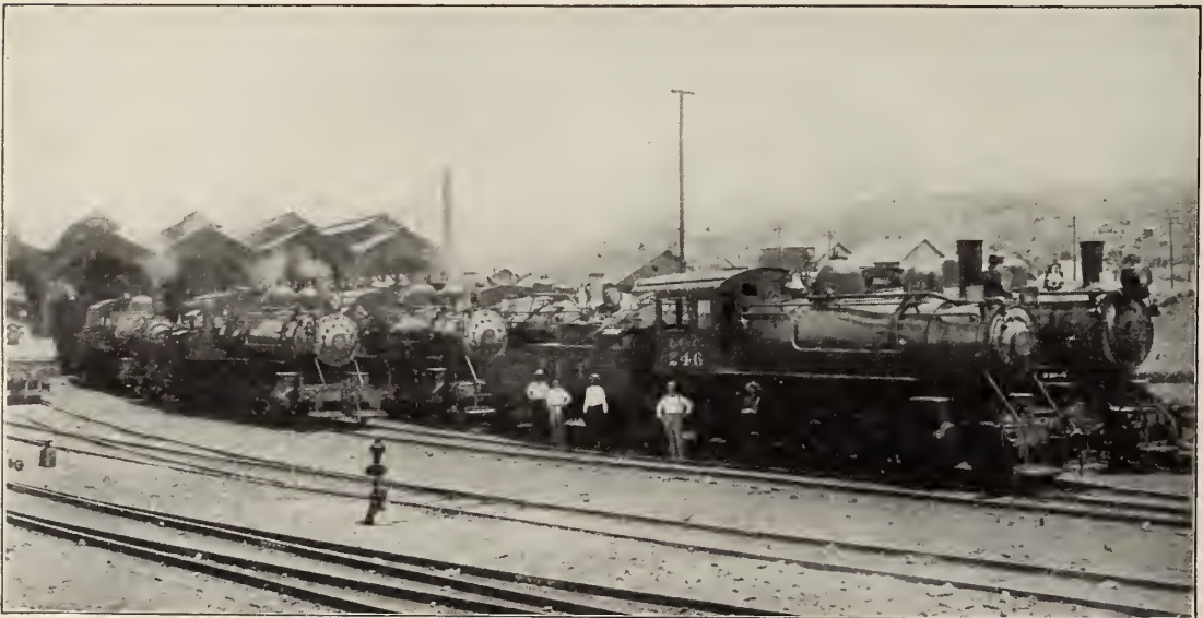
Engine house and yard at Las Cascadas. A very busy scene was presented in the morning when a hundred or more of the engines were leaving the yard to begin their daily work of pulling dirt trains out of the Cut to the dumping grounds.
