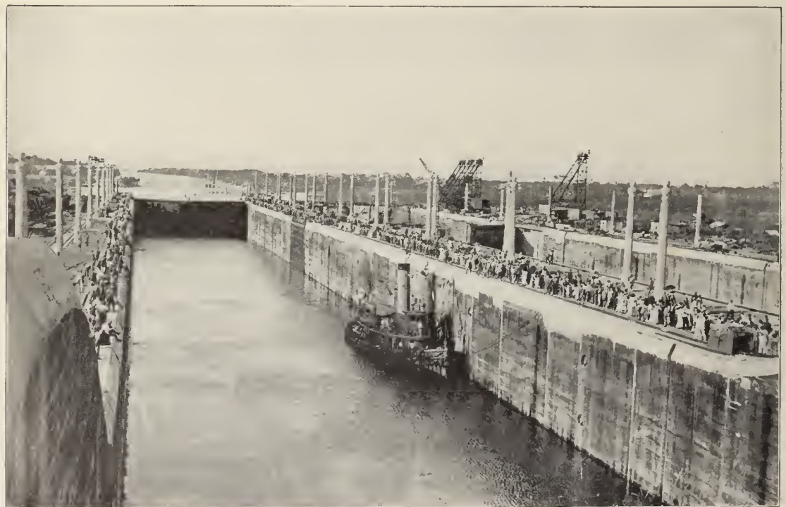
Gate is closed preparatory to filling the lock for the lift to the middle chamber.
