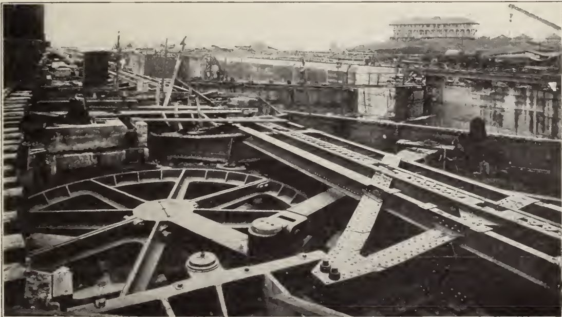
The operating mechanism of a lock gate. The wheel is a bull wheel, which, in operating, turns through an arc, giving the connecting rod the movement of an arm in opening and shutting a door. It is 19 feet in diameter, and weighs over 35,000 pounds.
