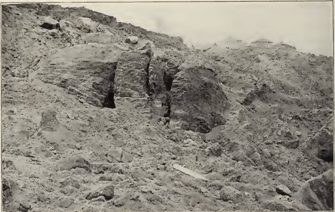
Telling effects of the slide in the west bank at Culebra. Most of this has now been cleared away, and the danger of similar trouble at this point has largely passed, because of the method adopted of terracing the upper levels to relieve the weight on the banks.
