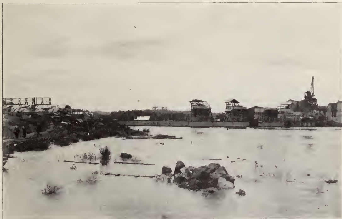
Gatun spillway, looking from the lake. The spillway is a concrete lined opening, 1,200 feet long, 285 feet wide and is situated about midway of Gatun Dam.
