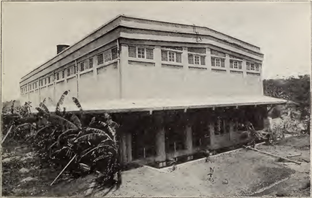
Power stations are situated at various points along the Canal to furnish power to the electrically-operated machinery, as well as to light the Canal Zone settlements. The building shown in the picture is the Miraflores station which supplied power to the construction machinery at Pedro Miguel and Miraflores Locks. It is an oil-burning plant but can be converted to a steam plant at any time. Many of the industrial plants and all passenger locomotives are equipped with oil burners.
