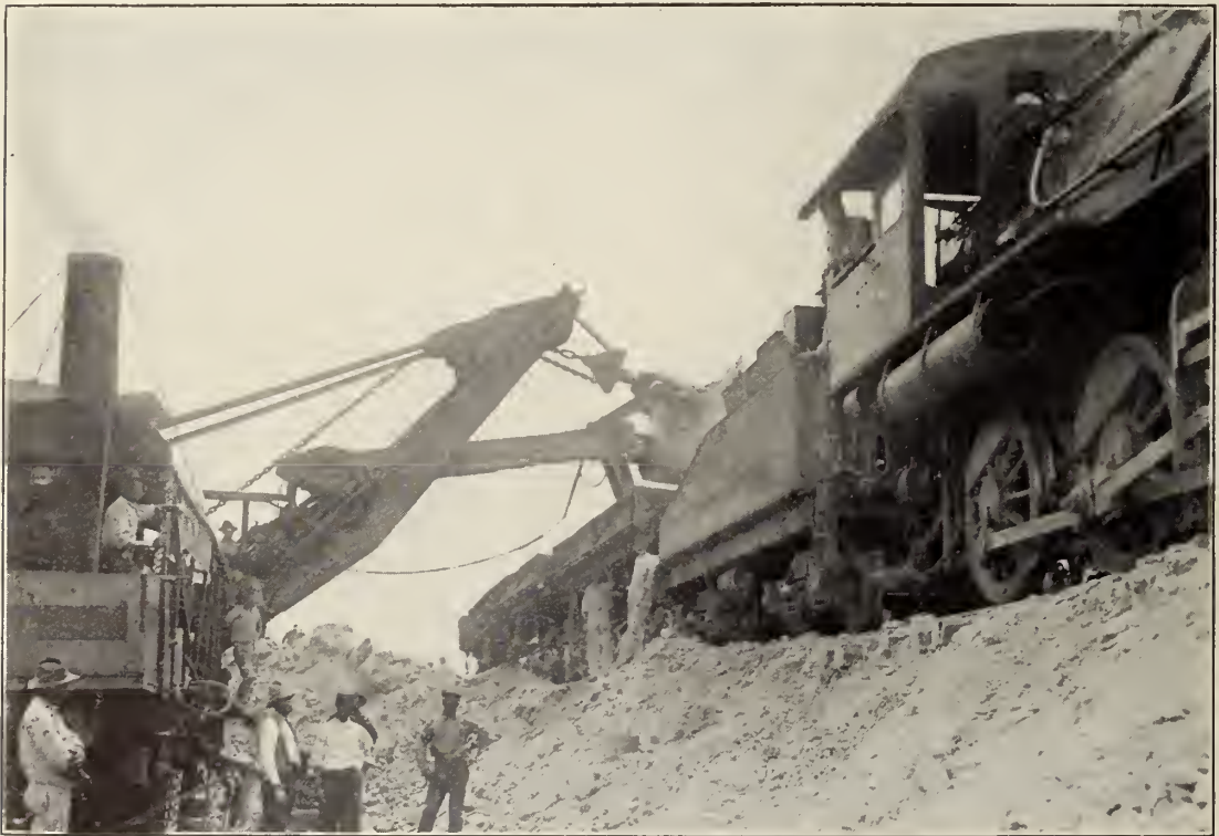
Loading dirt train for trestle fill.
