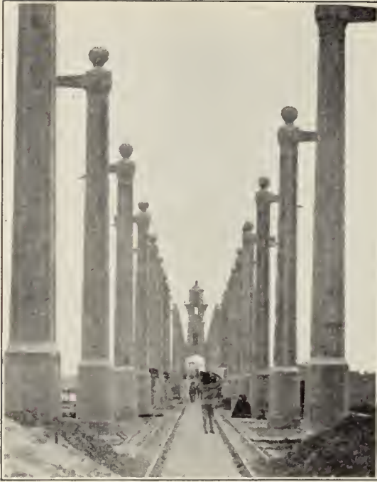
An avenue of lamp posts on Gatun Locks. Lighting tower in the distance.
