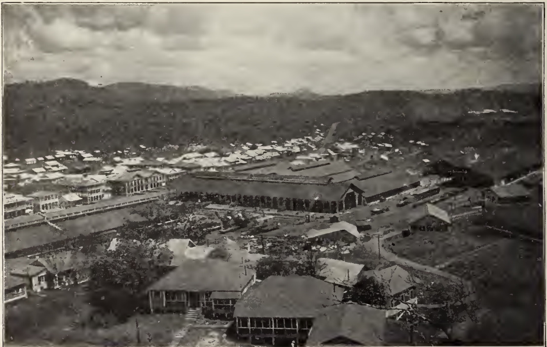
Repair shops at Empire, showing the native village in the background. All major repairs to steam shovels were made at these shops. Steam shovels were inspected daily and the minor repairs were done in the field.
