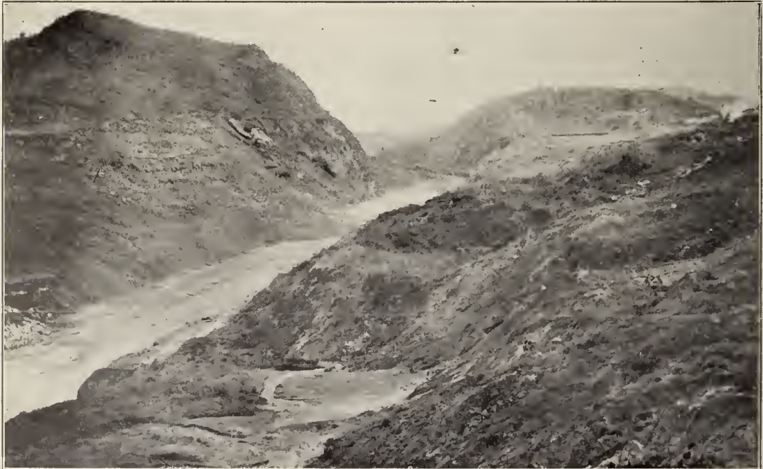
Culebra Cut opposite Culebra village after removal of steam shovels and construction tracks, Action of slides graphically pictured here.
