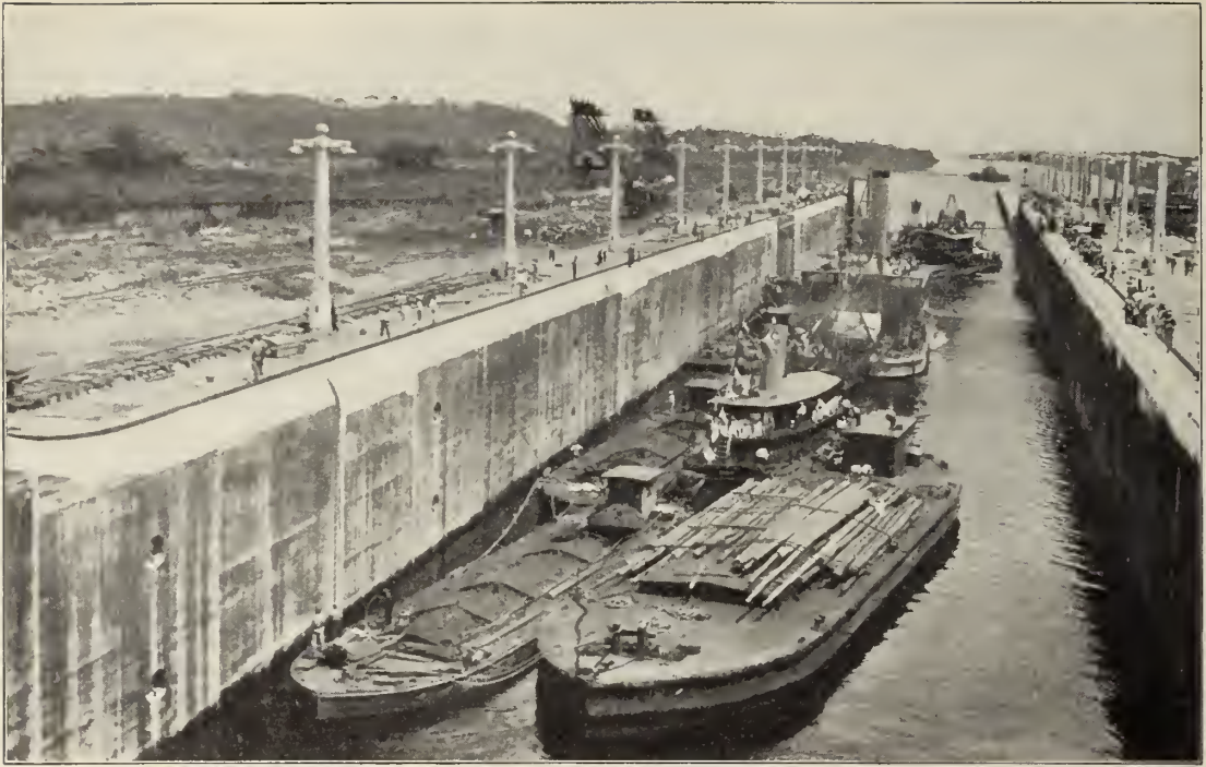
Tugs, dredges and barges entering the lower lock from the sea channel.
