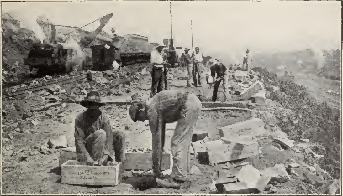
Laborers loading well-drill holes with dynamite near Contractor's Hill. A small charge is first exploded, enlarging the hole at the bottom. Then the main charge, usually consisting of from 75 to 200 pounds is placed, and exploded by means of an electric light wire.
