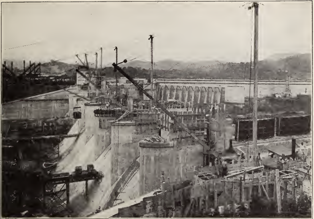
Miraflores spillway, completed September 1, 1913. Lies between Miraflores Locks and rising ground to the east, and forms Miraflores Lake. It also regulates the level of the lake.
