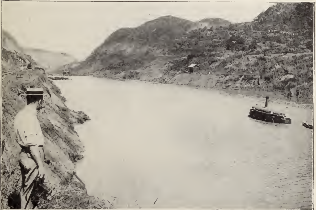
View of the Cut about 800 yards south of Cucaracha slide. Dredges No. 85 and 86 may be seen in the distance working on the south and north sides of the slide, the last barrier to a passage through the entire Canal.
