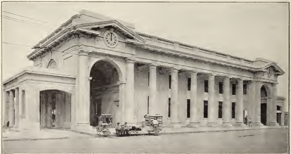
New Panama railroad passenger terminal in Panama, just completed.
