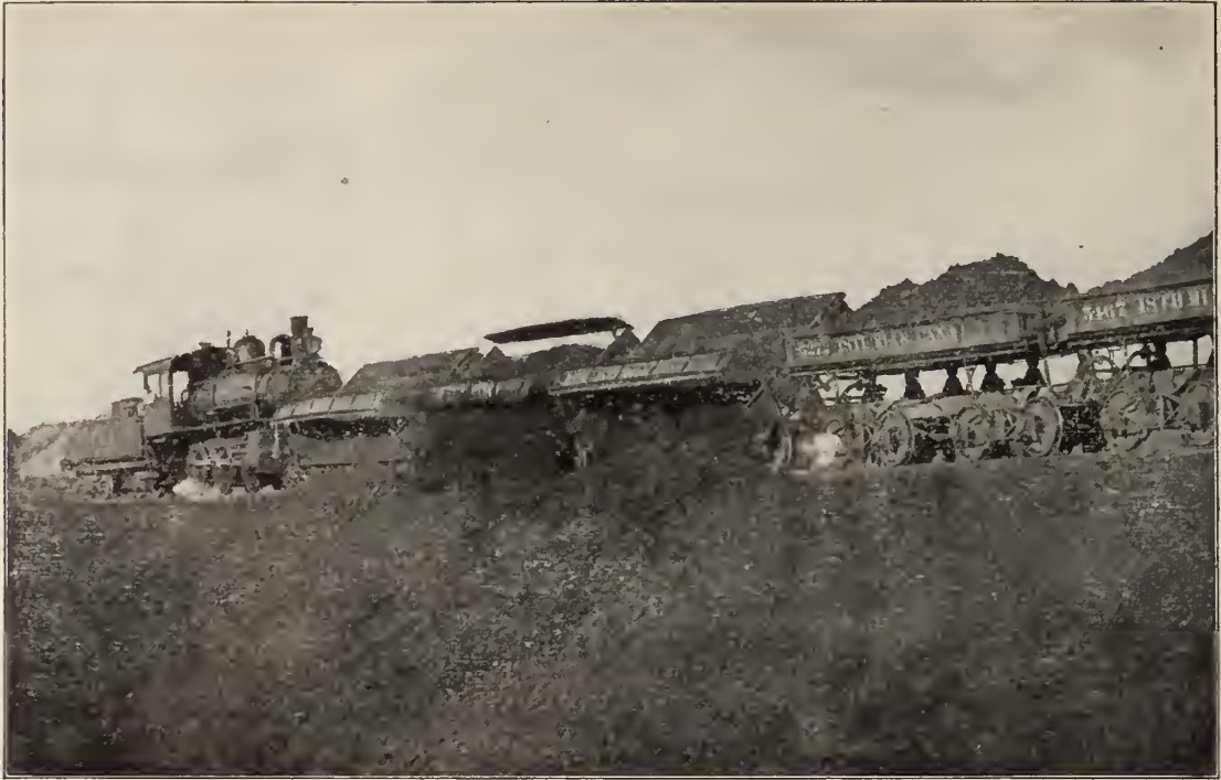
Excavated material is transported in several kinds of cars, one of which is the Western Dump Car, shown in the picture. In some of the cars, the body is held upright by a chain grip, which, when released, allows the body to tip, emptying the contents. Others are dumped by air.
