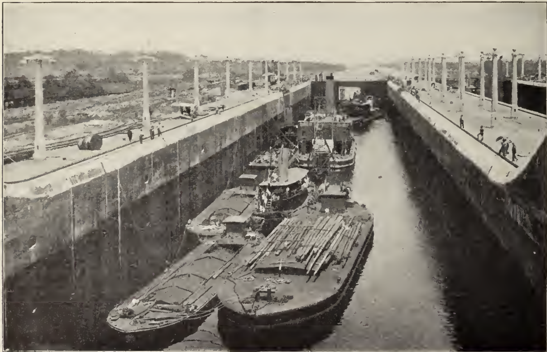
Closing the lower lock operating gate.
