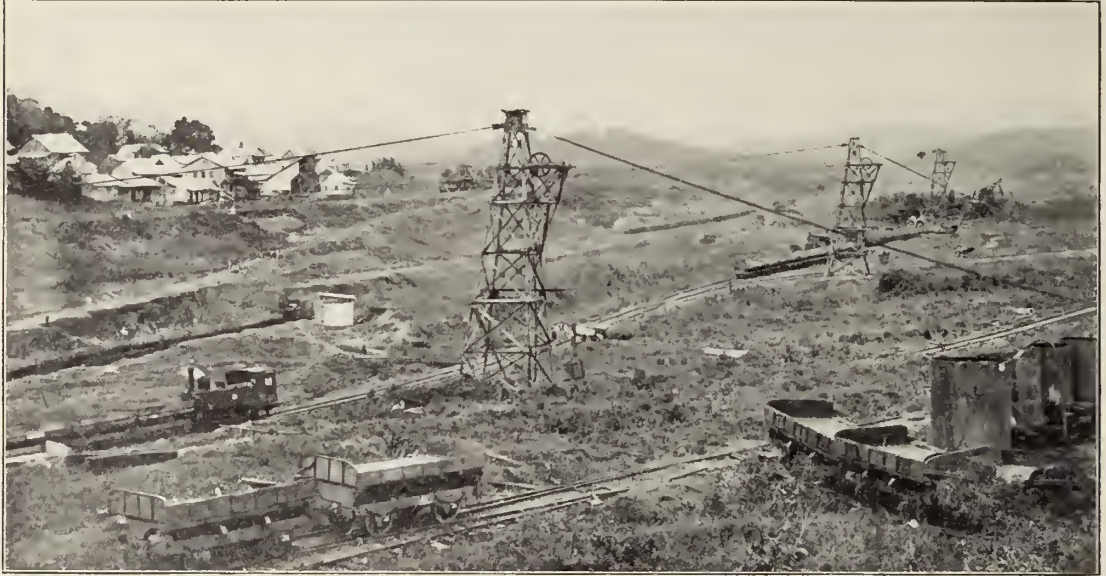
The Cut in French times, showing their cableway plan of excavation. These cableways carried the material out of the canal and deposited it to one side, but unfortunately not far enough, for much of it has slid back into the Cut, causing extra excavation.
