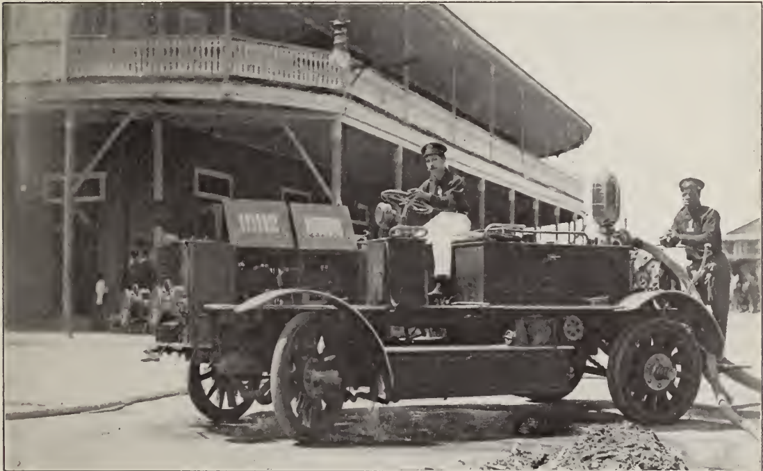
Automobile fire engine of the Panamanian fire department at Colon. The city of Panama is also provided with one of these modern machines.
