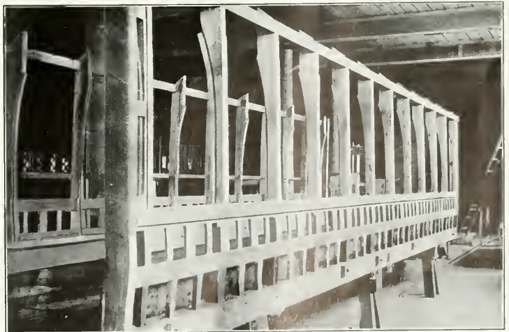
STREET CAR CONSTRUCTION
