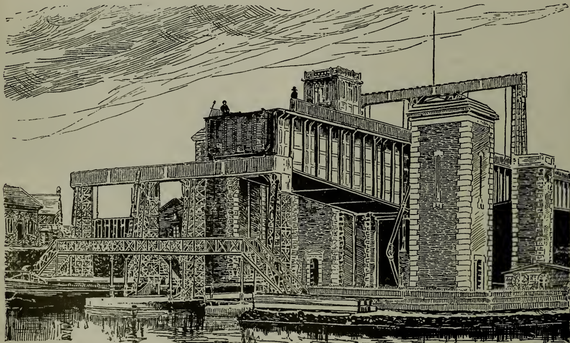
FIG. 4.—HYDRAULIC CANAL LIFT AT LES FONTINETTES, FRANCE.
