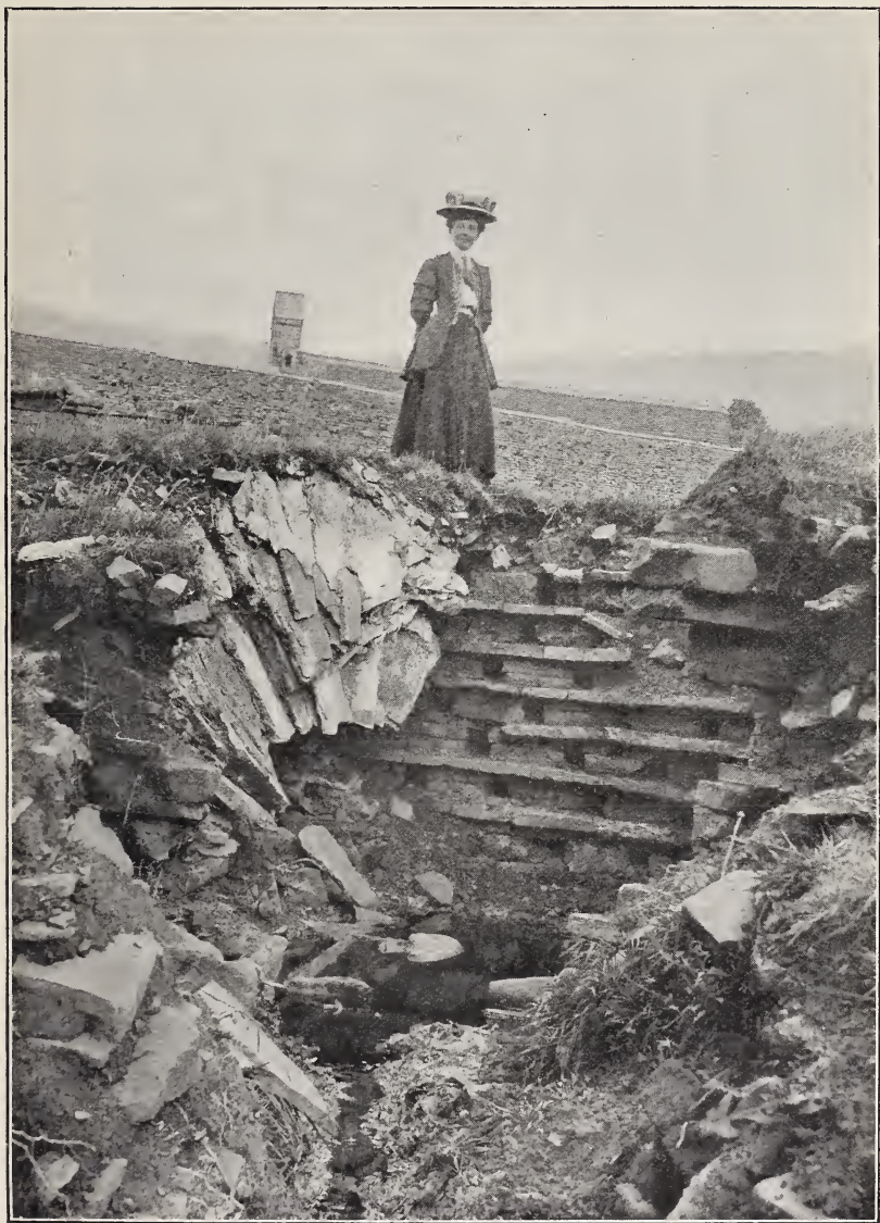
Columbarium, Llanthony, as seen through the breach made by the workmen, showing Roof
