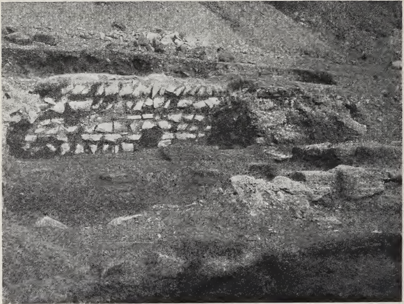
Glasfryn, Tremadoc : View showing position of hypocaust pillars in Room F
