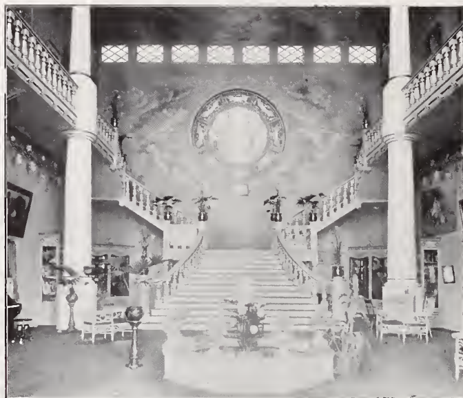
STAIRWAY IN WOMEN'S BUILDING.
