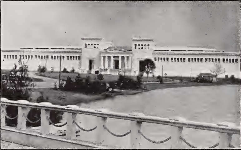
MACHINERY BUILDING, FROM LAKE WATAUGA.
