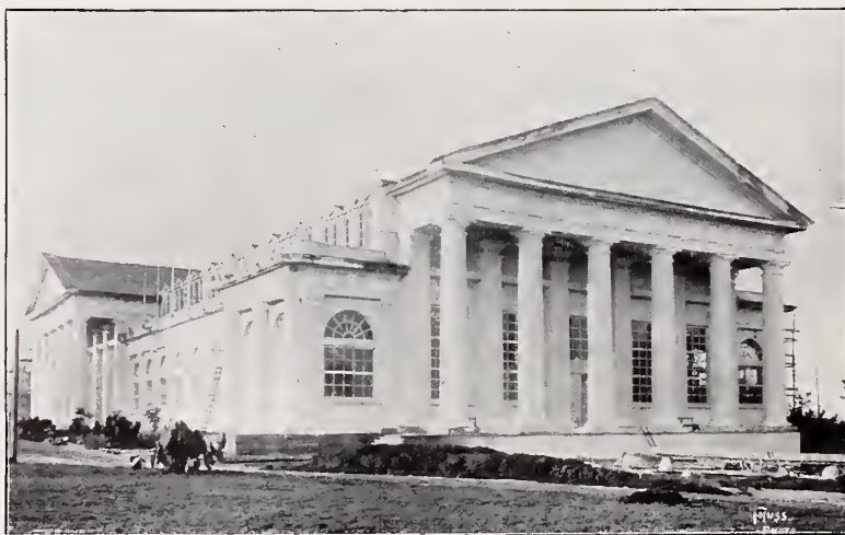
MINERALS AND FORESTRY BUILDING.
