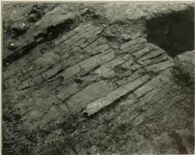
b. Close-up of slabs in place.
