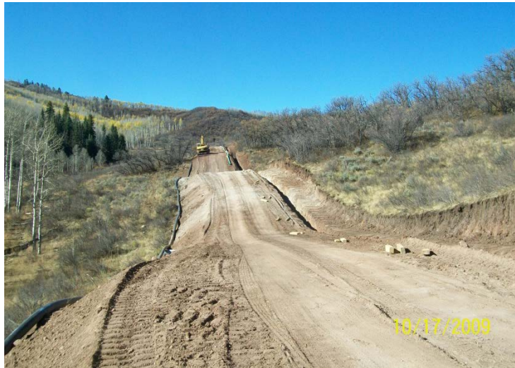
Photo 3: Pipeline trench parallel (co-located) to existing road
