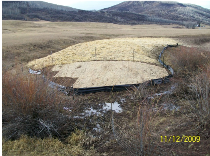
Photo 1: Wetland area with narrowed corridor following reclamation and replanting with local native species, per ACOE guidance [SPK-2009-01336].
