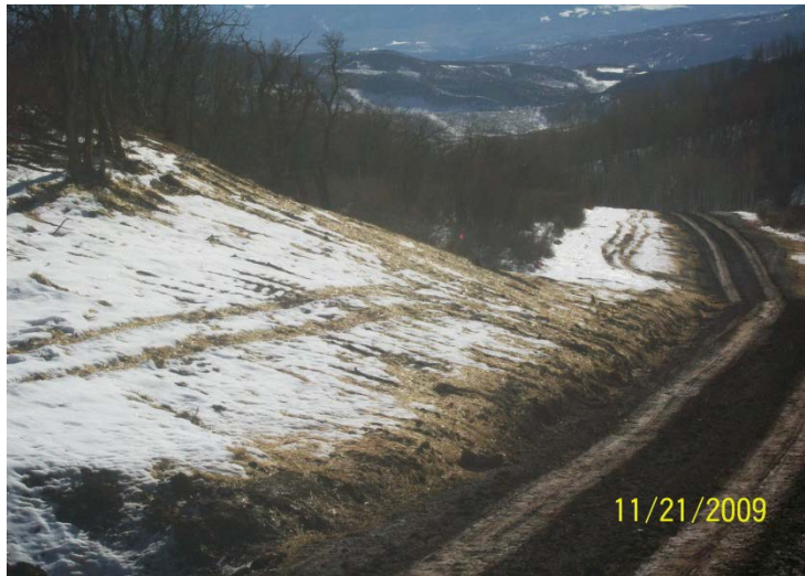
Photo 4: Reclaimed pipeline corridor adjacent to road
