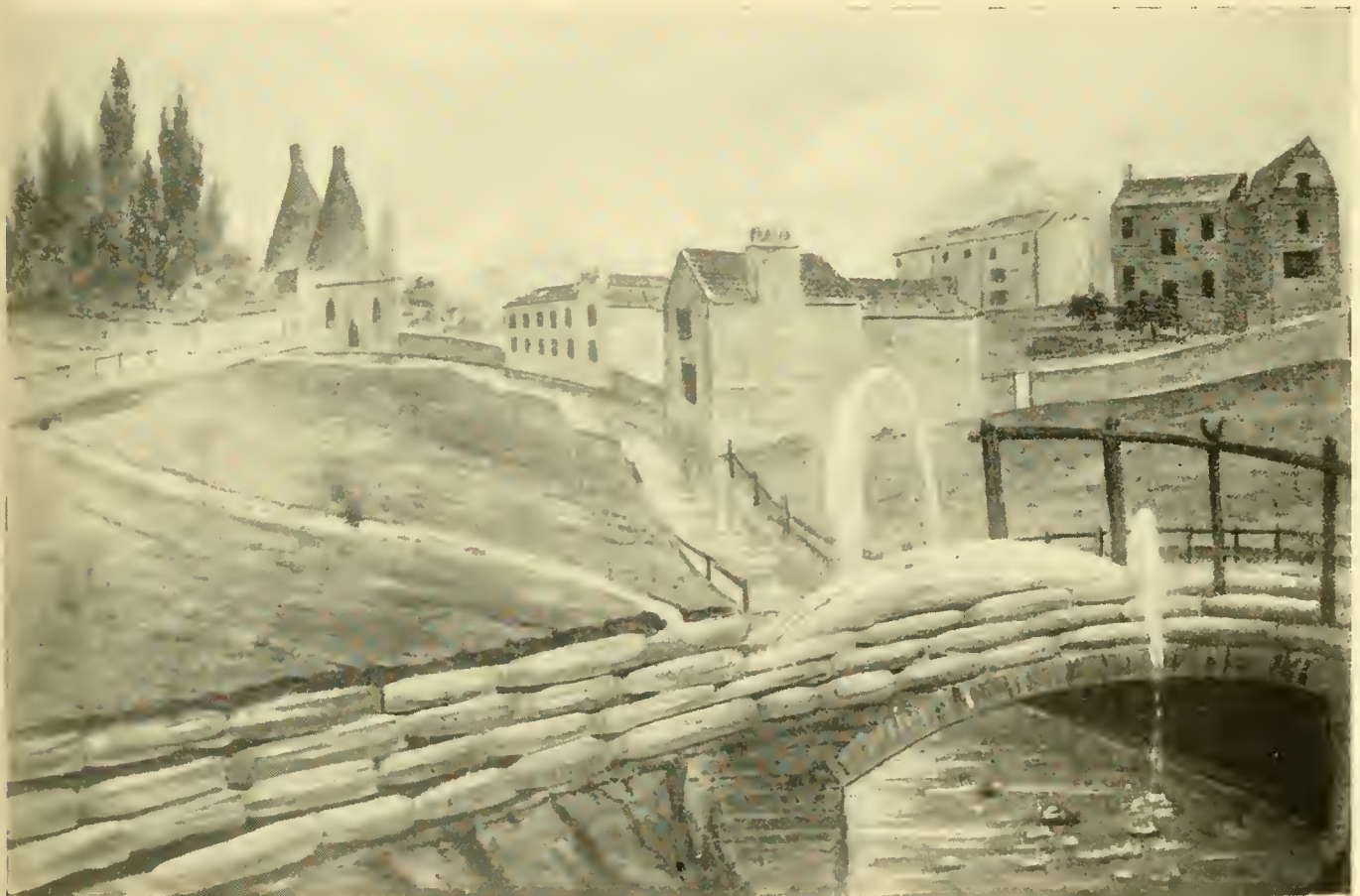
1. WOODEN WATER-MAINS IN COLD BATH FIELDS.
