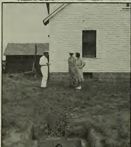
A Kansas farmer constructs a septic tank.
