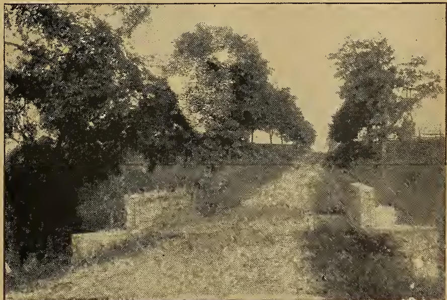
Concrete makes an elegant and substantial culvert bridge. Many of the small steel bridges of Columbiana County, Ohio, are built up into lasting structures by encasing the steelwork in cement. This is a picture of one of these.
