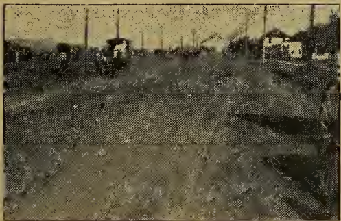
The loose earth in the center of the road has driven the traffic to the ditches
