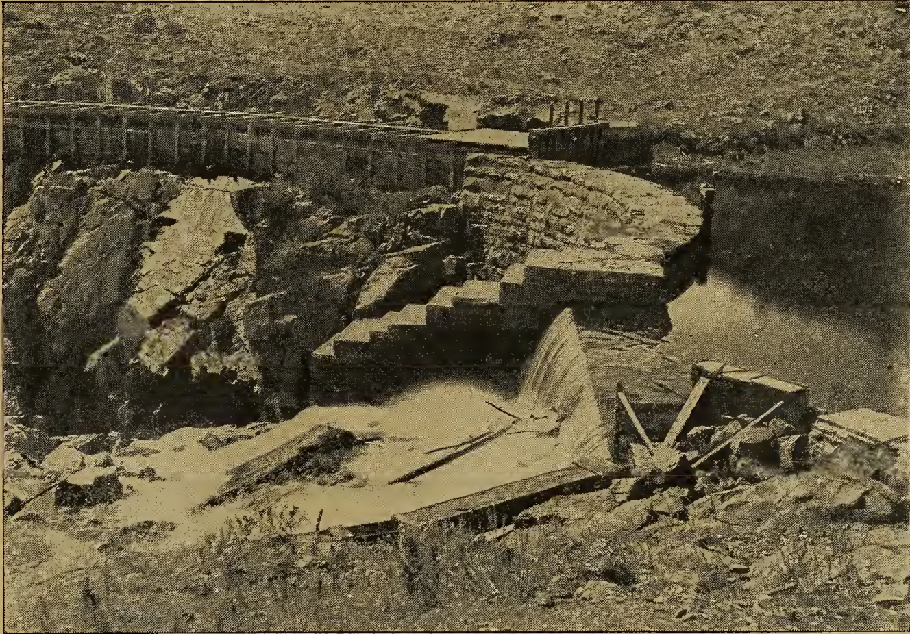
Diversion works of a canal in southern Colorado
