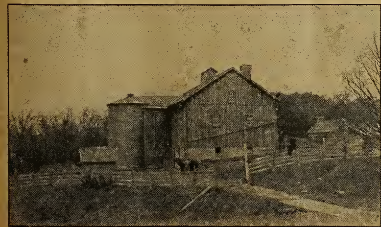
A silo makes the feeding methods practical
