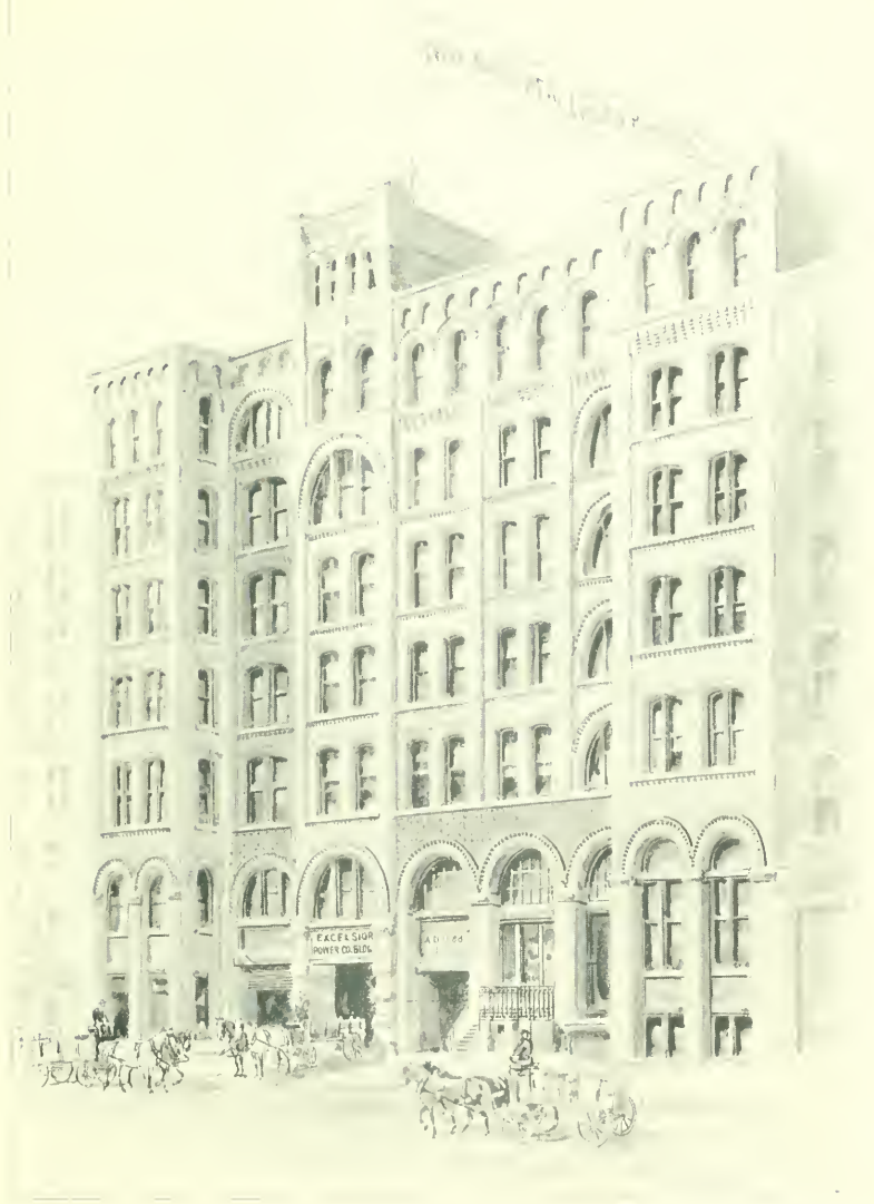
NEW YORK HEAT, LIGHT AND POWER COMPANY. GOLD STREET, WEST SIDE, BETWEEN FULTON AND JOHN STREETS.
