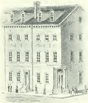
FIRST BUILDING. 1812.—THE BANK OF AMERICA.
