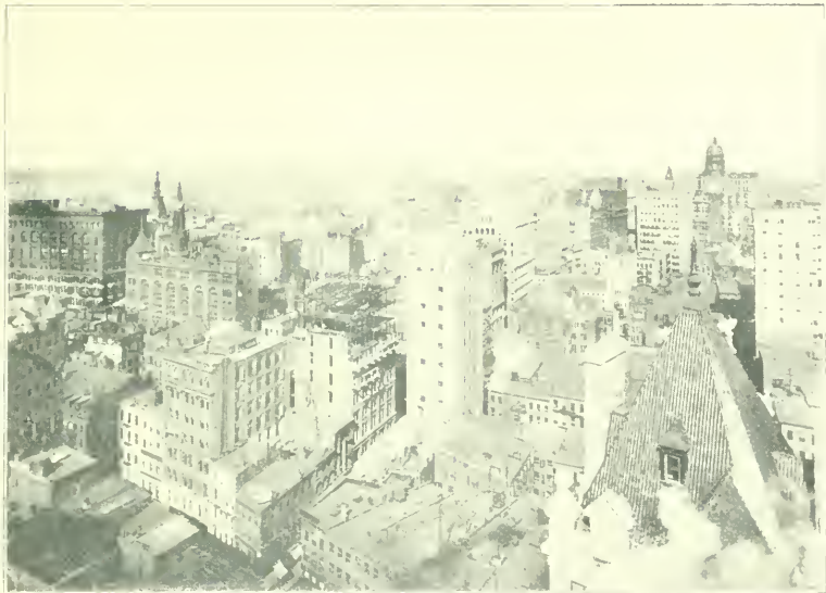
NORTHWEST VIEW FROM TOWER OF MUTUAL LIFE BUILDING. MUTUAL LIFE INSURANCE COMPANY, NASSAU LIBERTY AND CEDAR STREETS.
