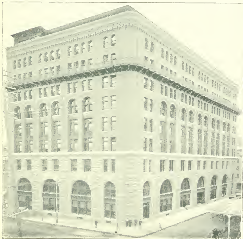
CENTRAL BUILDING, CENTRAL RAILROAD OF NEW JERSEY. LIBERTY AND WEST STREETS (NORTH RIVER), NEW YORK.
