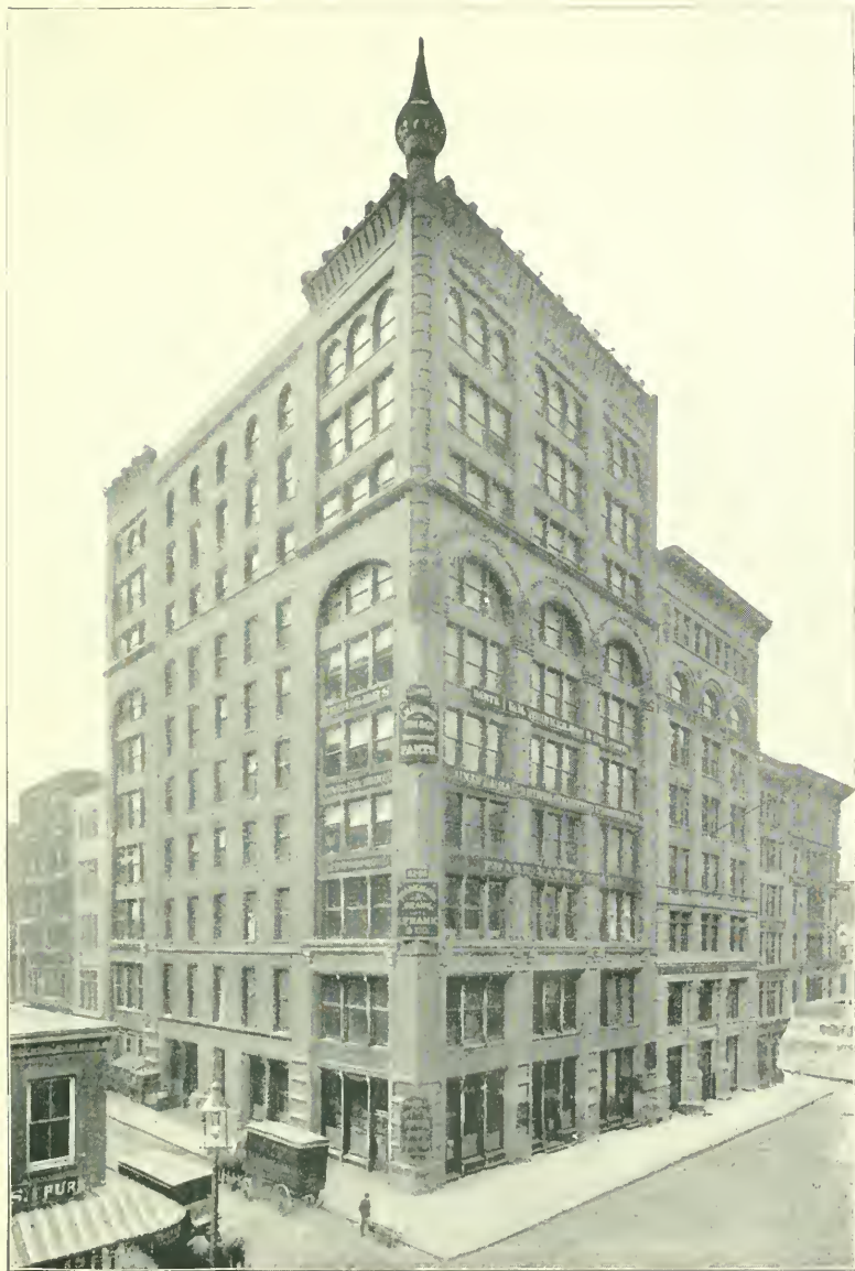
THE BLEECKER STREET BUILDING OF THE O. B. POTTER TRUST. BLEECKER STREET, SOUTHWEST CORNER OF WOOSTER STREET.
