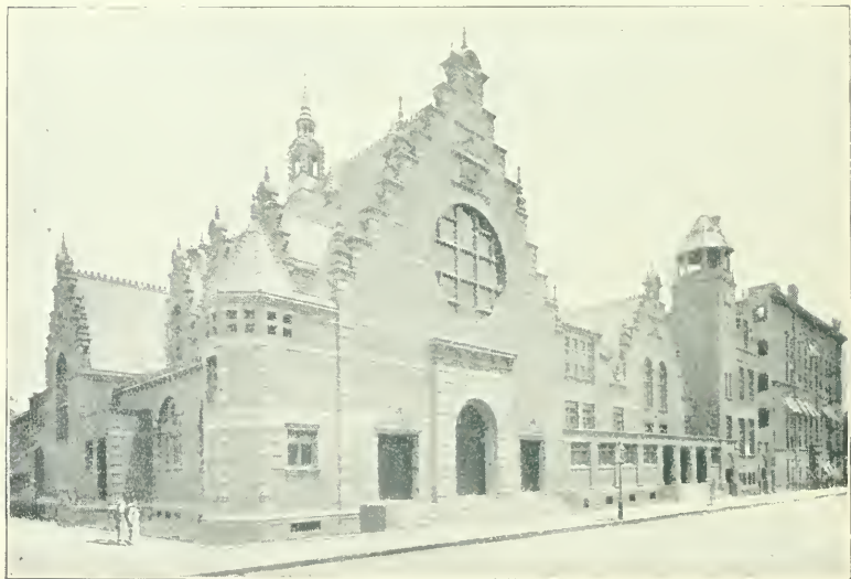
COLLEGIATE REFORMED CHURCH. WEST END AVENUE AND 77TH STREET.
