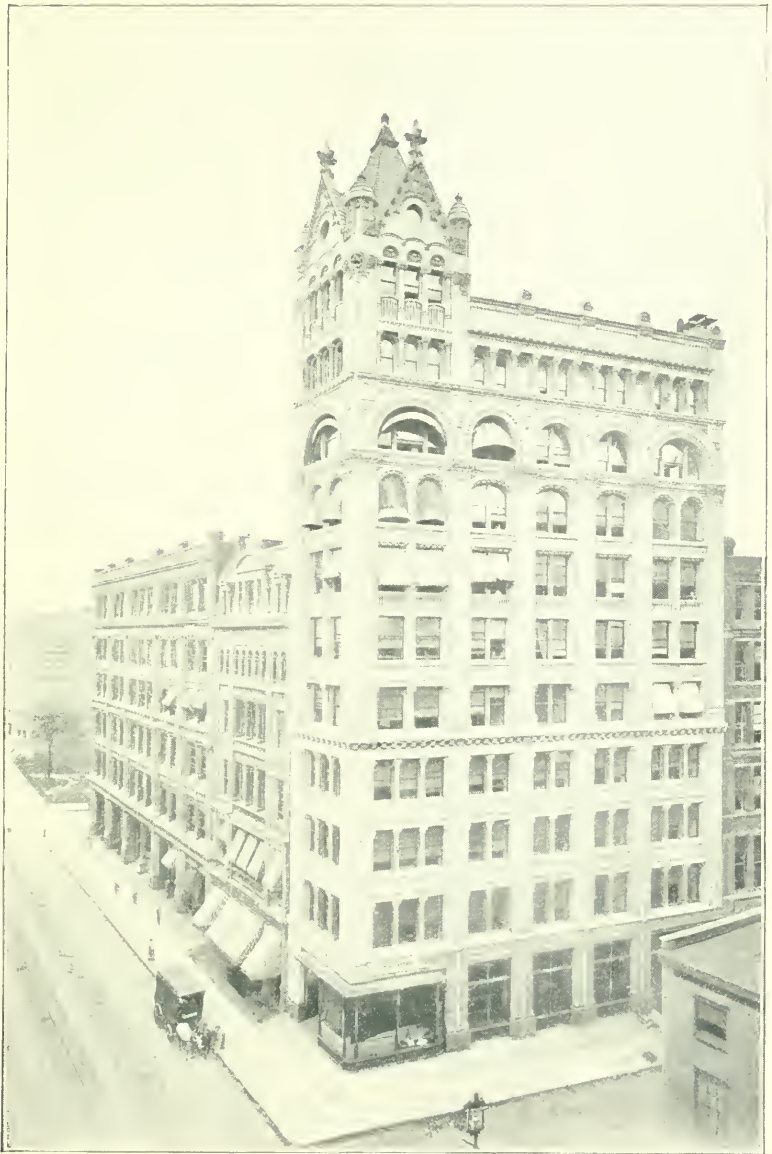
THE MCINTYRE BUILDING. BROADWAY, NORTHEAST CORNER OF 18TH STREET.
