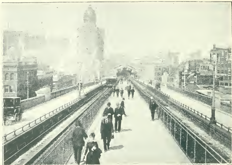
CABLE CARS ON THE EAST RIVER BRIDGE. VIEW OF NEW-YORK END, LOOKING TOWARD NEW YORK.
