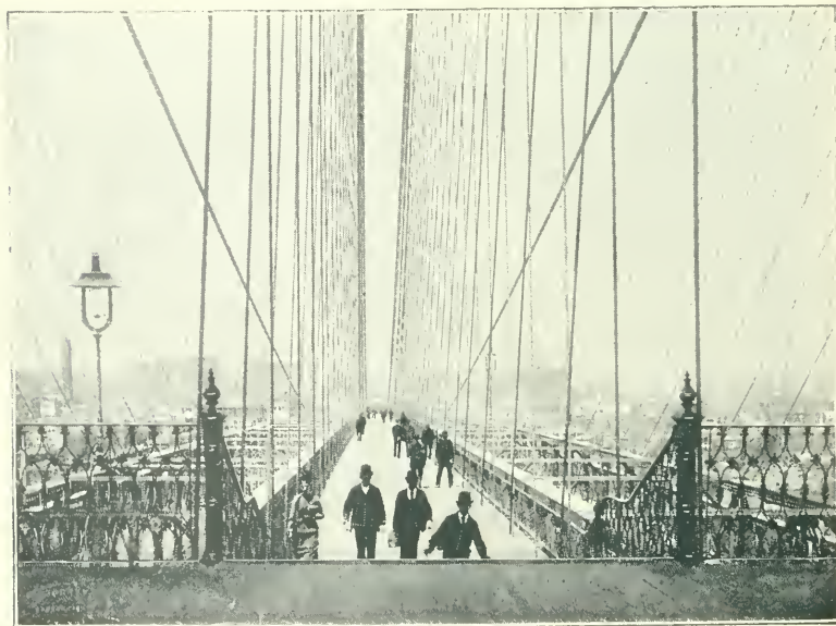
BROOKLYN BRIDGE PROMENADE. VIEW LOOKING TOWARD NEW YORK.
