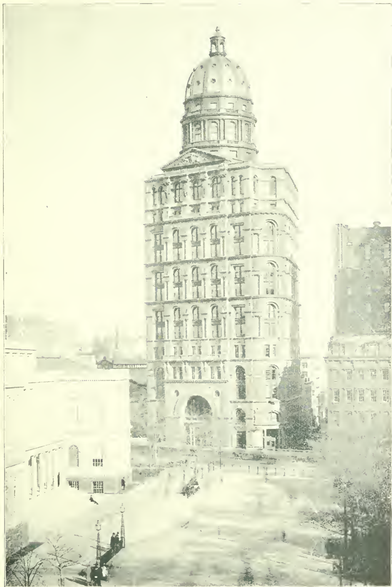
THE "WORLD" BUILDING, PARK ROW AND FRANKFORT STREET. AS SEEN FROM BROADWAY, ACROSS CITY HALL PARK.
