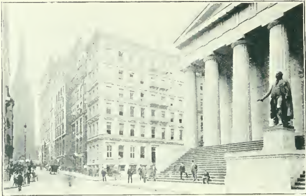
WALL STREET. NORTH SIDE, FROM THE SUB-TREASURY TO TRINITY CHURCH.
