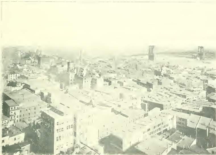
NORTHEAST VIEW FROM TOWER OF MUTUAL LIFE BUILDING. MUTUAL LIFE INSURANCE COMPANY, NASSAU, LIBERTY AND CEDAR STREETS.
