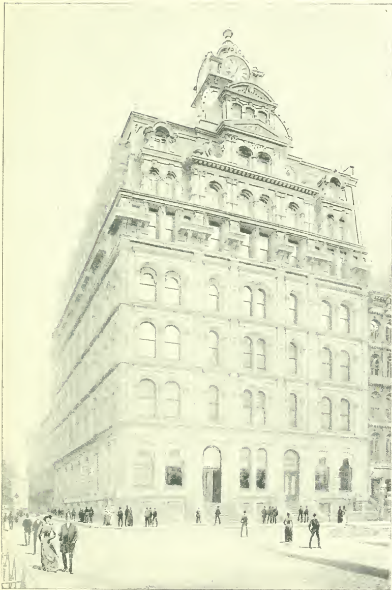
MUTUAL LIFE BROADWAY BUILDING. BROADWAY, SOUTHEAST CORNER LIBERTY STREET.
