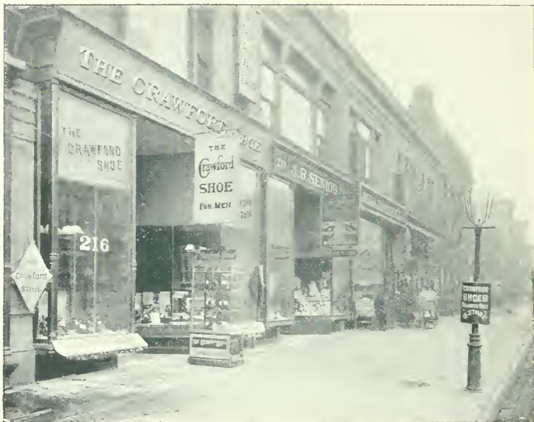
THE CRAWFORD (HARLEM) SHOE STORE, No. 216 WEST 125TH STREET, BETWEEN SEVENTH AND EIGHTH AVENUES.
