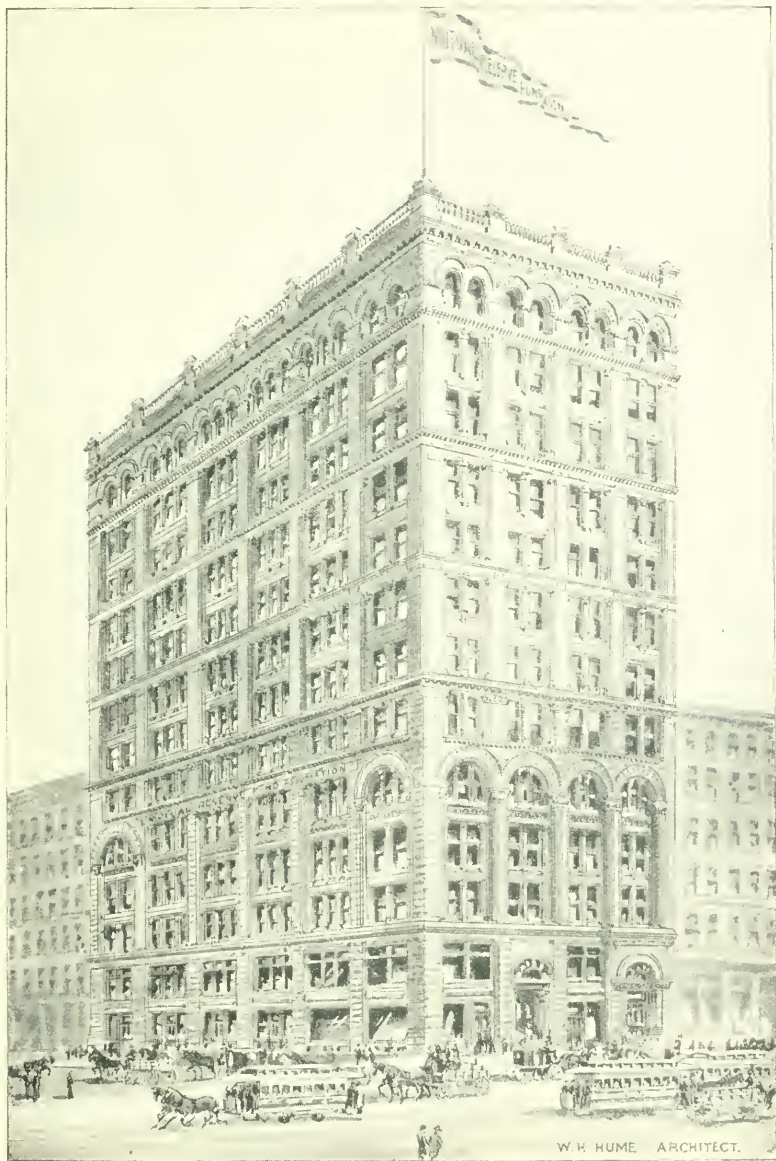
MUTUAL RESERVE FUND LIFE ASSOCIATION. MUTUAL RESERVE BUILDING, BROADWAY, NORTHWEST CORNER OF DUANE STREET.
