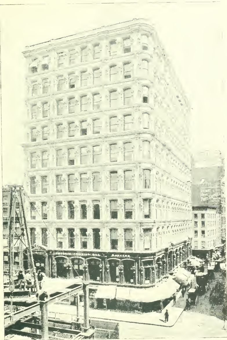
LAWRENCE, FRAZIER & CO., BANKERS. BENNETT BUILDING, NASSAU STREET, NORTHWEST CORNER OF FULTON STREET.
