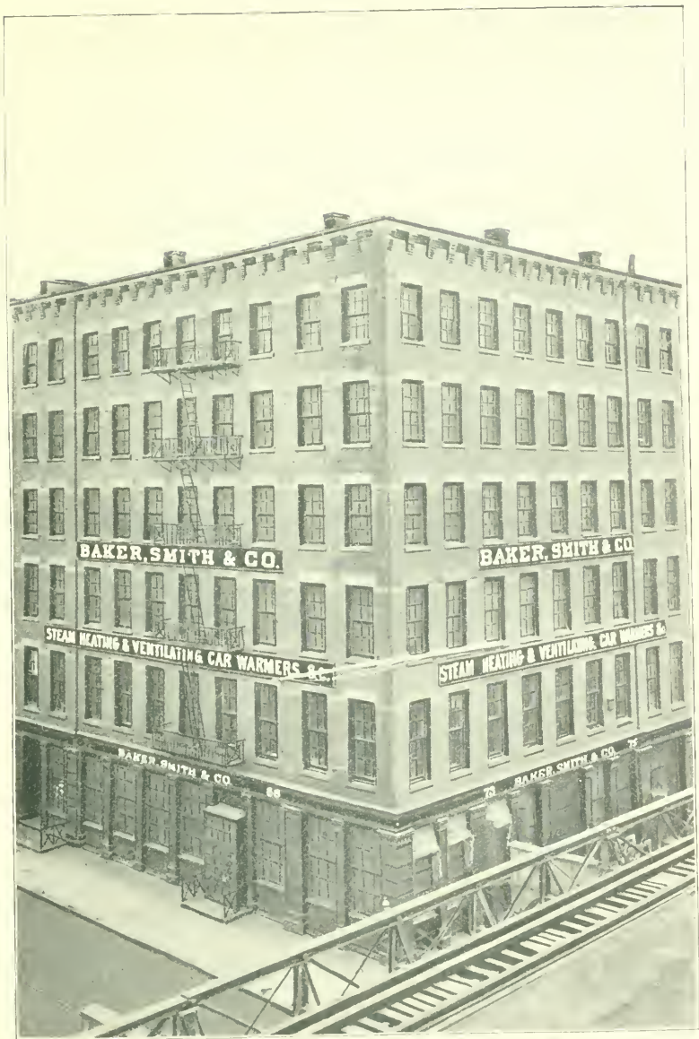
BAKER, SMITH & CO., HEATING AND VENTILATING APPARATUS. SOUTH FIFTH AVENUE, SOUTHEAST CORNER HOUSTON STREET.
