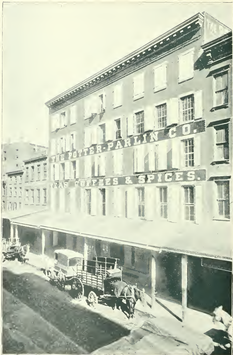
READE STREET FRONT.
