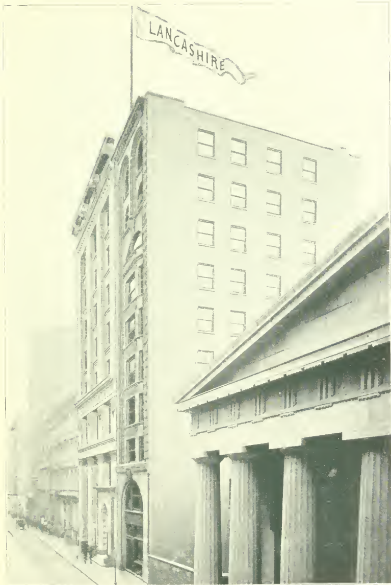
LANCASHIRE INSURANCE COMPANY OF MANCHESTER, ENGLAND. LANCASHIRE BUILDING, No. 25 PINE STREET, ADJOINING UNITED STATES SUB-TREASURY.
