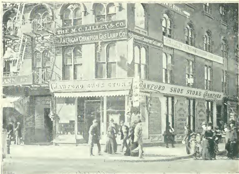
CRAWFORD SHOE STORE. BROADWAY, SOUTHWEST CORNER OF 12TH STREET.
