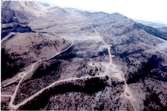
Main LHTA Road Network Looking South Showing Range Support Facility
