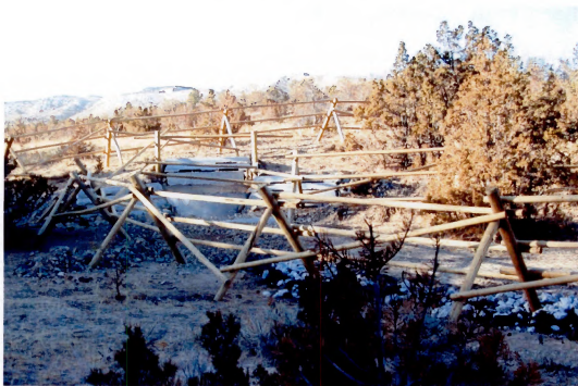
Stock Watering Tank Runoff Channel
