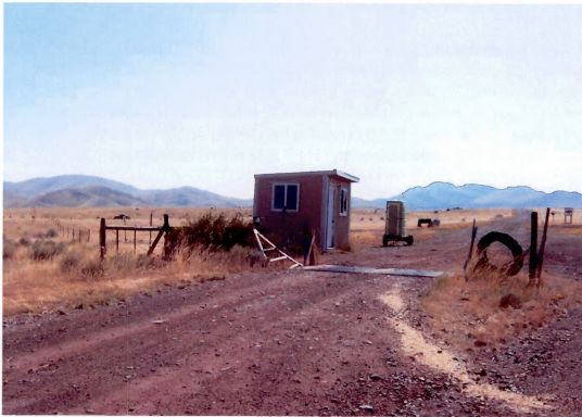
North Gate Guard Shack
