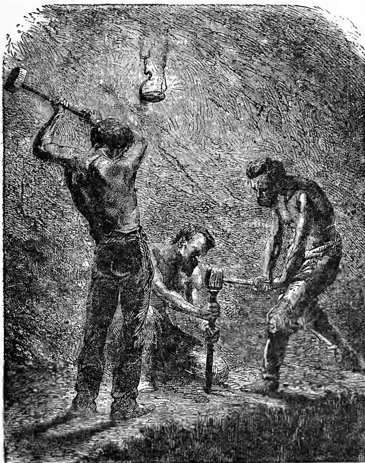
MINING LIFE.—BORING A BLAST HOLE.
