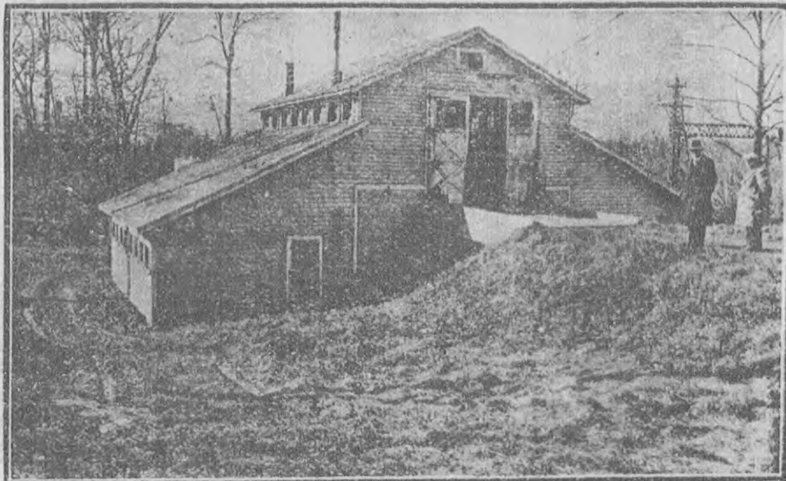
8-Cell Beccari Plant from the North Showing Charging Floor At top of Cells. Scarsdale, Wetchester County, New York.
