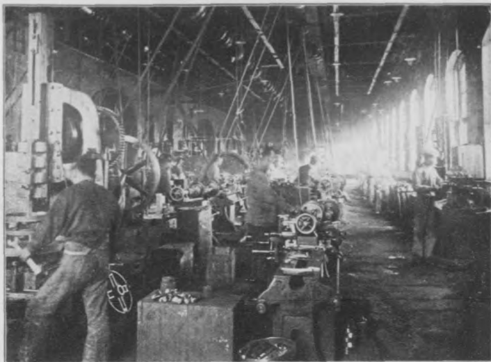
No. 1 Workshop, Shibaura Engineering Works.
