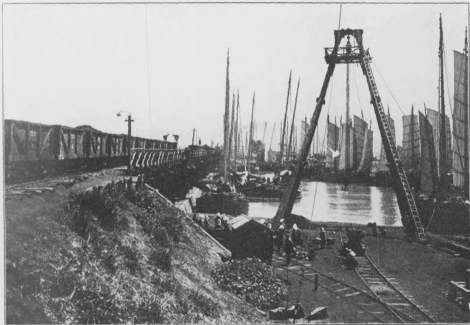
Wet Dock for Coal Loading, Miike Colliery.
