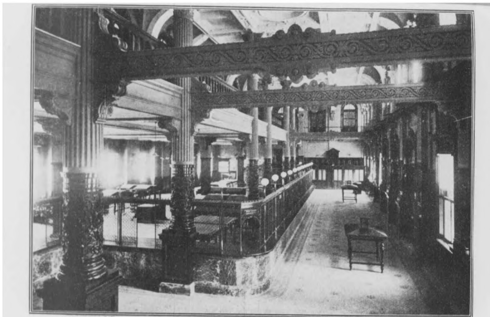
景内行總行銀井三 An Interior of the Main Office of Mitsui Bank at Tokio.
