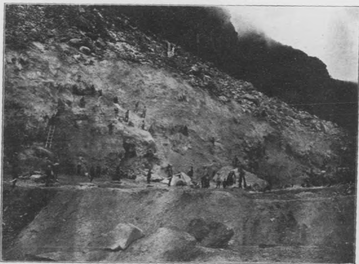
Mining Sulphur Ore by Open Work at Tsurugishita, Tsurugizan Mine.
