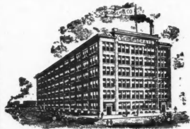
FACTORY 132 ND TO 133 RD ST & BROOK AVE
