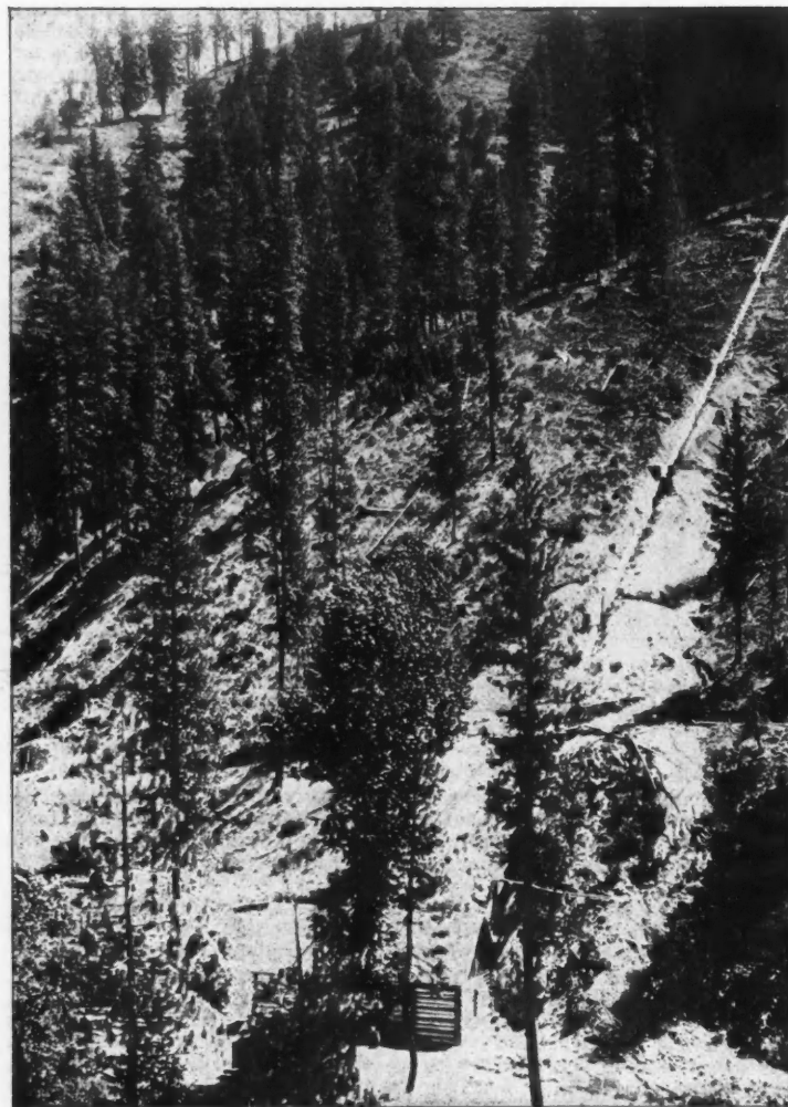
PIPE LINE, BED ROCK DREDGING COMPANY, IDAHO.
