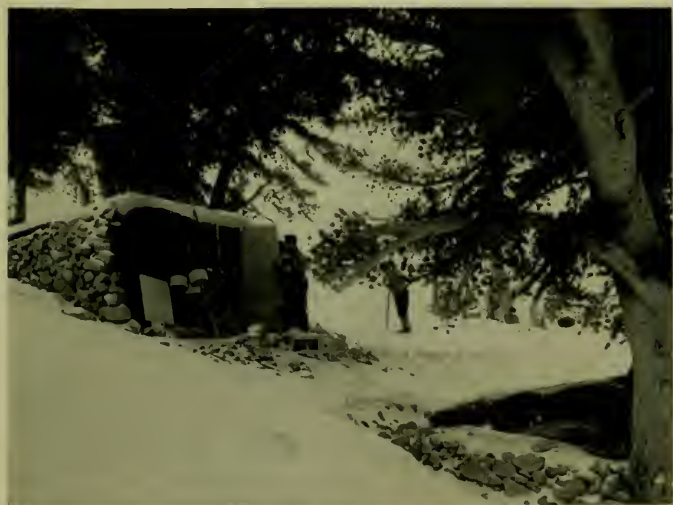
REFUGE HUT AND HEADQUARTERS FOR SNOW STUDIES, ON MT. ROSE, 9000 FEET
