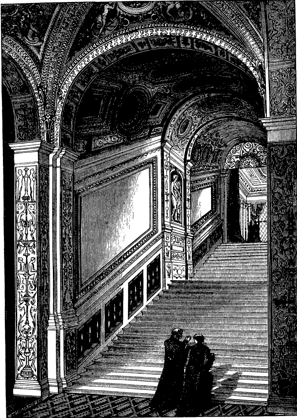
GRAND STAIRCASE IN THE DUCAL PALACE.
