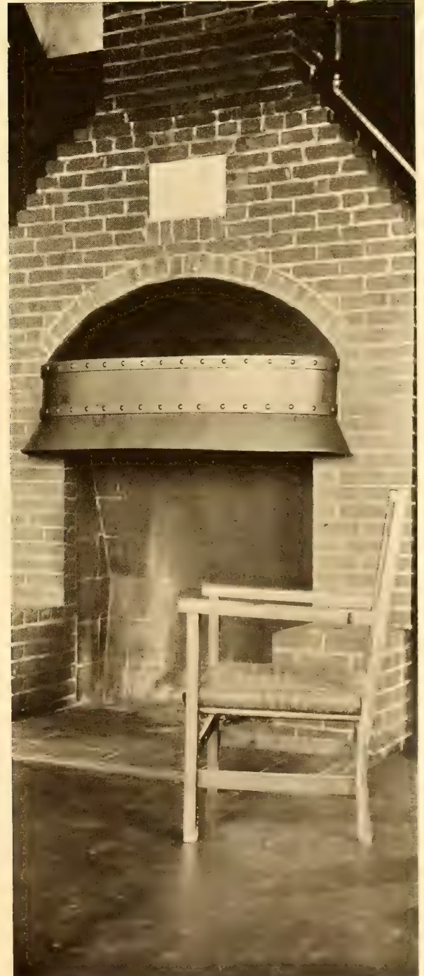
The Fireplace in the Living-room Is Built of Common Brick and Has a Hood of Hammered Iron
