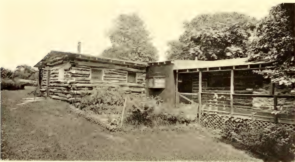
Ties in Their Natural Silver Gray and Posts and Trim Painted Green
