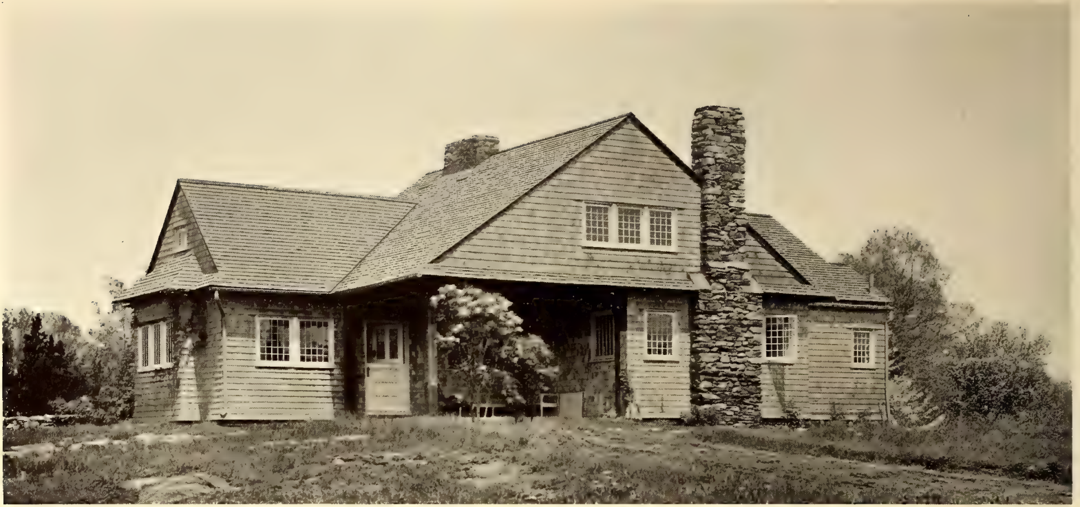
Fieldstone and Natural Shingle Form the Exterior Walls of the House
