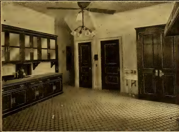
Kitchen Showing Interlocking Rubber Tiling in Residence of Mr. Webb Horton, Middleton, N. Y.
