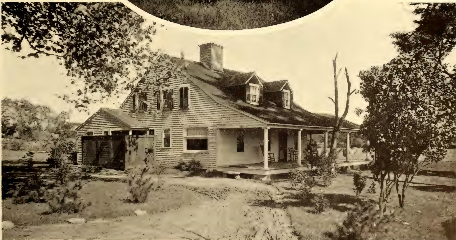
"Shing-wak": The Home of Thomas Alsop, Esq., Showing the House Before and After the Alteration
