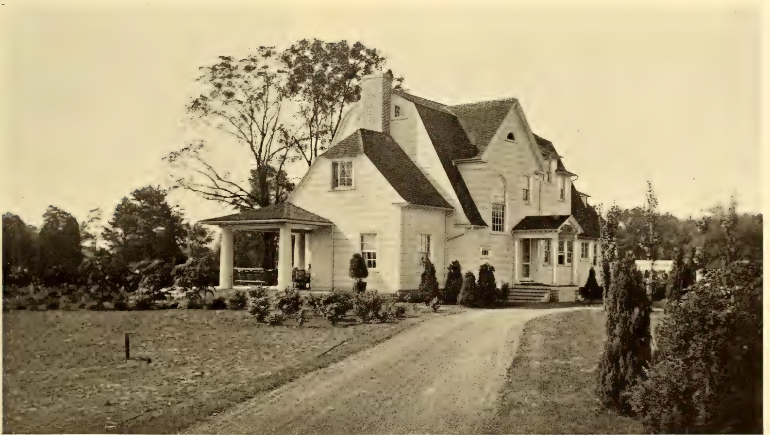
The Exterior of the House Is Covered with Hand-riven Cypress Shingles Painted White
