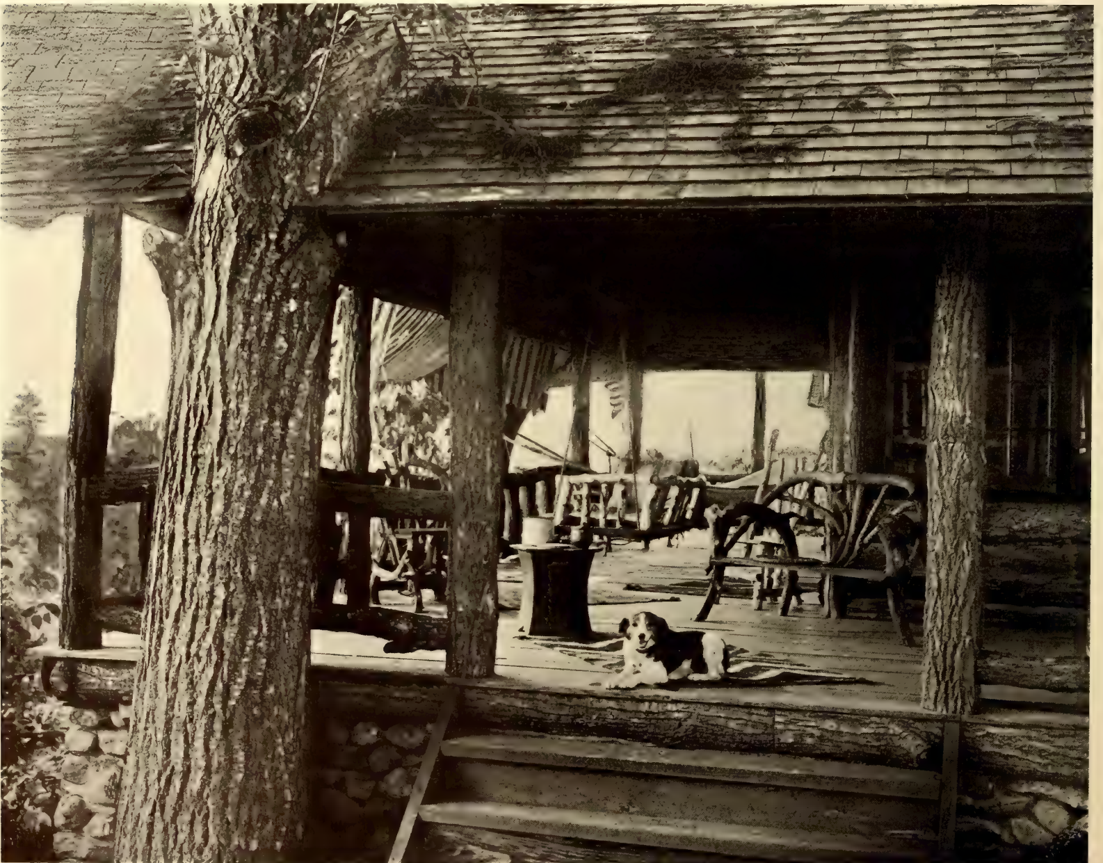
The Rough Irregular Surface of Locust Logs Is Admirable for the Rustic Work of the Piazza
