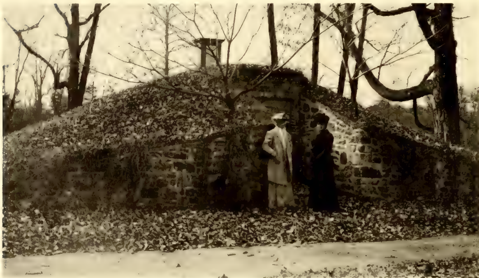
Dome-shaped Spring-House at Andalusia
