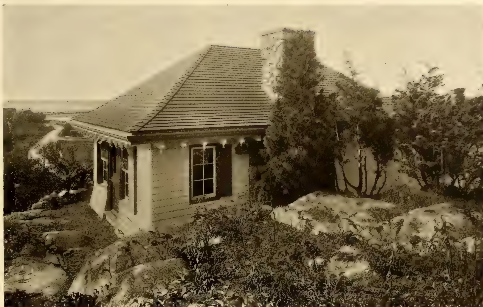
The Overhanging Roof Is Thickly Set with Electric Lights
