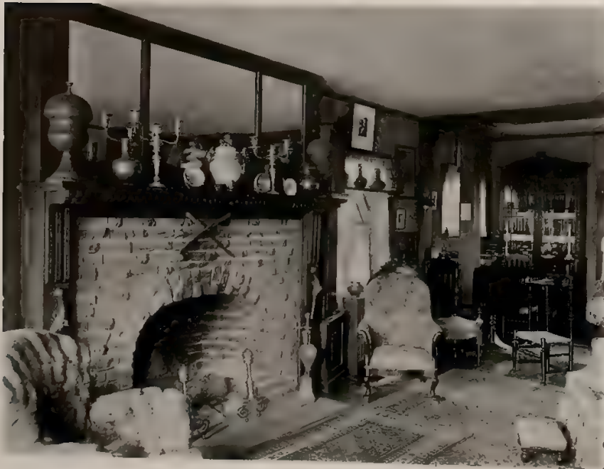
The living-room has an open fireplace of klinker brick
