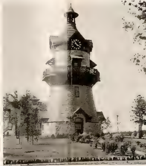
Clock and Water Tower
