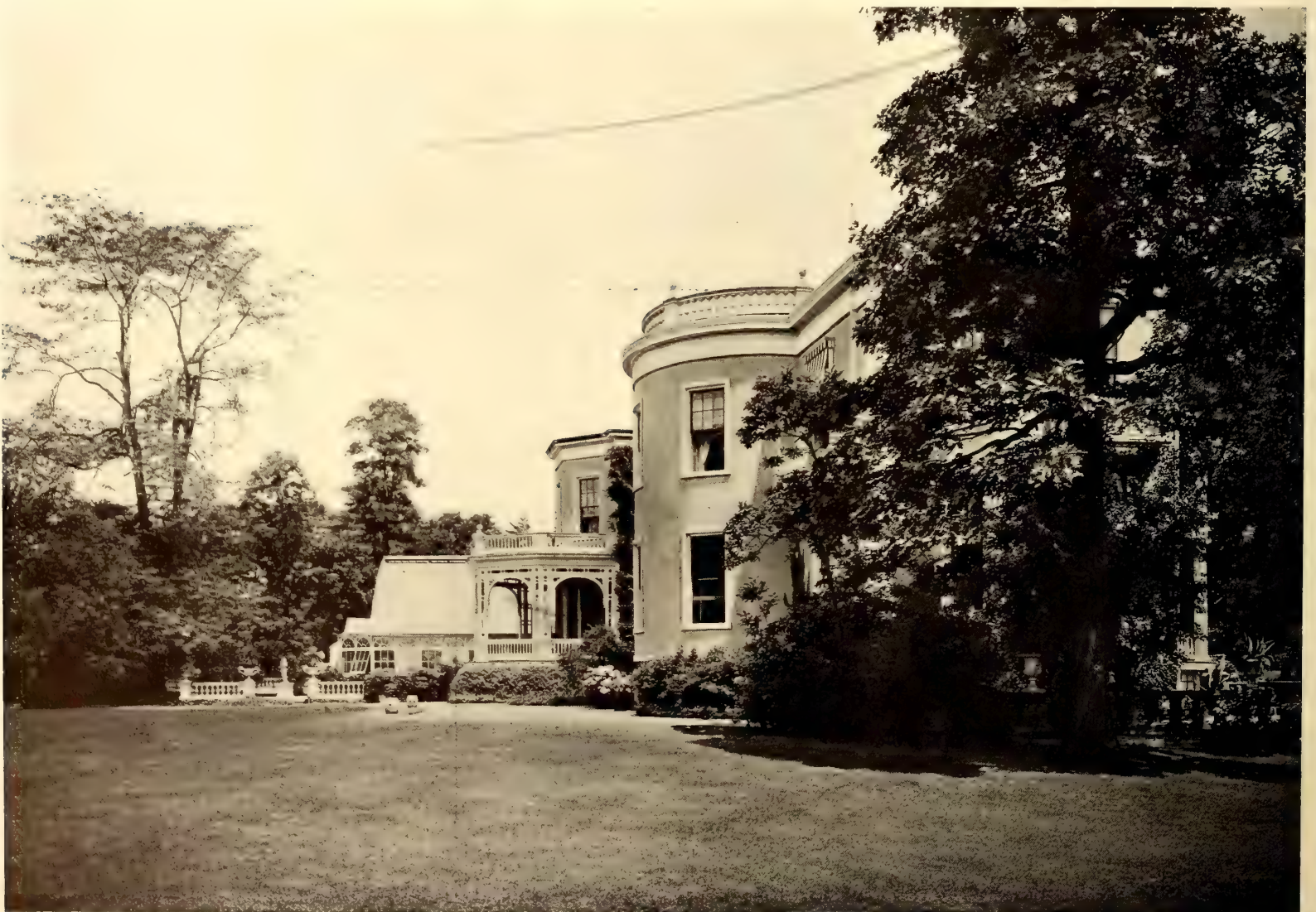
The House, Porch, Conservatory and Terrace Are Handsomely Grouped Amid a Massing of Trees, Some of which Are of True Forest Growth
