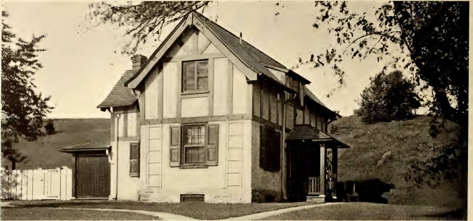
Stucco and Half Timber Are Always Interesting
