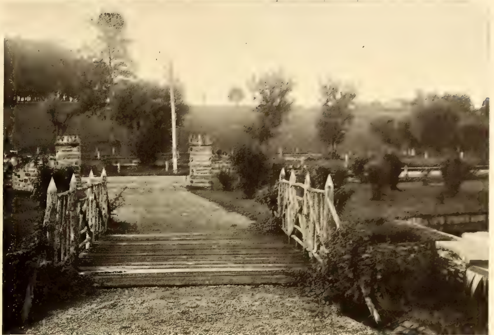
Bridge Roadway with Rustic Railing
