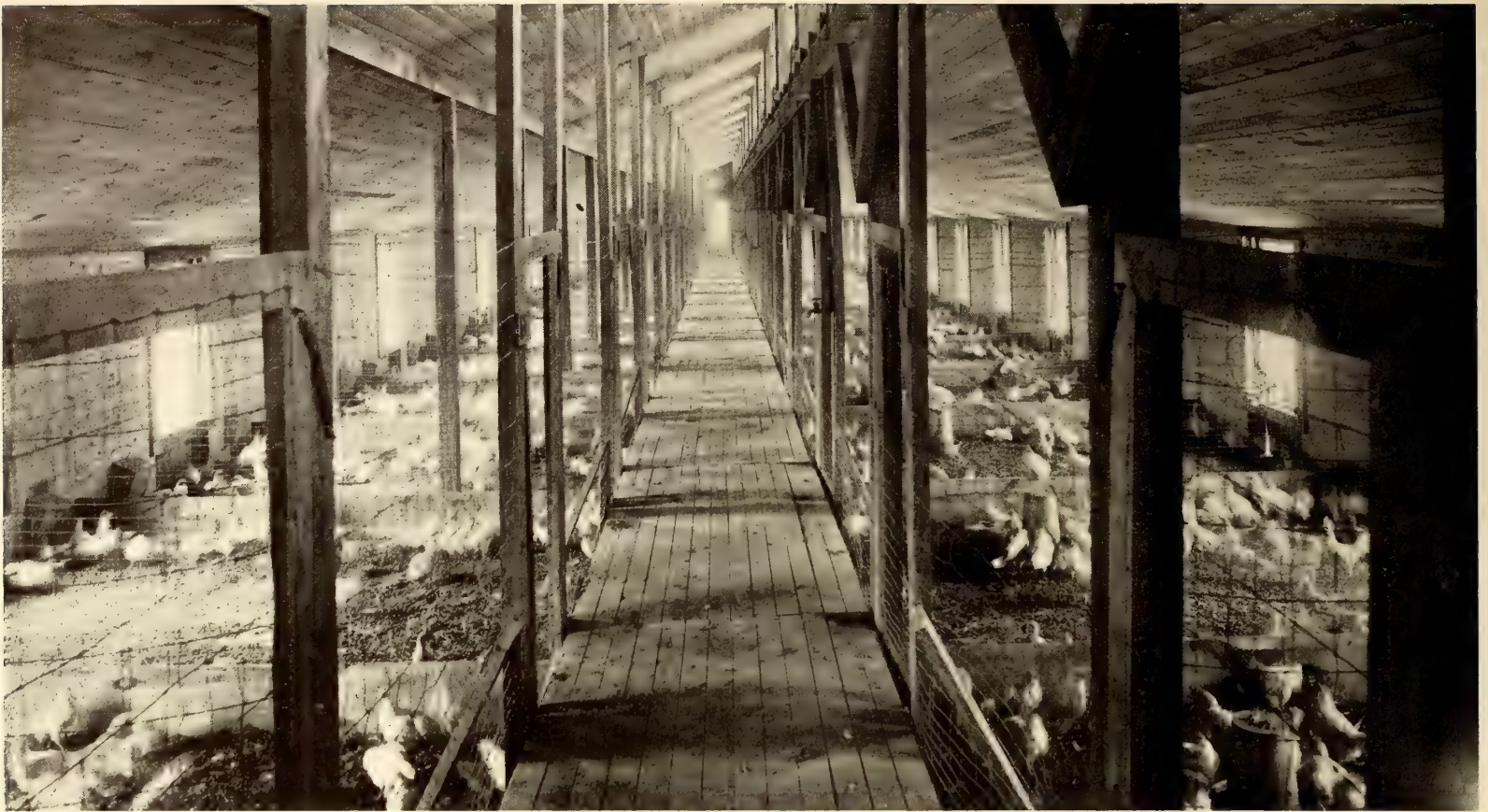
Interior View of the Chicken House
