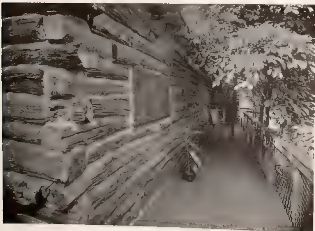
The Porch Above the Creek
