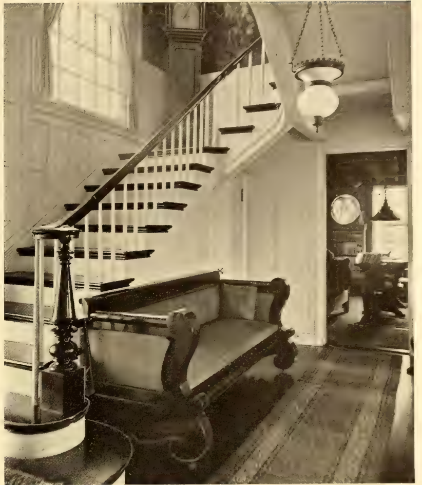
The Staircase Is a Handsome Feature of the Hall with Its Mahogany Treads and Rail and Its White Painted Balusters
