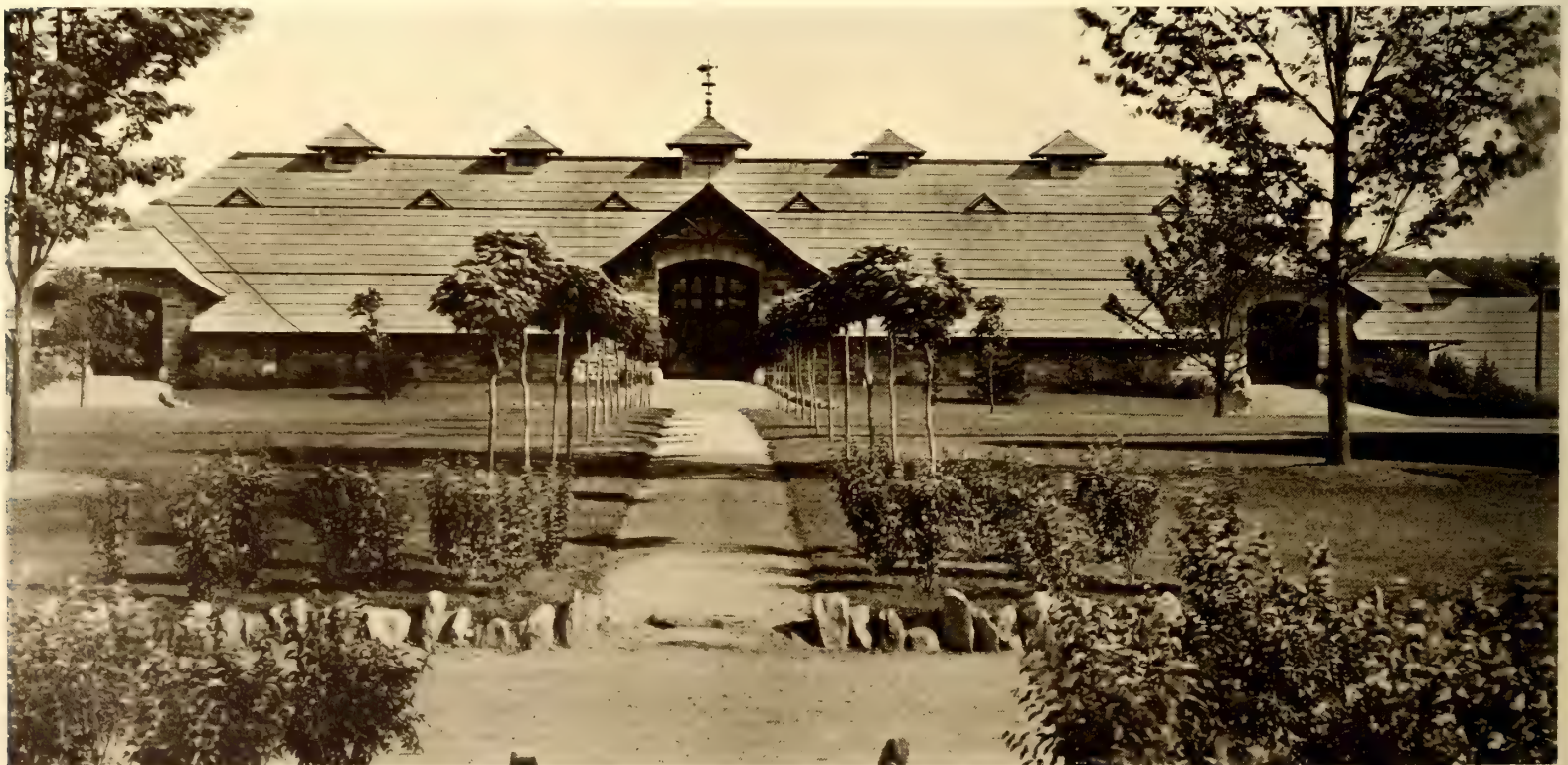
The Farm Barn Is Built of Stone with an Immense Shingled Roof
