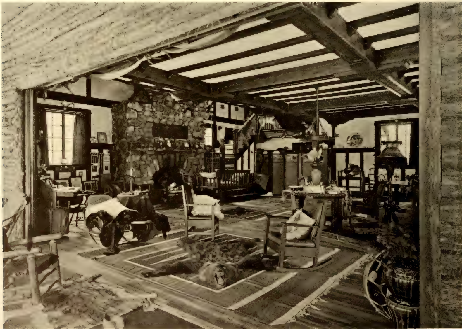
The Fireplace of the Living-room Is Built of Fieldstone Laid up at Random
