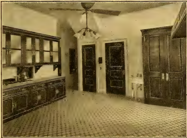
Kitchen Showing Interlocking Rubber Tiling in Residence of Mr. Webb Horton, Middleton, N. Y.
