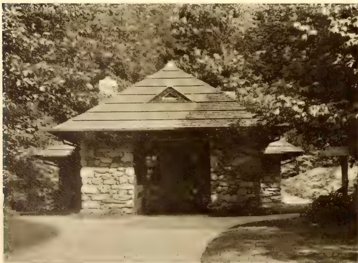
The Pump House for the Water Supply
