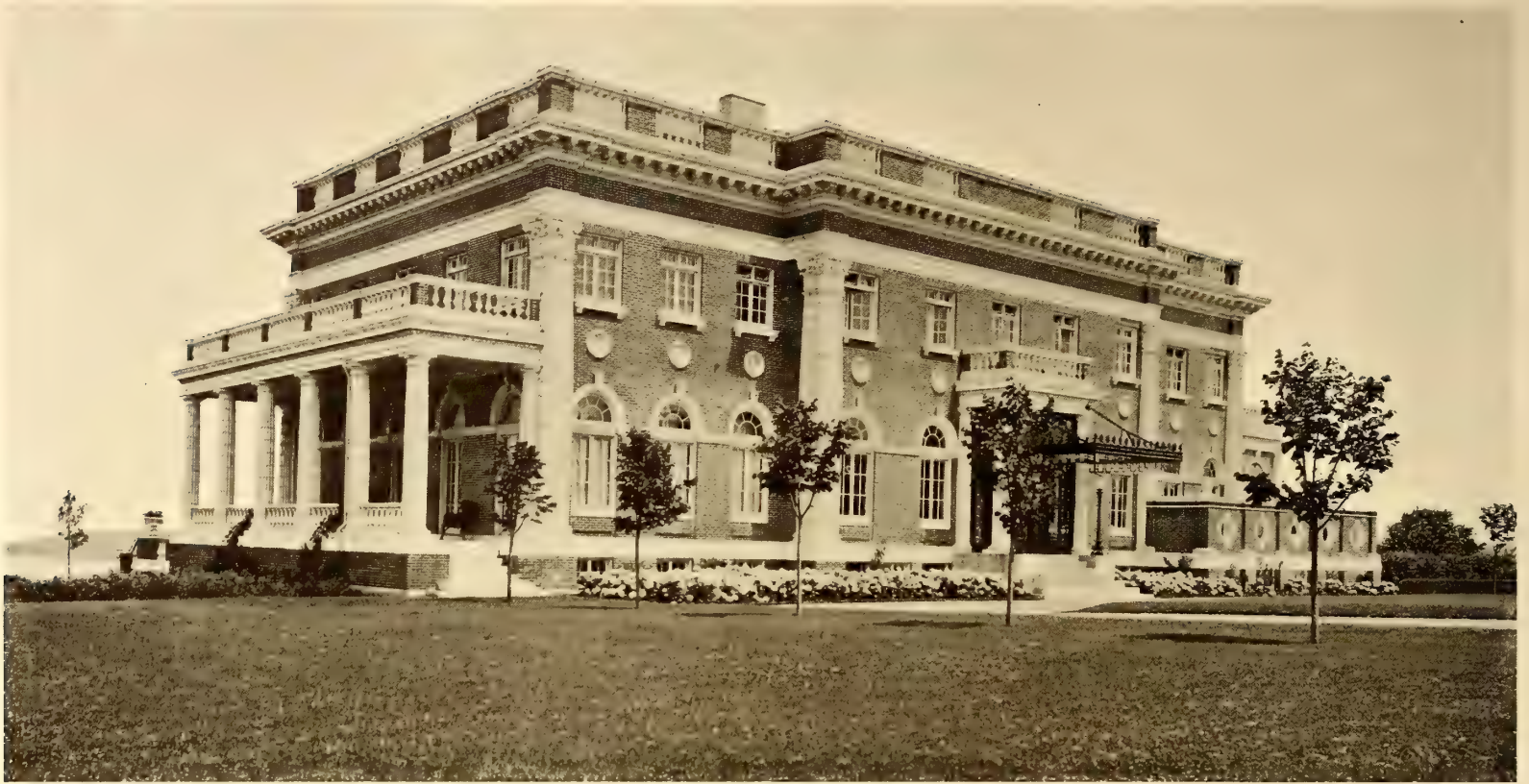
The House Is Built of Red Brick with White Glazed Terra Cotta Trim
