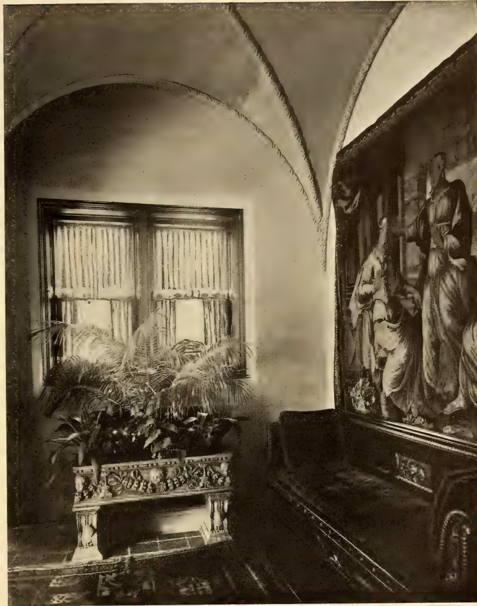
The Vestibule Is a Vaulted Chamber Walled with Stone
