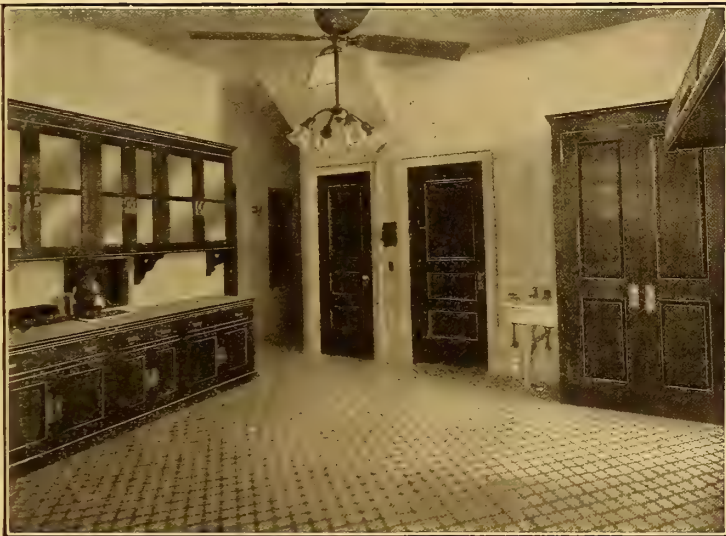
Kitchen Showing Interlocking Rubber Tiling in Residence of Mr. Webb Horton, Middleton, N. Y.
