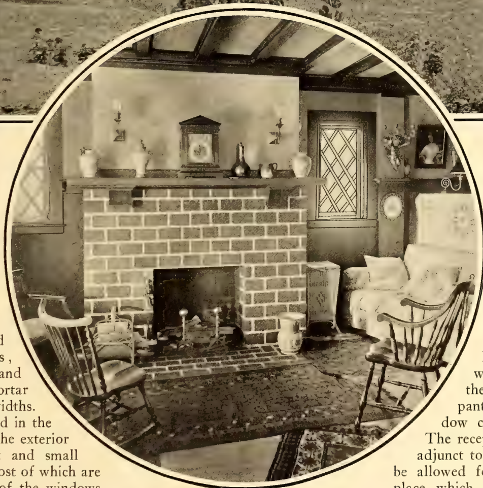
The Fireplace in the Living-room Is Built of Wire-cut Bricks Laid Edgewise
