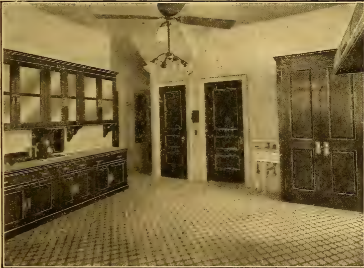
Kitchen Showing Interlocking Rubber Tiling in Residence of Mr. Webb Horton, Middleton, N. Y.
