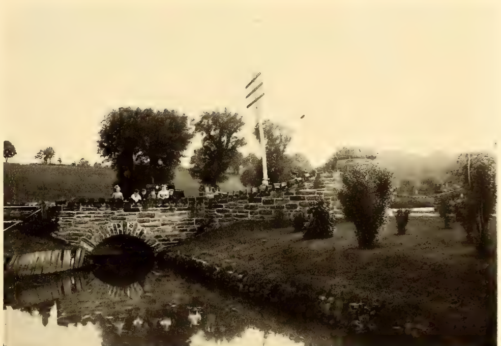
Entrance Bridge Across a Public Highway
