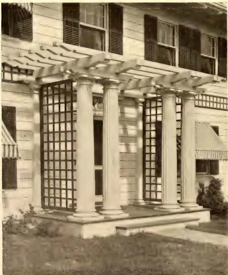
The Pergola-like Porch of the Entrance Door
