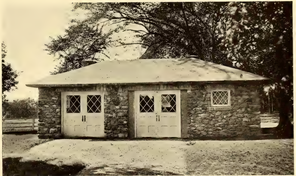
Exterior Walls of Field Stone Are Highly Effective
