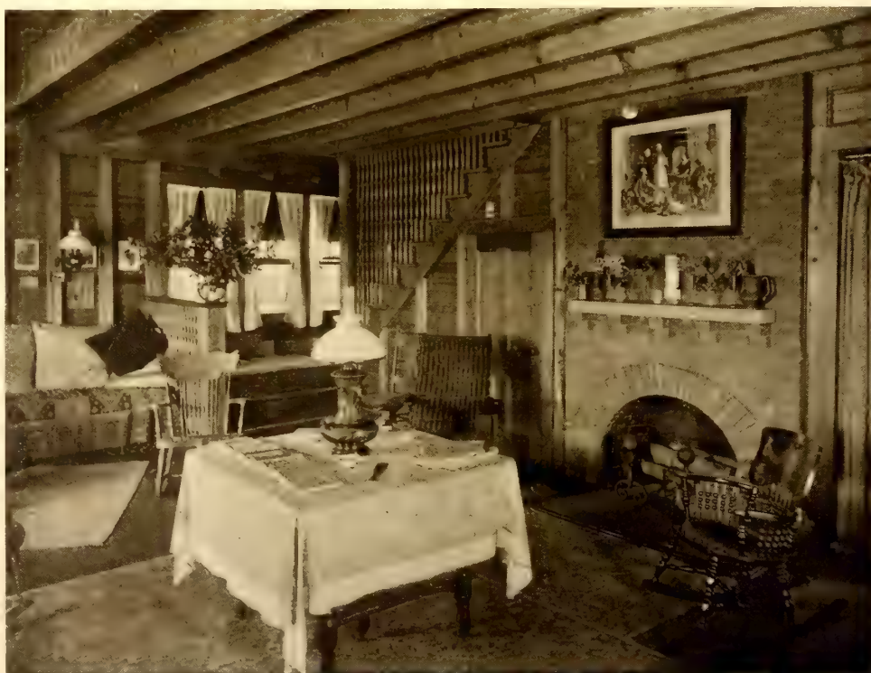
The studs and floor joists are exposed to view and are stained a soft brown color
