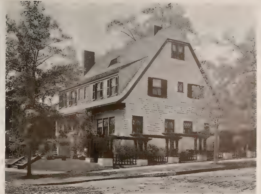
The pergola fence is an unusual and effective arrangement
