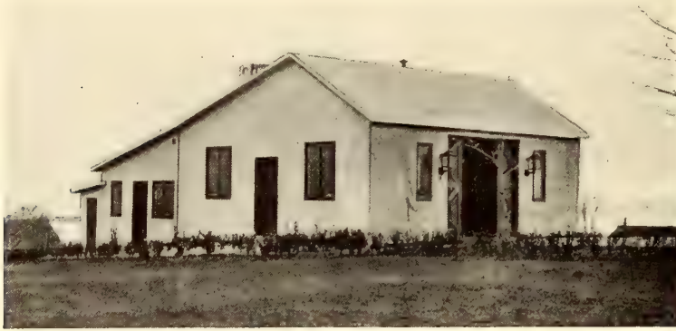
Garage with Three Rooms and Bath Attached for Chauffeur's Family Reinforced Concrete Throughout
