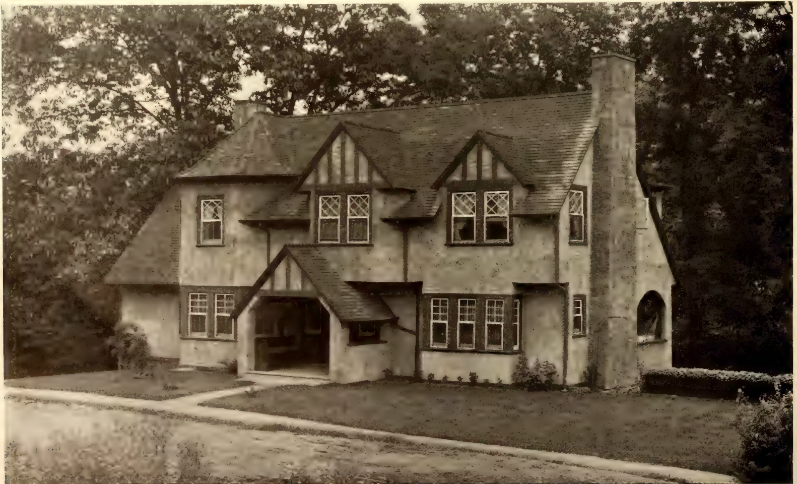
The House Is Built of Stucco from the Grade to the Peak, and the Whole Is Covered with a Shingled Roof Stained a Soft Green Tone
