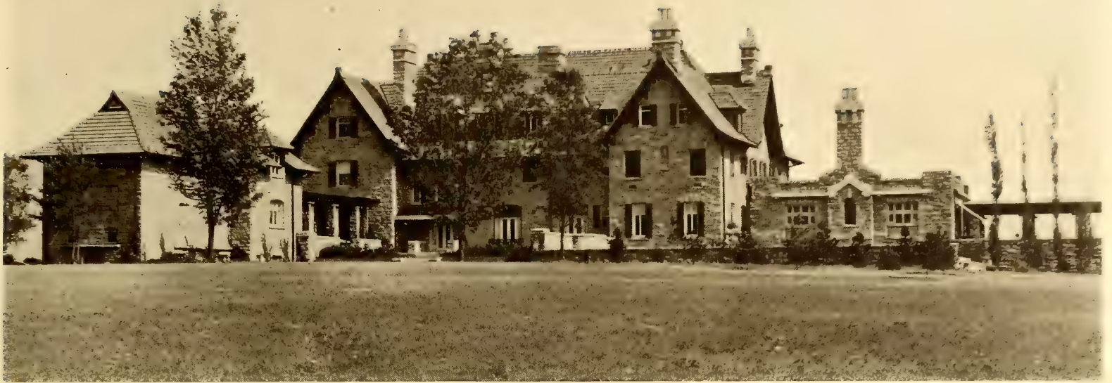
The Casino, Manor House and Dining-room
