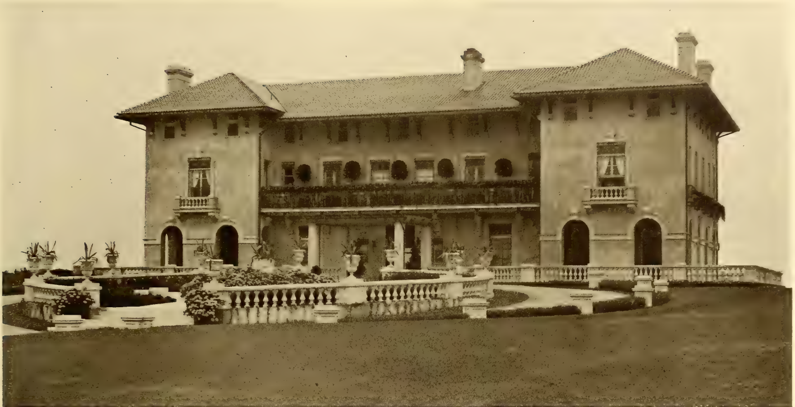
The House Is Built of Gray Stucco with Roof of Green Spanish Tiles
