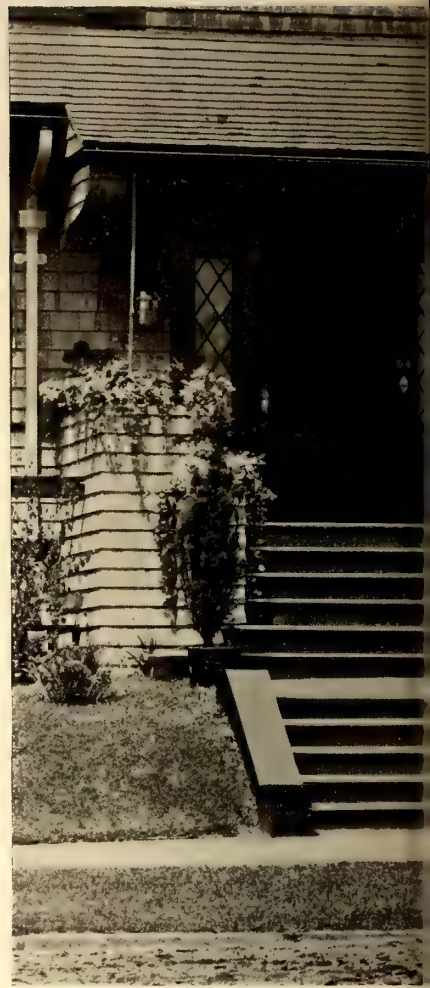
Flower boxes built in the buttress
