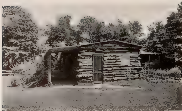
Seven Hundred Old Railway Ties Transformed Into a Bungalow
