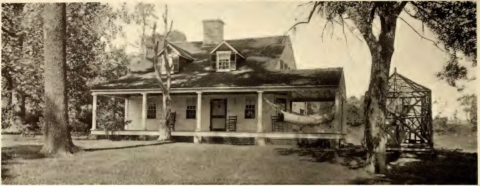
“Shing-wak”: A Piazza and Dormer Windows in the Roof Were the Exterior Alterations
