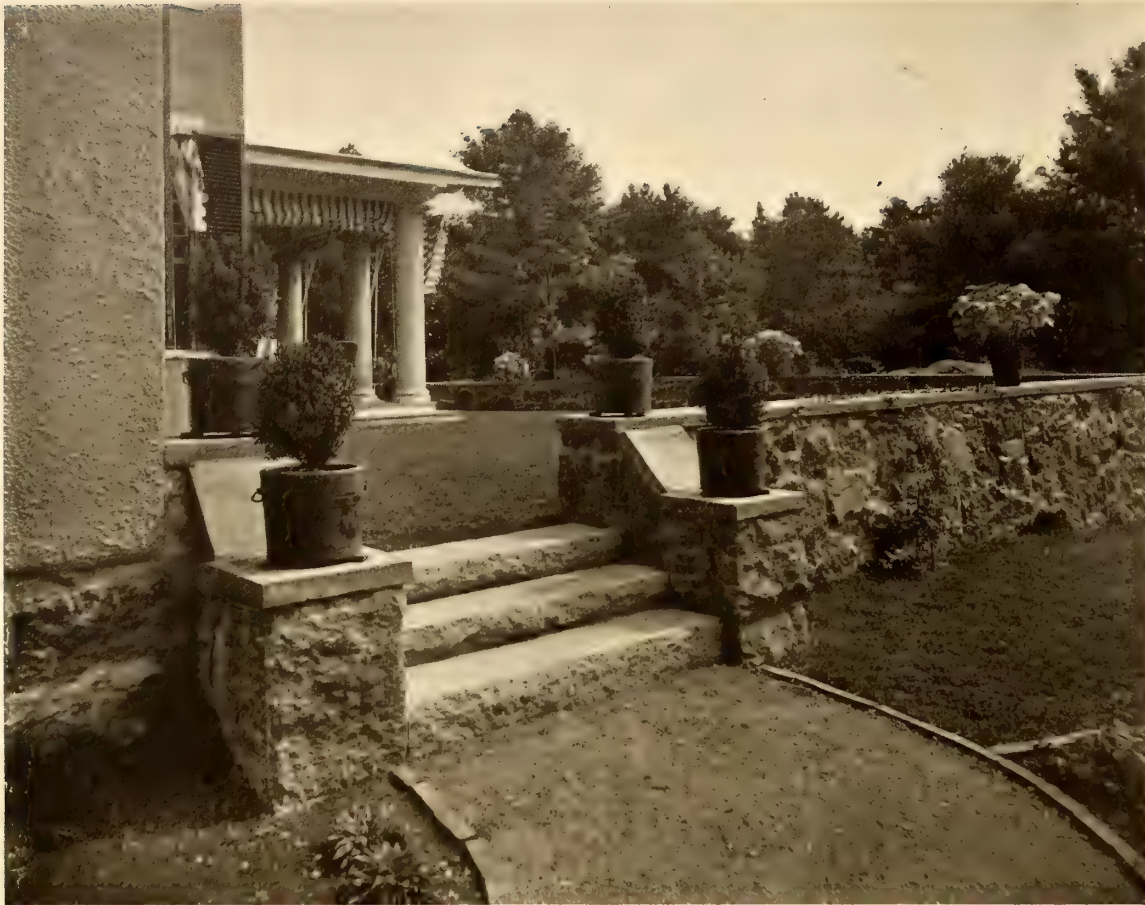
The Inner Porch Overlooks a Terrace Supported by Walls of Stone
