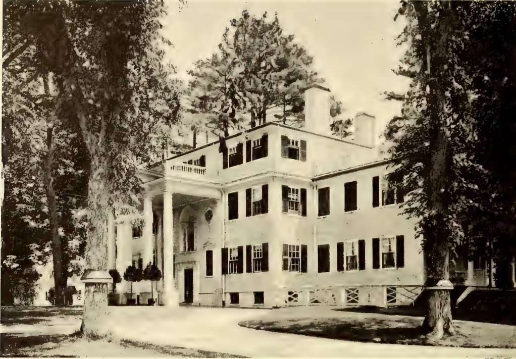
The House Is Typically Colonial in Design, Painted White, with Green Blinds
