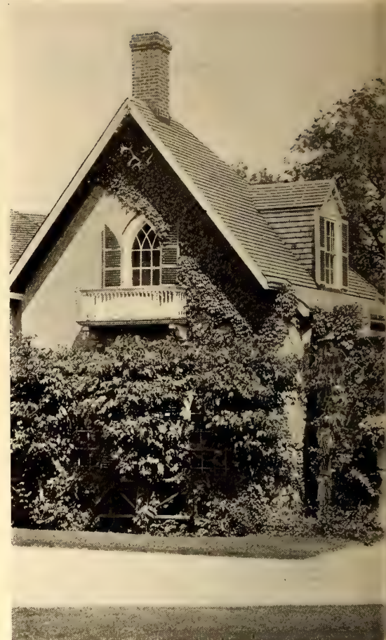
Much of the walls are smothered
