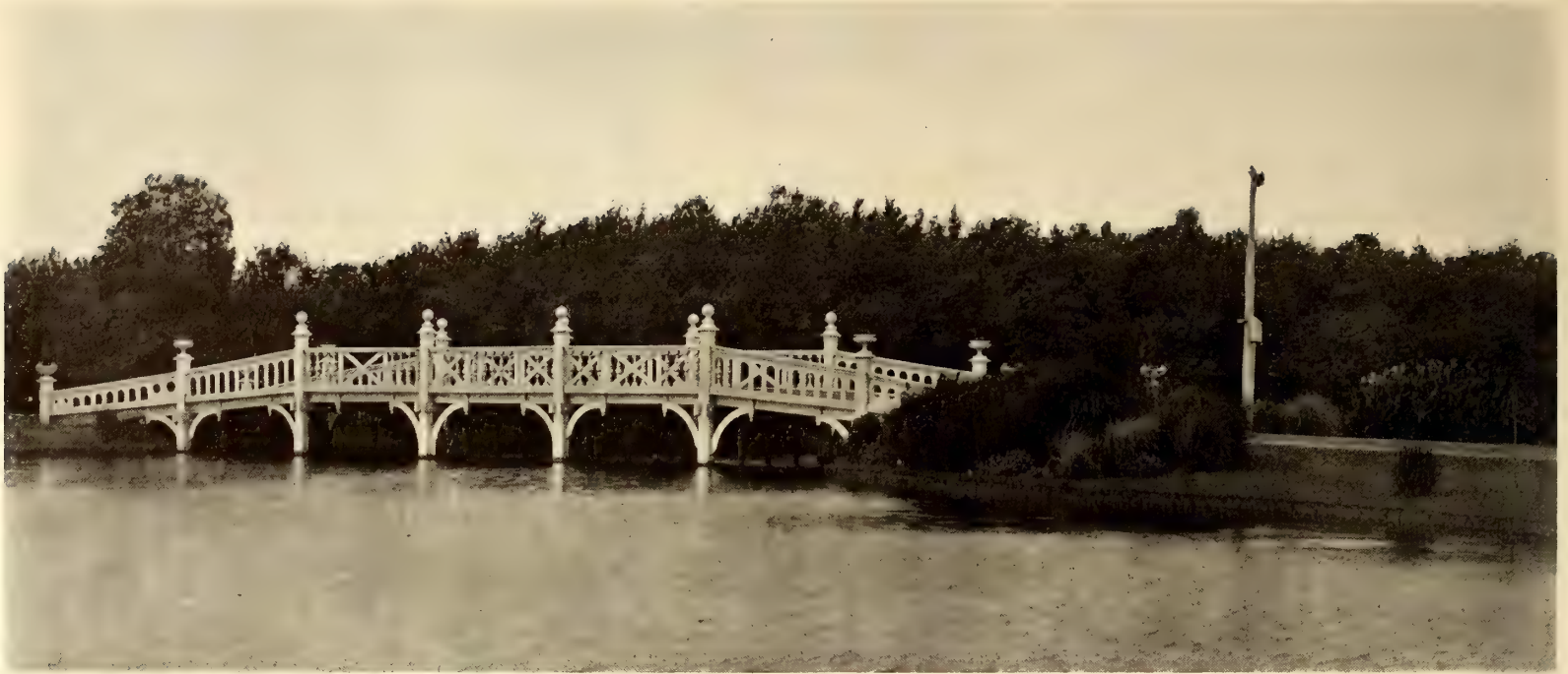
The Bridge and Abutments in a Water Park
