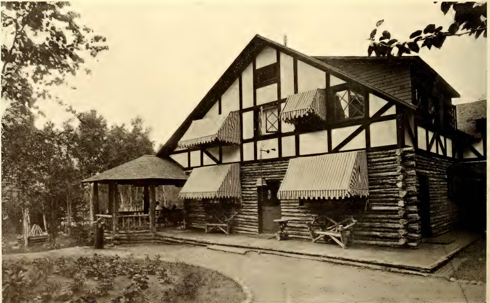
The First Story Is Built of Red Cedar Logs ; the Second Is Stuccoed with Exposed Timbers ; the Roof Is Shingled
