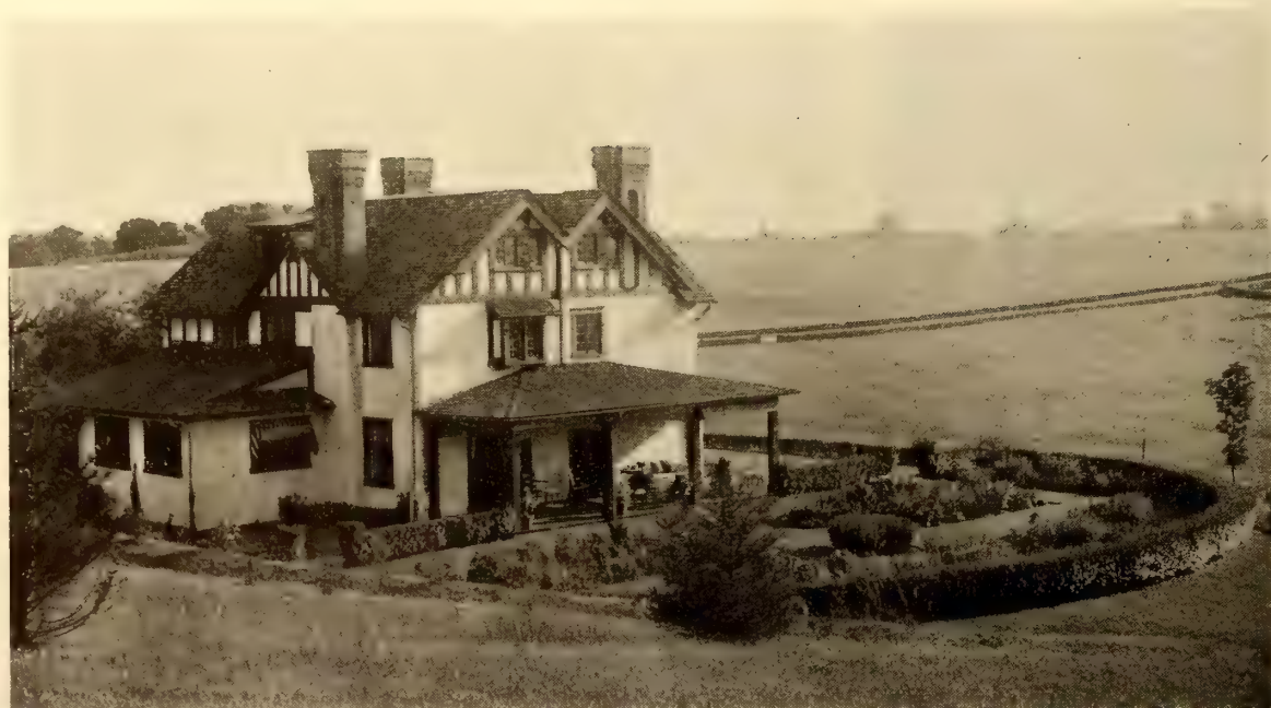
"Orchard Lea" Is a Stucco House with Half-timber Gables
