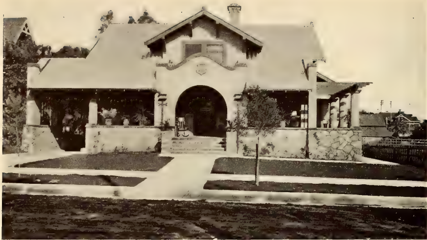
A Pleasing Combination of Cement, Crimson Roof Tiles and Cobblestones Cost $5,500
