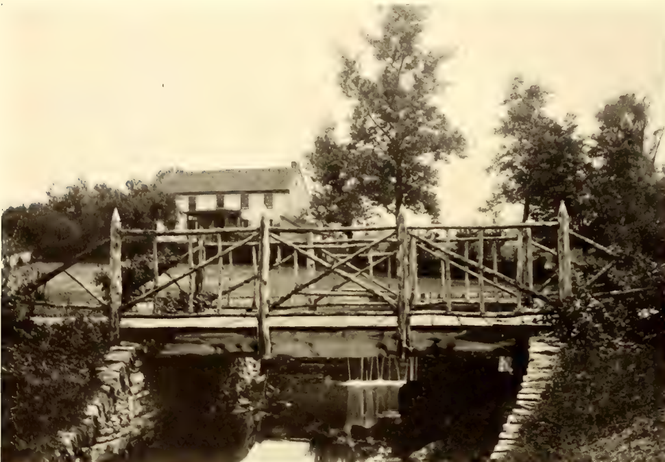
A Rustic Bridge of Simple Design
