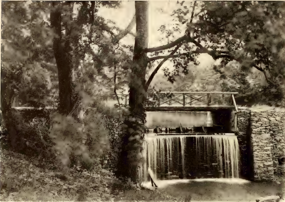
Bridge Above a Dam
