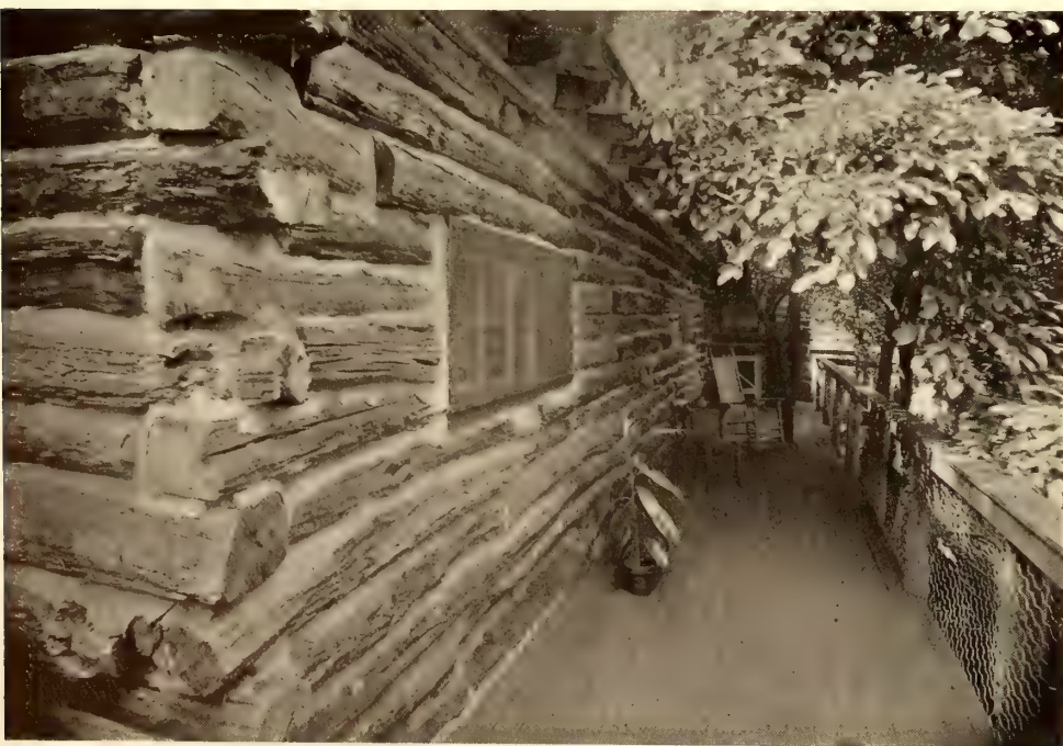
The Porch Above the Creek
