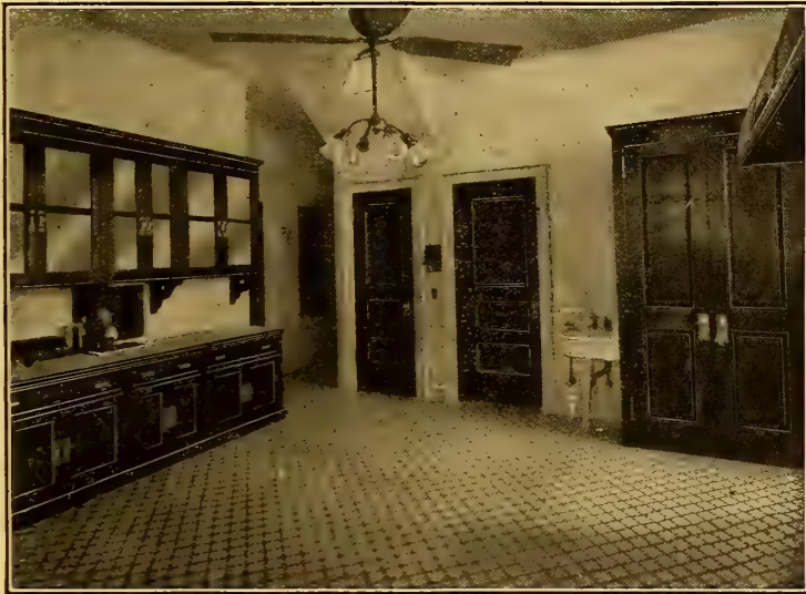
Kitchen Showing Interlocking Rubber Tiling in Residence of Mr. Webb Horton, Middleton, N. Y.
