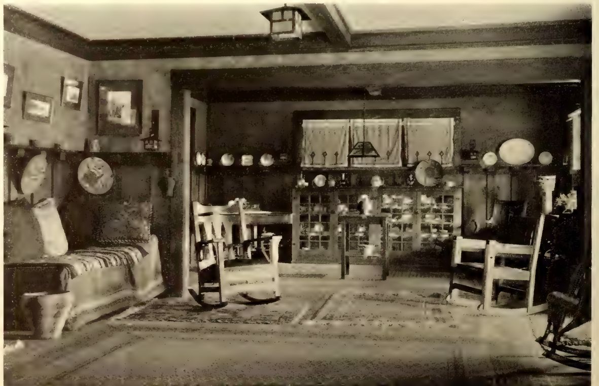
Looking from the Living-room Into the Dining-room. Showing Paneling, Block Supports for Plate Rail, and China Cabinet
