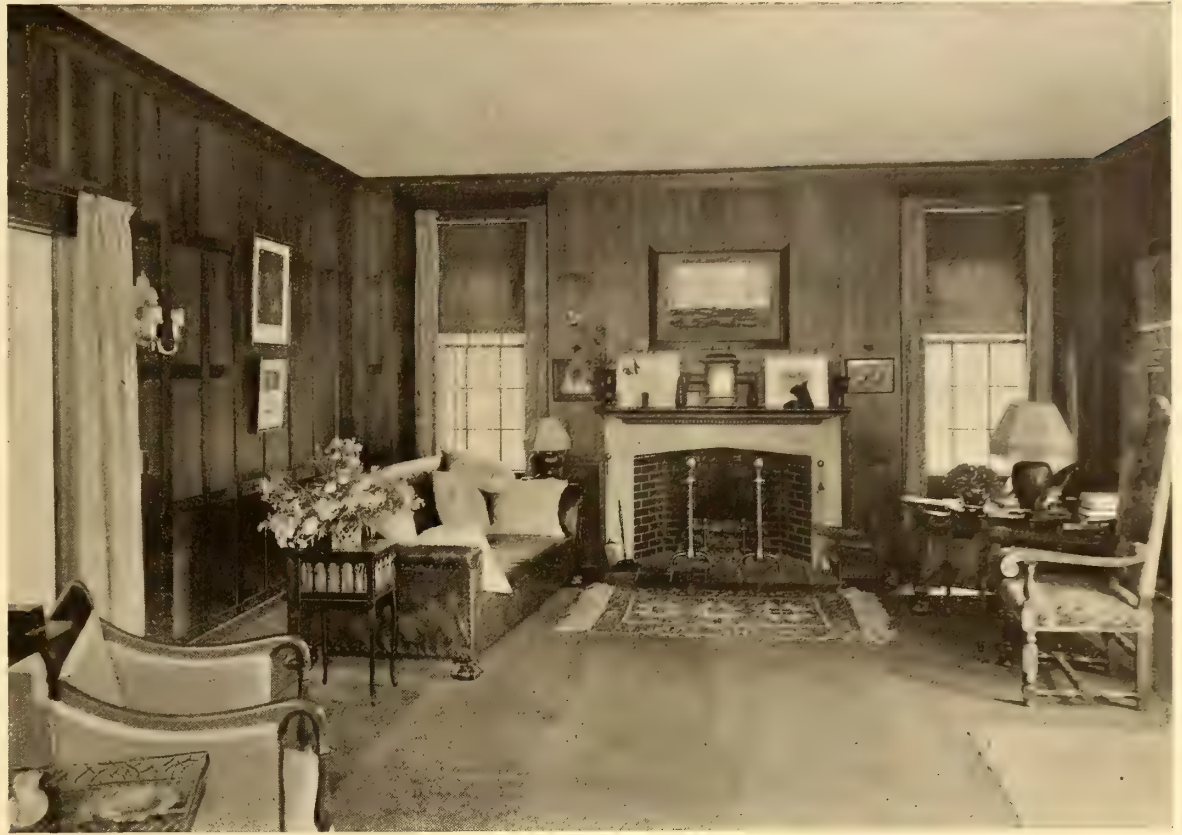
The Library Fireplace Is Built of Caen Stone
