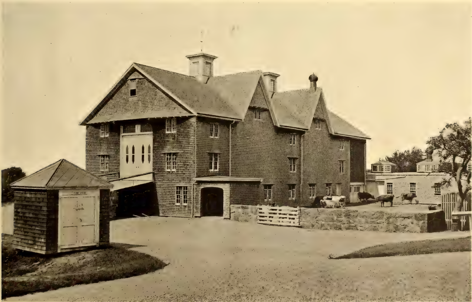
The "Bank," Is Three Stories in Height, Affording Accommodation for Cattle and Storage for Hay
