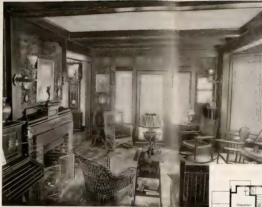
The Walls Are Paneled with Cypress Battens, with the Space Between Covered with Tapestry
