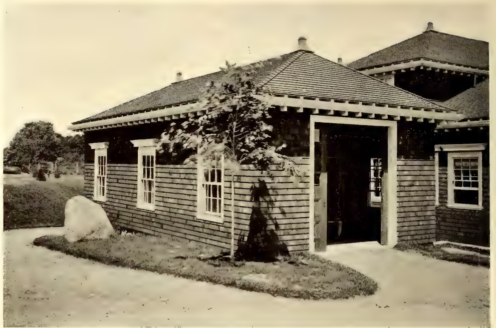
Garage Design in Harmony with the House
