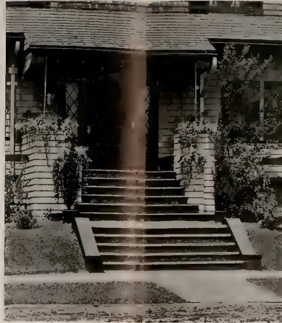
Flower boxes built in the buttresses are the feature of the entrance porch
