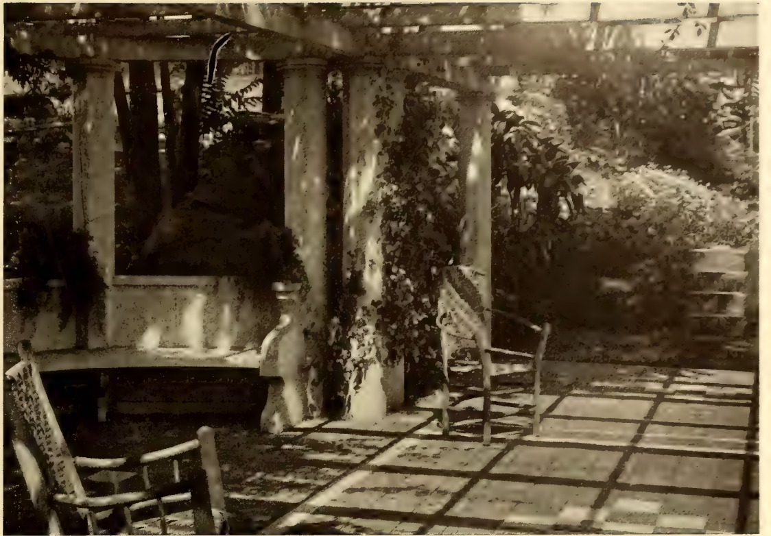
The Seat of the Pergola Wall
