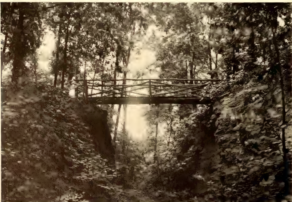
A High Bridge Across a Stream
