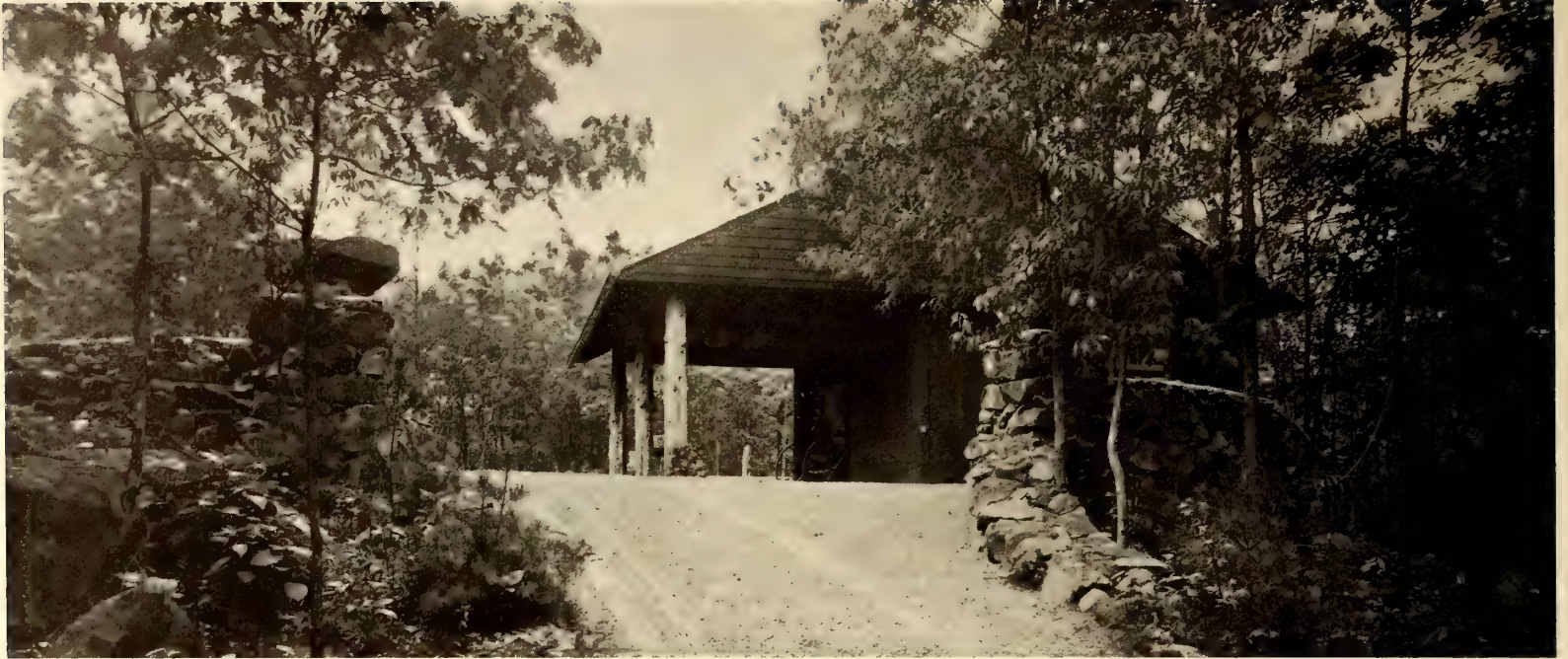
Fieldstone Wall and Gate Posts Are Built at the Entrance to the Property
