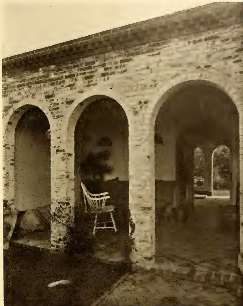
The Cloisters are Happy Characteristics of this Interesting House
