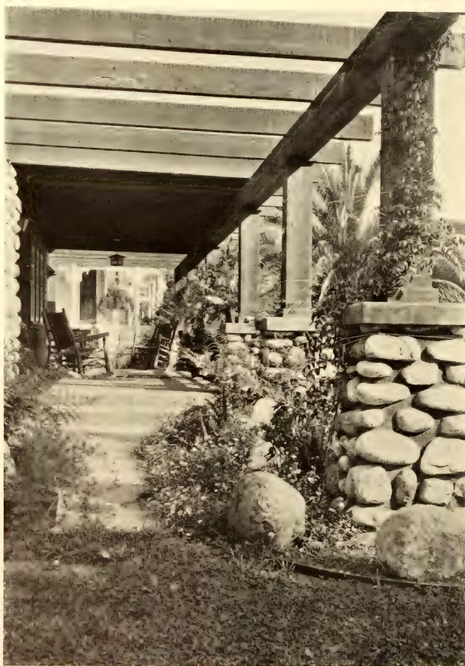
The Spacious Veranda Has Cemented Floor and Steps, and Roof of Heavy Rough Timbers, Supported by Posts on Cobblestone Foundations
