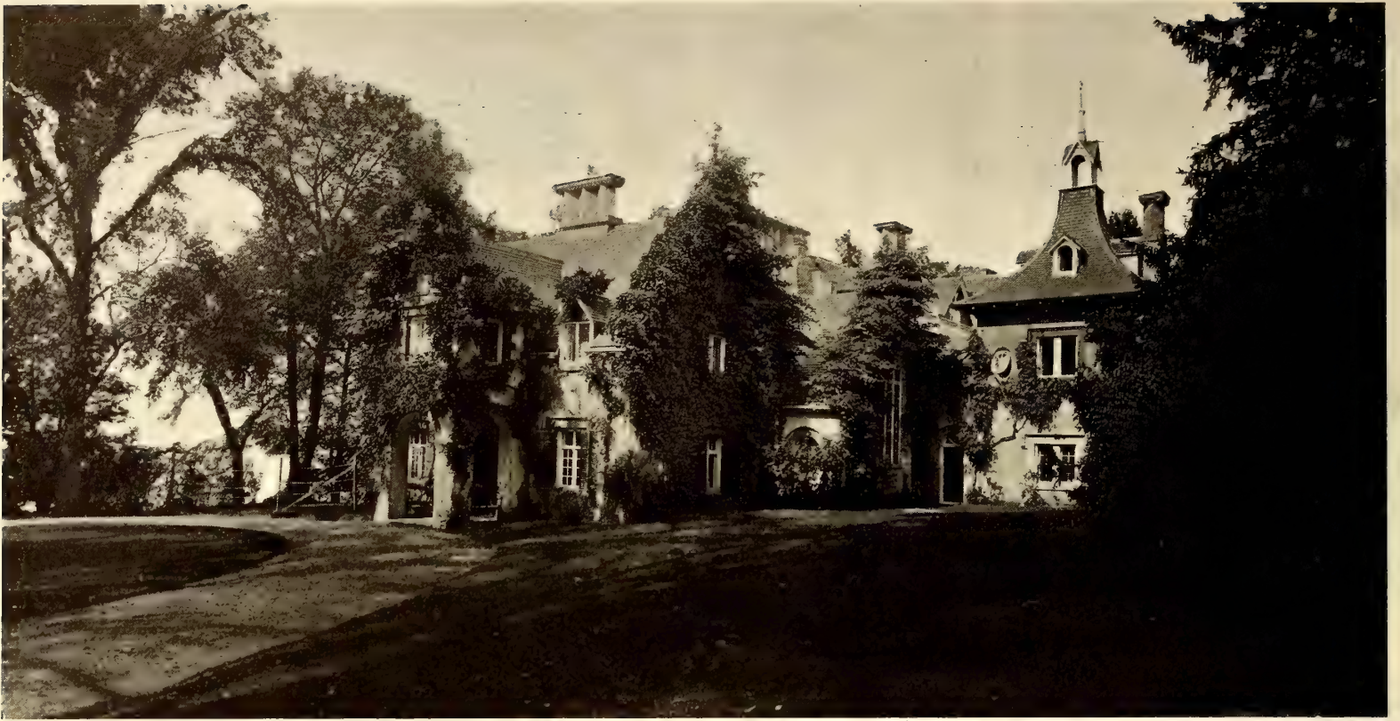
The Structure Is of Stucco with Roof of Bright Red Tiles, as It Appears After the Alterations
