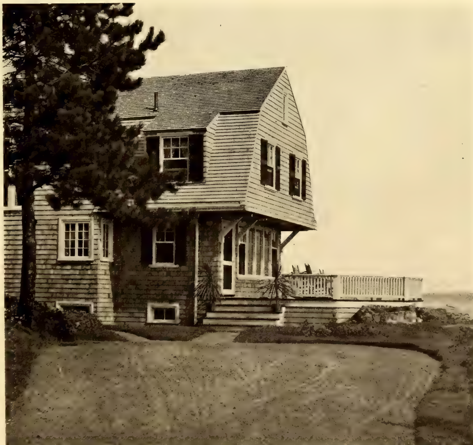
Gable End and Terrace
