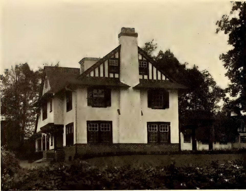
The Houses Are Built of Stucco with a White Cement Wash and Red Brick Base
