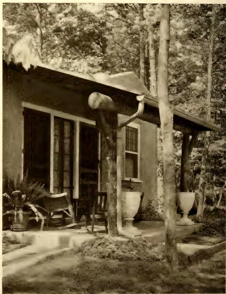
A Rustic Porch Is Built at the Front of the Bungalow
