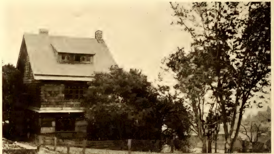
Double Rows of Shingles Are Used for the First Story of the House; Regular Shingled Sides Complete the Second Story
