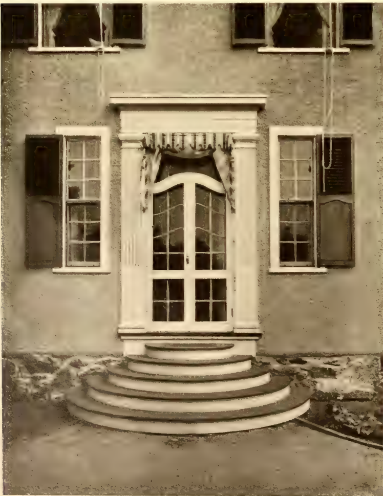
The Side Portal Stands atop a Semicircular Pyramid of Steps Leading to the Garden
