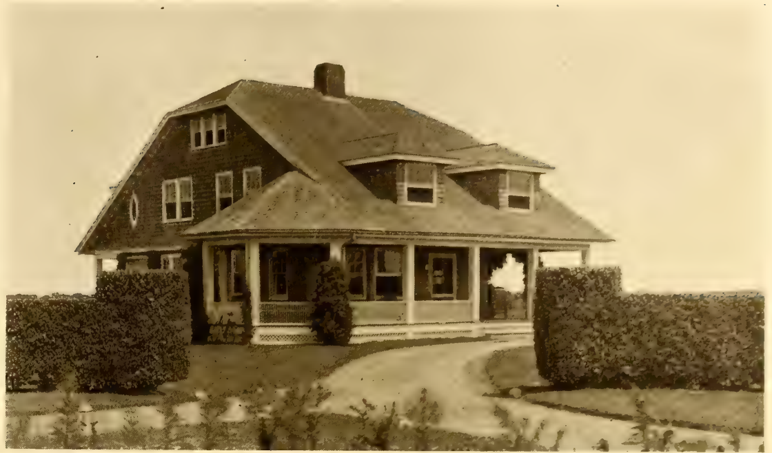
The house is covered with shingles, finished with weathered stain, and the trim in painted white
