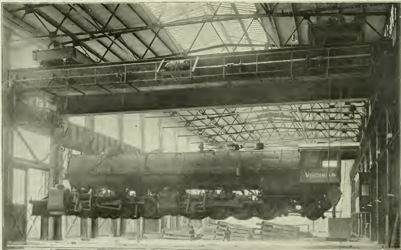
Mallet Locomotive Lifted by a 200-Ton Niles Crane; Virginian Railway.
