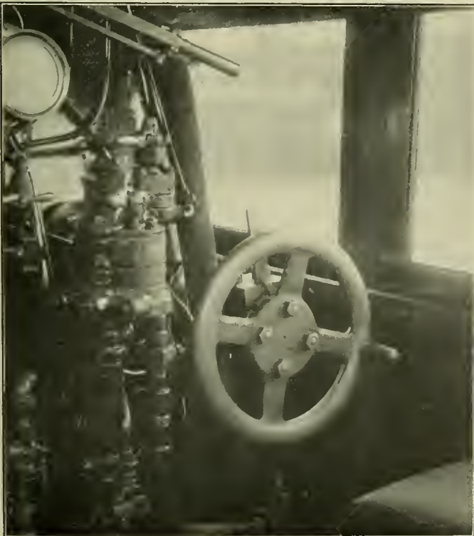
Operating Wheel for Screw Reverse Gear.
