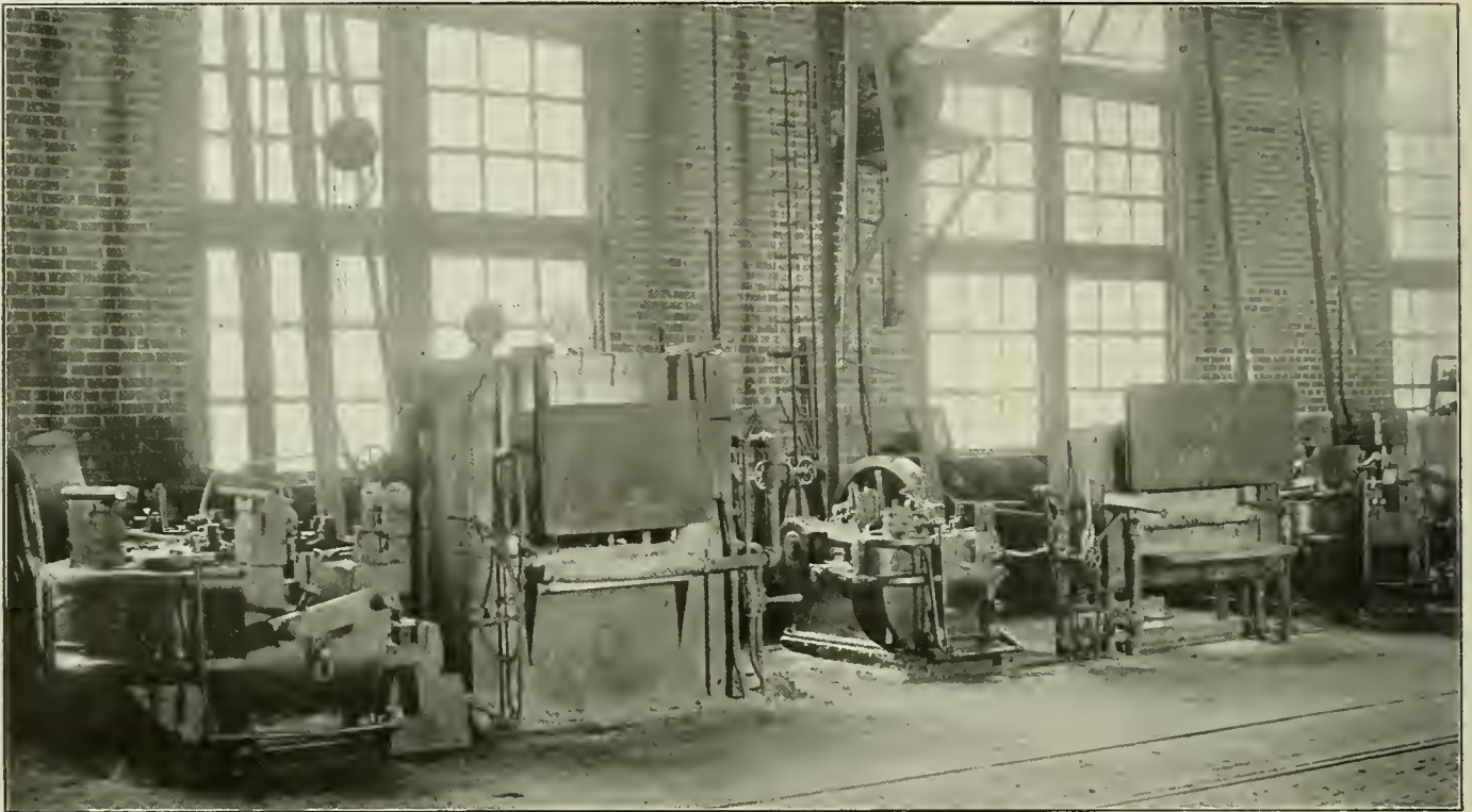
Gas Furnaces for the Forging Machines.
