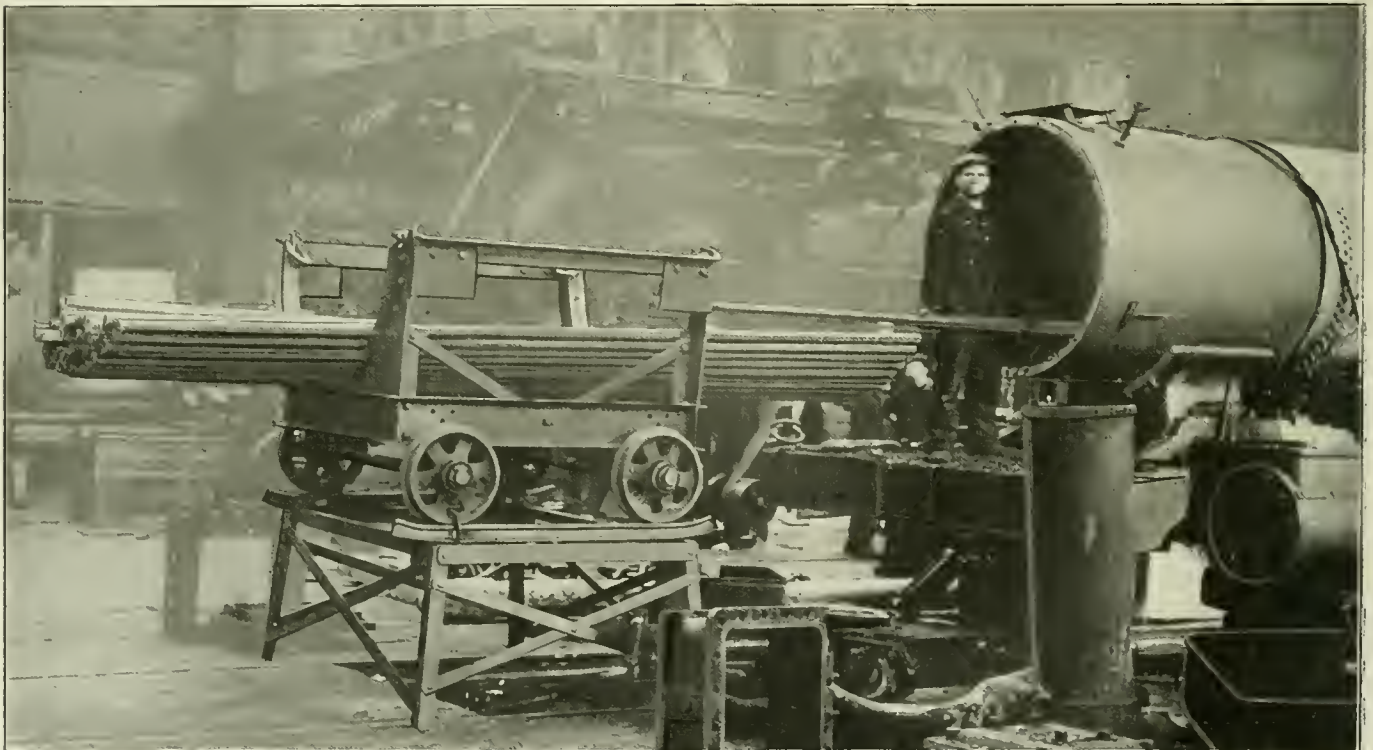
Fig. 2—Removing Tubes from the Boiler and Loading on the Flue Car in the Erecting Shop.
