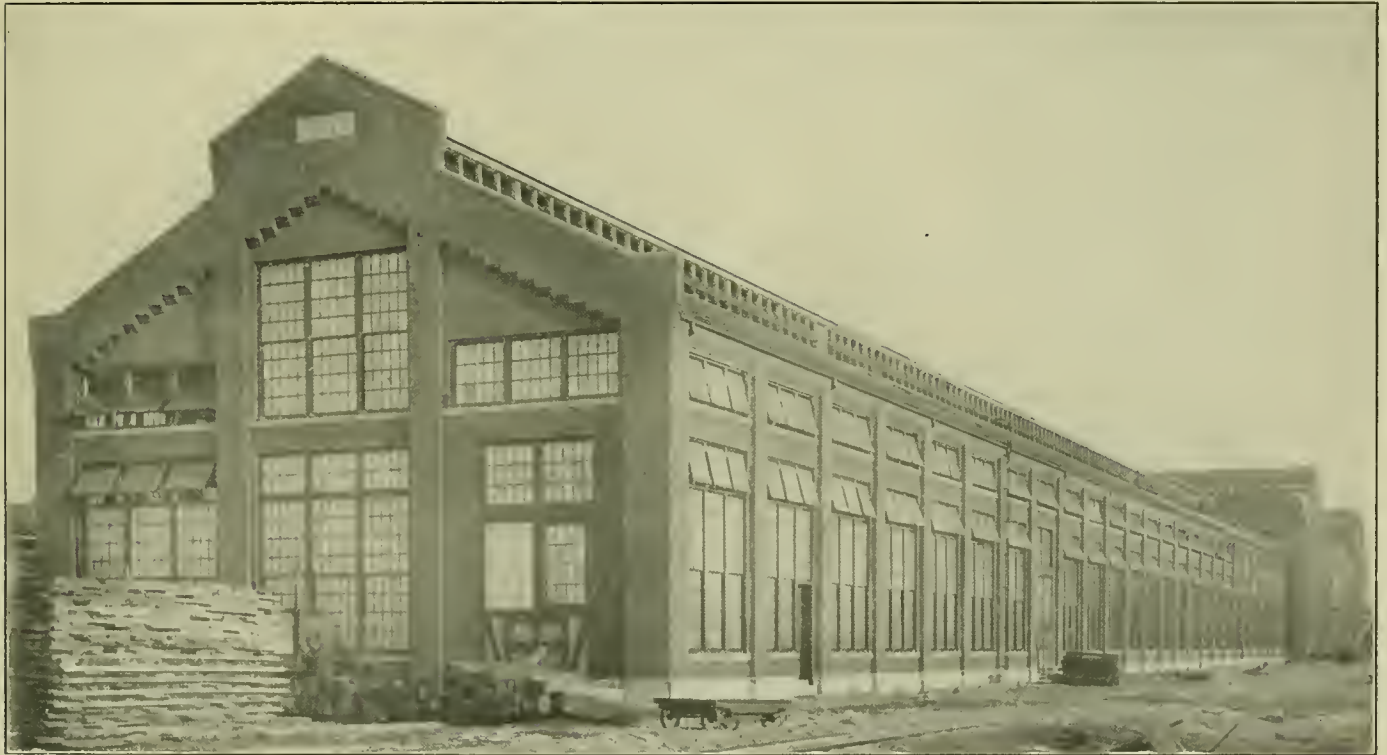
General View of Tank, Cab and Pilot Shop; Machine and Erecting Shop in the Background.
