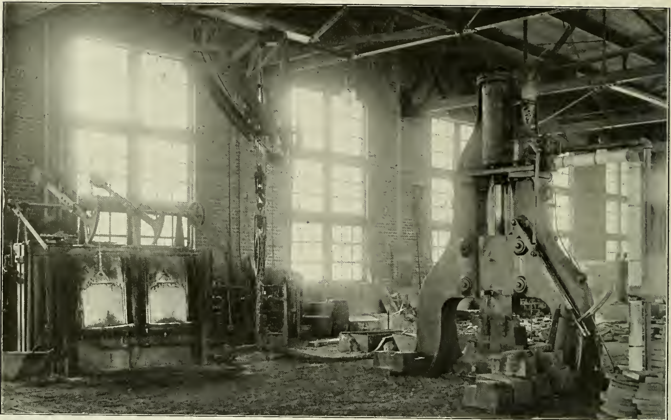
Gas Furnace for Steam Hammer Work.
