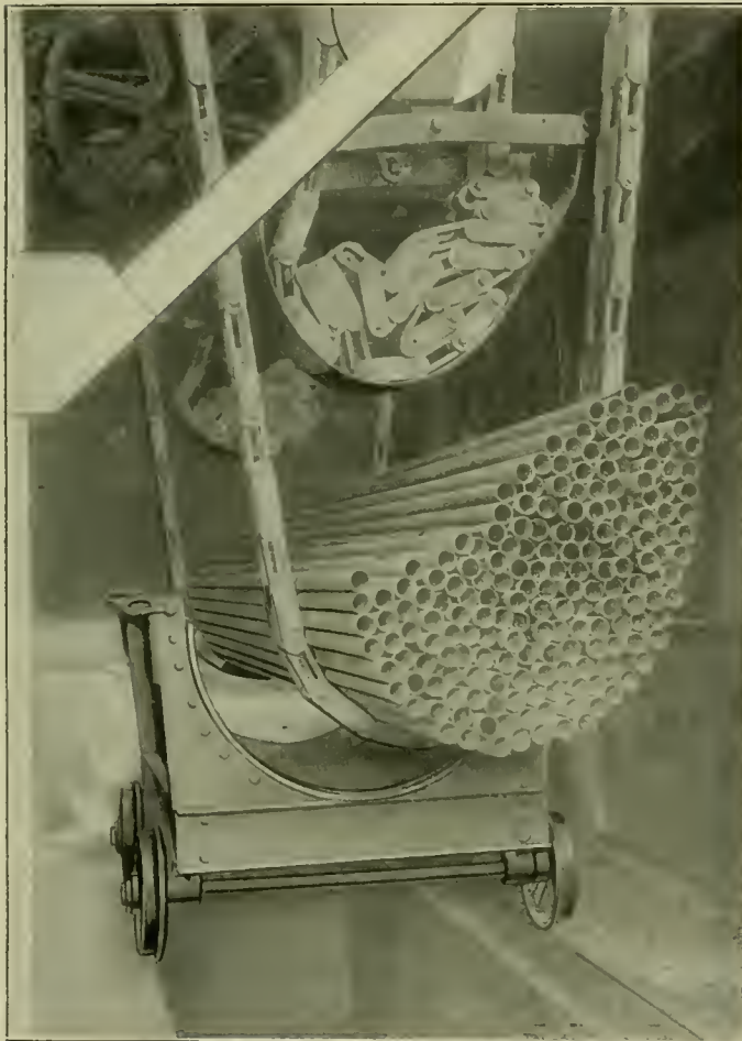
Fig. 4—Removing or Loading Flues at the Cleaner.
