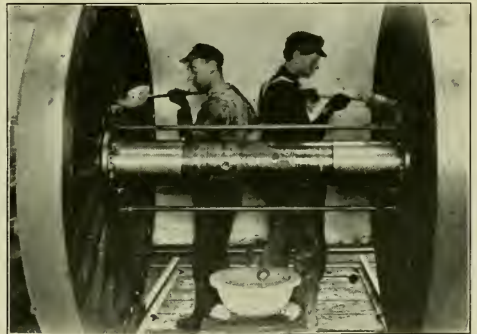
Fig. 11—Pouring Babbitt Hub Liners.
