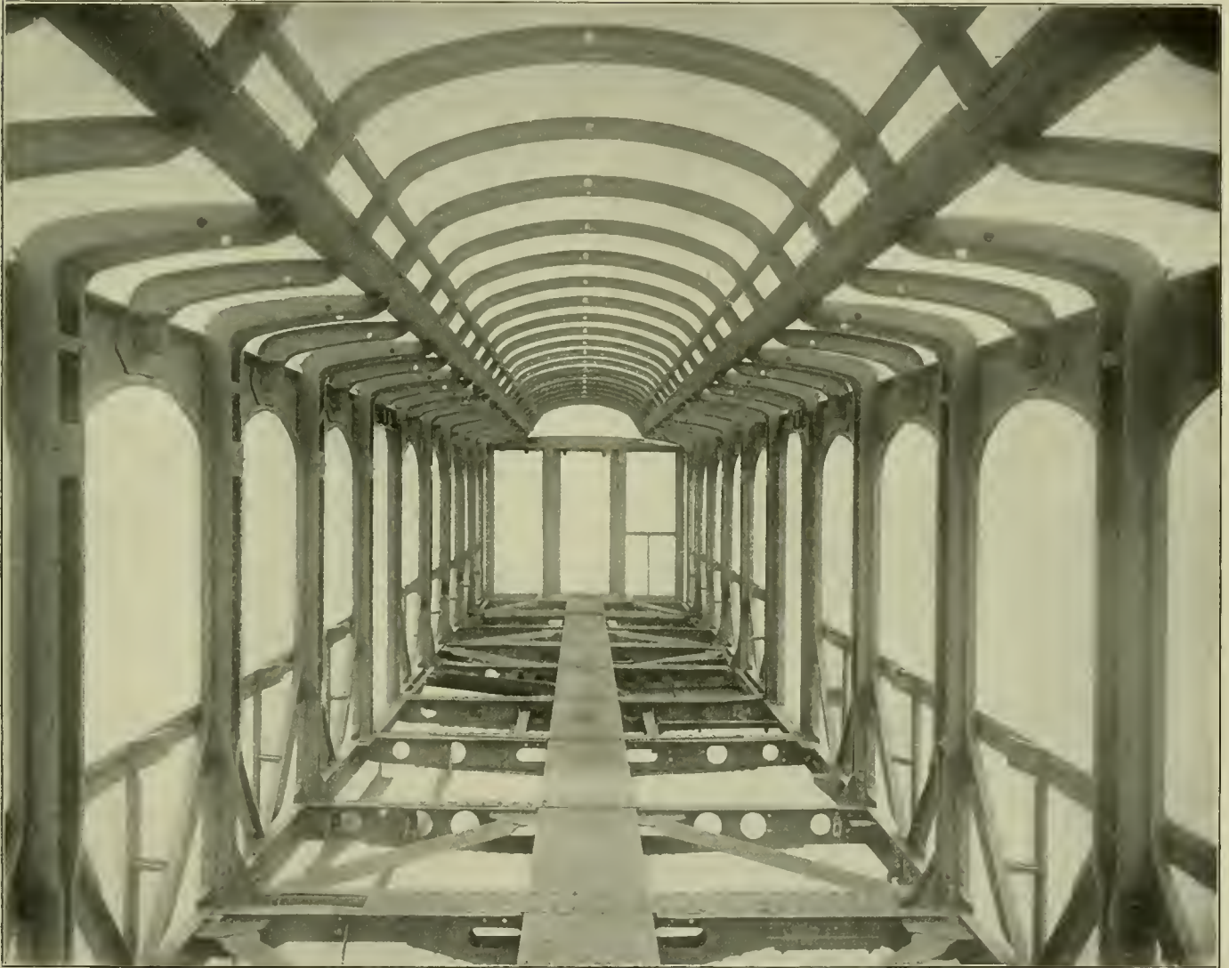
Showing the Extent to Which Pressed Steel Shapes are Used in the Framing of the All-Steel Suburban Cars.
