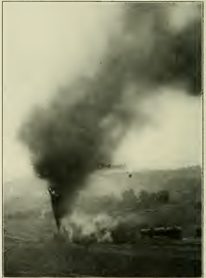
Radial Stay Boiler Just as the Crown Sheet Gave Away.
