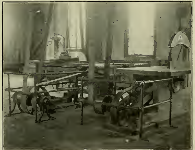
Fig. 7—Railing and Guards for Safeguarding Woodworking Machines.
