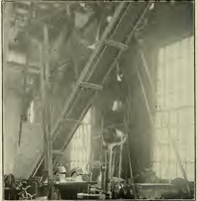
Fig. 3—Protecting the Workmen From the Breakage of a Main Belt.
