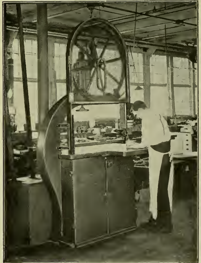
Safeguards on a Band Saw.
