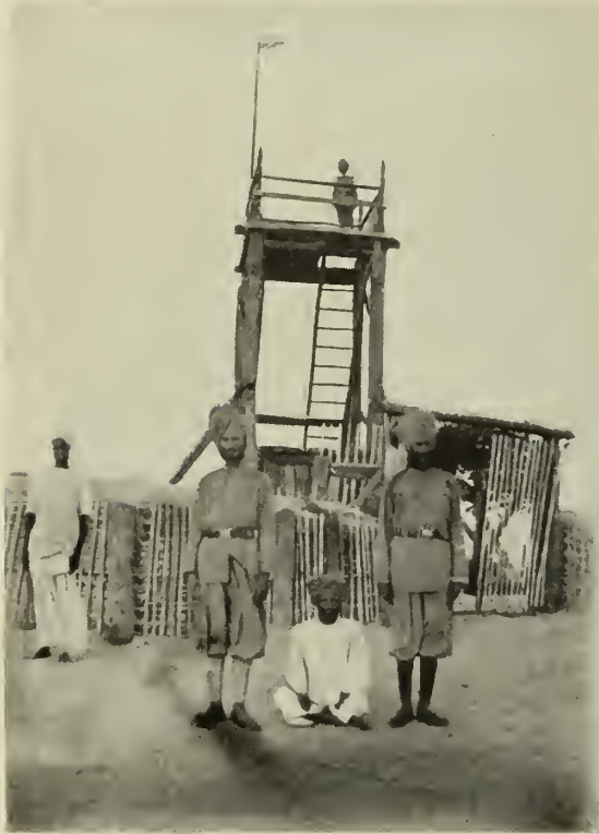
WATCH TOWER AT FORT JOHNSTON ERECTED BY CAPTAIN C. E. JOHNSON TO WATCH ZARAFI
