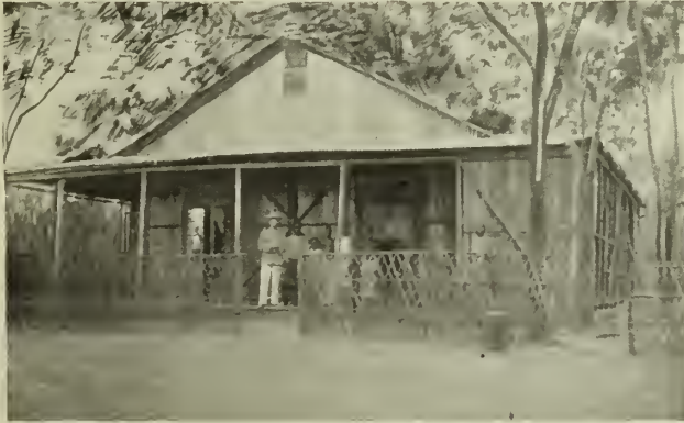
COLLECTOR'S HOUSE AT FORT LISTER
