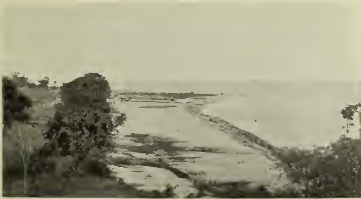
THE BEACH AT MAKANJIRA'S (PRESENT SITE OF FORT MAGUIRE)
