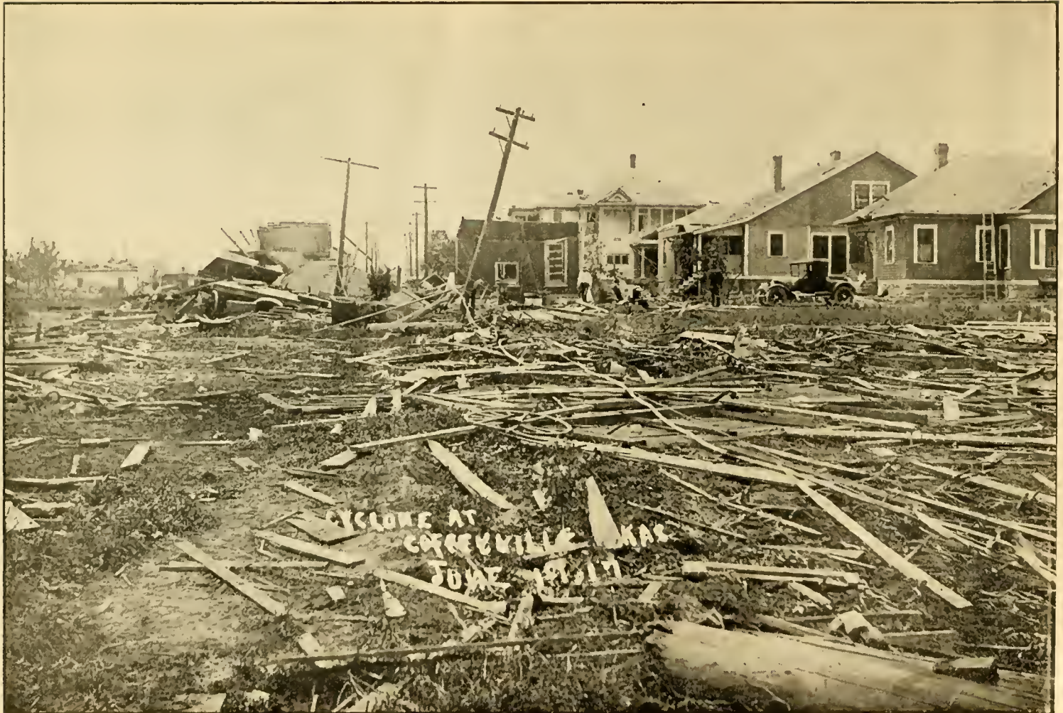
Path of Cyclone in 1300 Block looking north and west.
