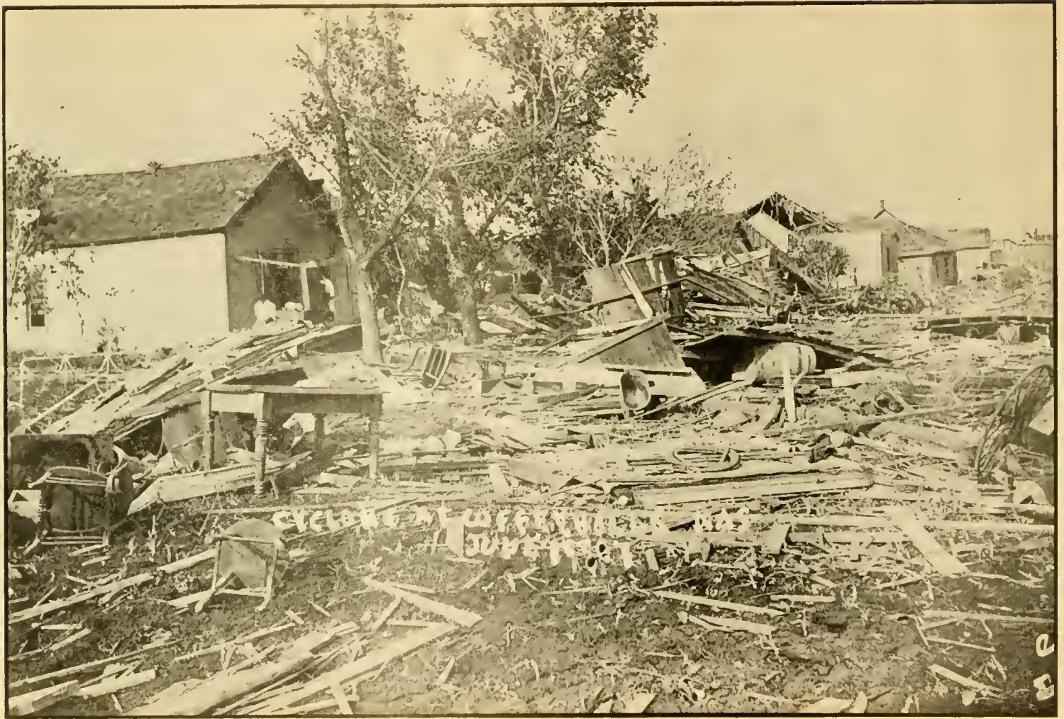
1200 Block at 1219 Walnut, looking east.
