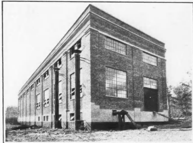
Completed building as viewed from the Northeast corner
