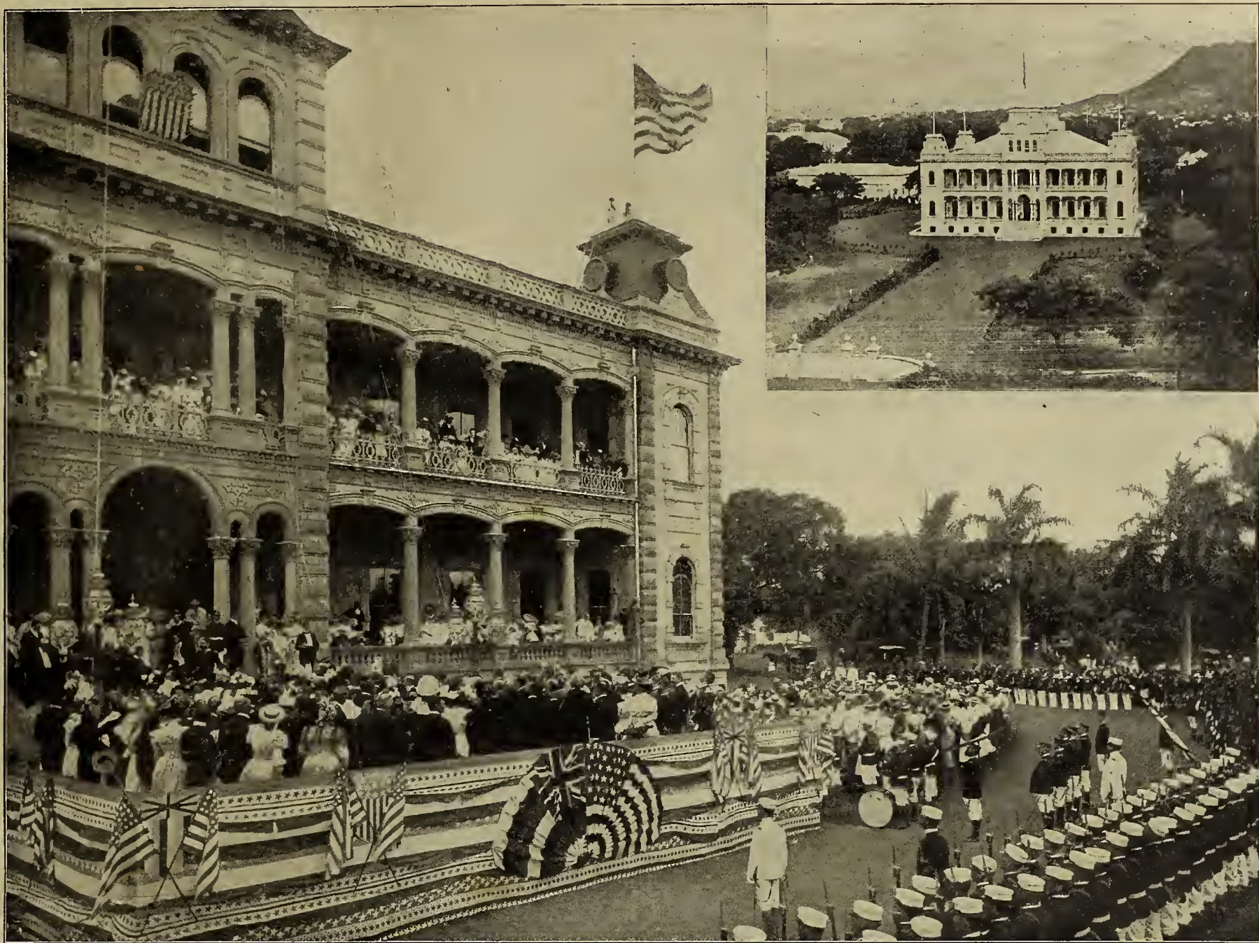
Raising the United States Flag Over the Hawaiian Capitol Building During Annexation Ceremonies, August 12, 1898—A View of the Building From a Distance
