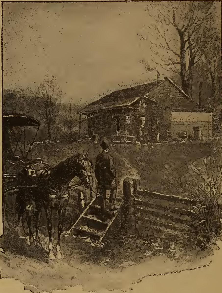
"THE HOUSE WAS A DILAPIDATED STRUCTURE OF LOGS"
