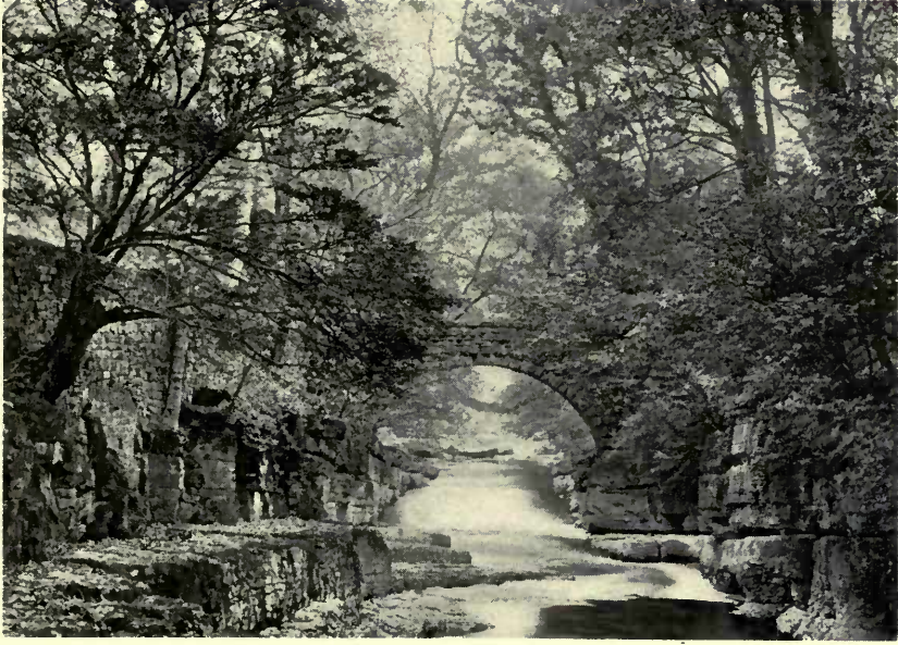
BRIDGE OVER THE GRETA.
