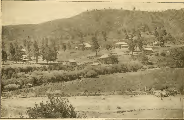
Augus on the Bonito River Near Intake of the Pipe Line Which Carries Water Thirty Miles to Carrizozo
