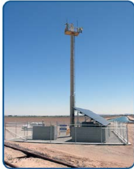
Figure 2. Remote Video Surveillance System 85
