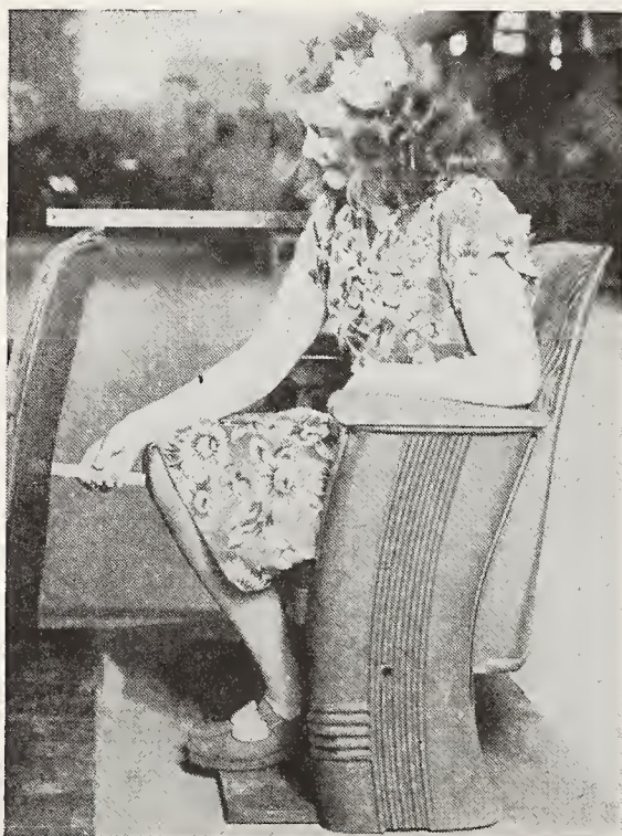
Indicating 6-inch space gained for passage by retraction of seat of the Air-O chair. The chairs used for these photographs were experimental models.
