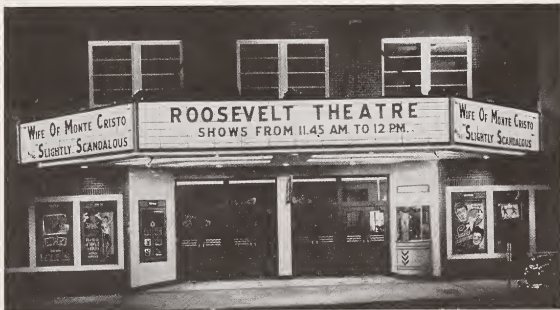
The change that modern attraction advertising equipment has brought in marquee display practices is well illustrated by this recent installation of Adler panels and letters. Relatively shallow, these panels are nevertheless used so as to get maximum display, using 10- and 16-inch letters with liberal lighted space. The theatre is the Roosevelt in Jacksonville, Fla., designed by Roy A. Benjamin.
