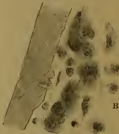
B—Part of clay walling, full of passages.
