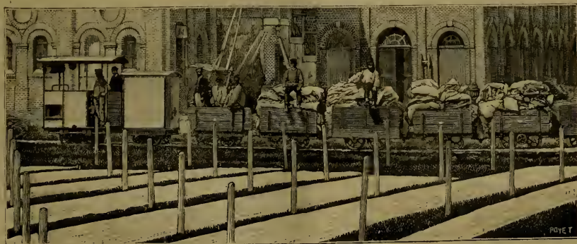
FIG. 4.—The return of the electric train from the bleaching ground.
