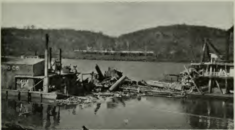
View of the wreckage following a boiler explosion in an Ohio river steamboat.
