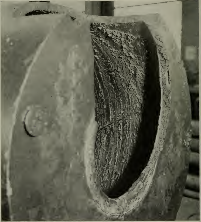
Figure 3—Lard cooler which exploded under normal use because of the failure of a defective casting.
