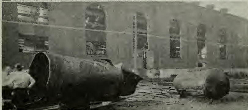
Results of a combustion explosion in an air line and two large air receivers.
