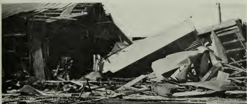
Figure 3—Wreckage following the explosion of a horizontal tubular boiler in New Mexico.
