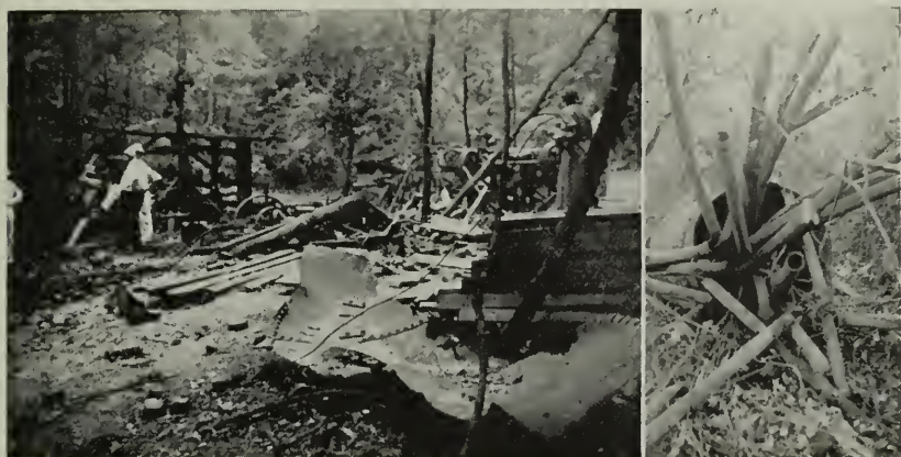
Figure 6—Left—Scene of an explosion in which two persons were killed and two injured. Right—Result of a lap seam crack. Three persons were injured by the explosion.
