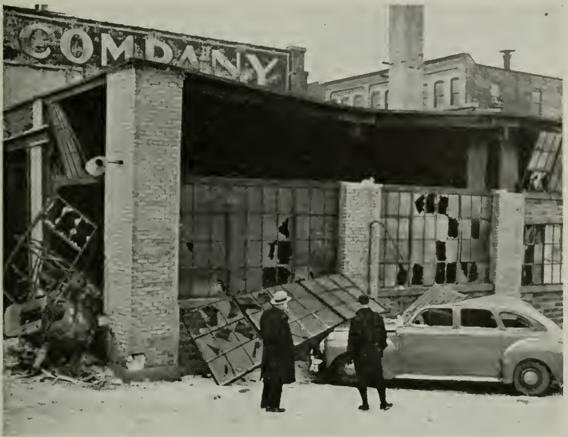
Figure 3—A check valve between a hot water heating boiler and its relief valve was reported as the cause of the explosion which wrecked this building.
