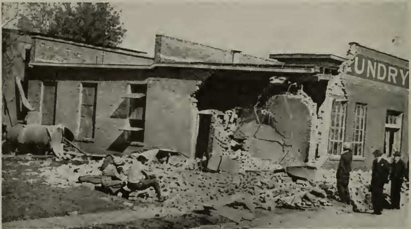
Figure 3—Damage following a boiler explosion at a laundry.
