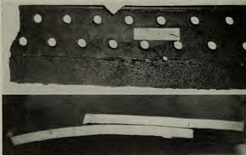
Figure 5—Top and end views of a typical lap seam crack. Notice that this defect is on the opposite side of the seam from the failures shown in Figures 1, 3, and 4. The picture at the upper right shows a lap seam failure under hydrostatic test.
