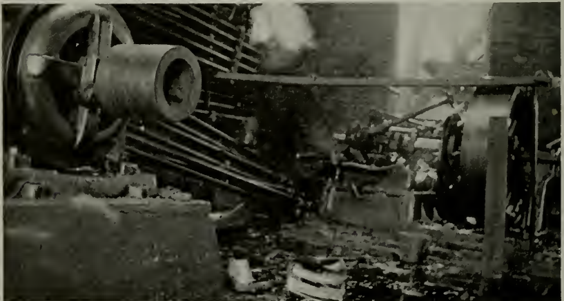
Figure 4—Only the bottom of the crankcase, the shaft and the wheel remained after this vertical twin-cylinder belt-driven ammonia compressor exploded. The cause was attributed to a combustion explosion in the crankcase. $7,500 was the estimated damage.
