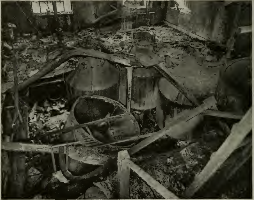
Scene in a soda recovery room at a paper pulp manufacturing plant after an explosion of a soda leaching tank.
