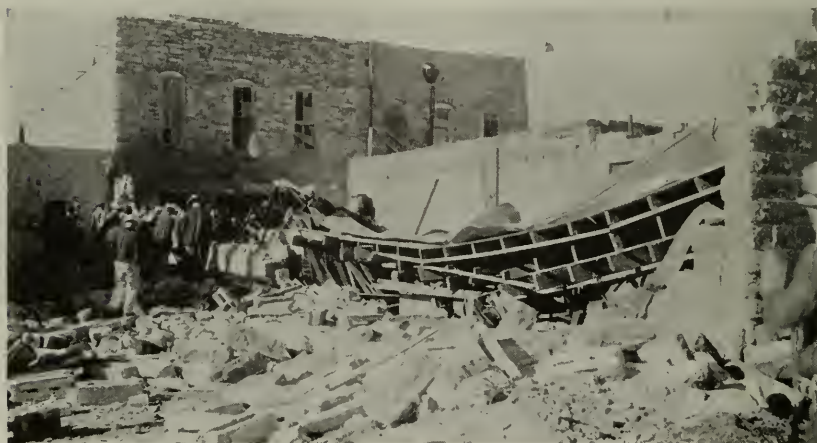
Figure 5—Wreckage after the failure of a welded patch on a Scotch-Marine type boiler.
