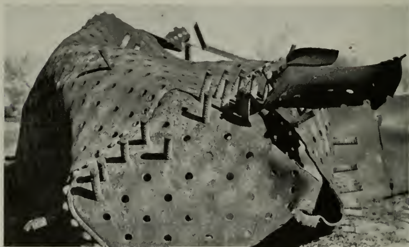
Figure 1—Firebox of a locomotive type boiler in an oil field after its explosion due to low water and over-heating.
