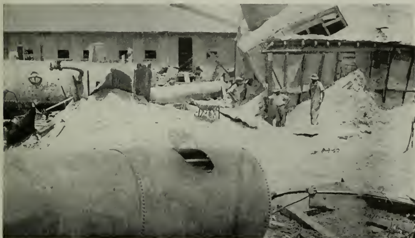
Figure 2. The shell, the hole where the patch shown in Figure 1 was attempted, and some of the debris which followed the explosion. Two other boilers were blown from their settings, the failing boiler rocketed 75 ft, the boiler house was wrecked, and one man was killed. It was reported that the boilers were not insured.
