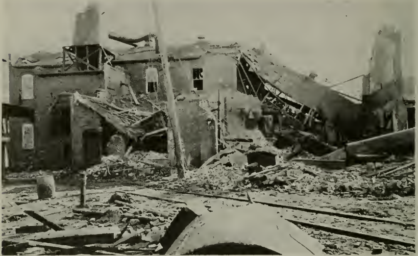
Figure 2—View of a North Carolina manufacturing plant wrecked by an explosion of a horizontal tubular boiler. Overheating from an accumulation of scale and sediment caused the accident.
