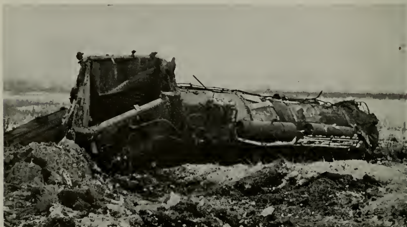
Figure 3—Weighing more than 40 tons, this track locomotive boiler was hurled 500' when low water caused failure of the crown sheet.
