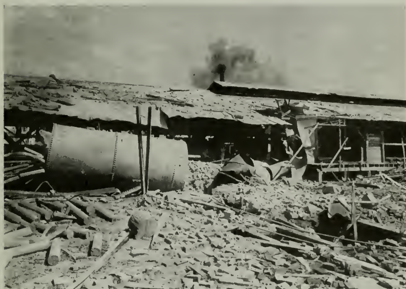
Figure 3—Georgia sawmill extensively damaged by an explosion of a horizontal tubular boiler. The feedwater contained tannic acid which resulted in rapid internal corrosion.
