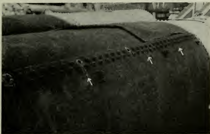
Figure 4—Failure in Boiler No. 3 after the hydrostatic test. The break at the right is clearly from embrittlement. The continuation of the failure across the boiler is a stress tear similar to that in Boiler No. 2, which exploded under steam pressure. The lap seam crack slots are indicated by the arrows.
