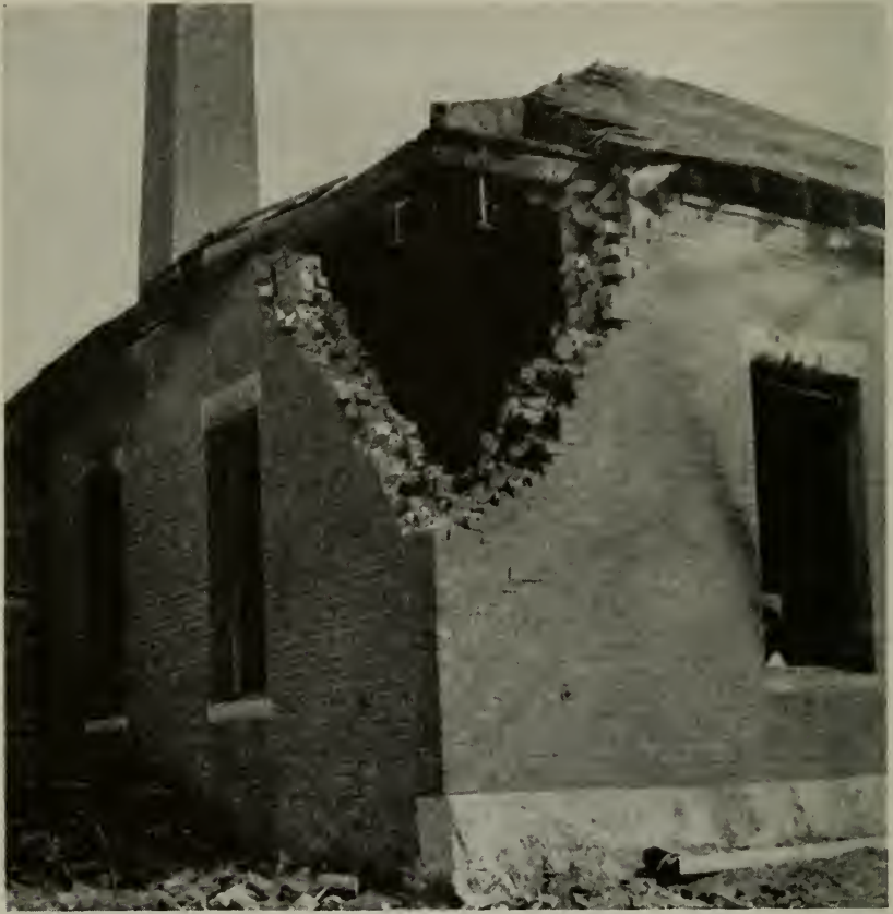
Figure 4—Where an air tank head passed after an explosion. The photograph gives an idea of the force of compressed air suddenly released.
