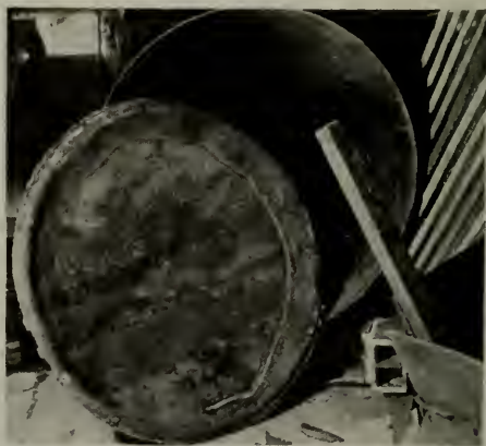
Figure 4. Head of a pneumatic tank which blew out when seal welding failed. Passing through a tile wall, the head damaged supplies in an adjacent room. The shell skidded in the opposite direction, breaking piping and sewer connections. Above the tank, floors and plaster were damaged. Insurance was not carried on the tank.
