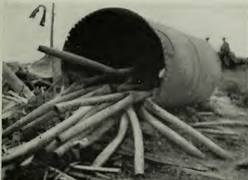
Figure 2—Two courses of a three-course horizontal tubular boiler which exploded because of corrosion.
