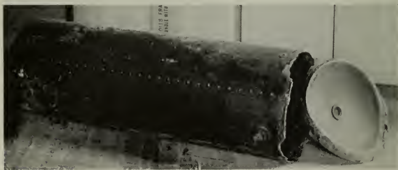
Figure 2—Reversed minus head An improperly adjusted safety valve permitted the building up of excessive pressure.
