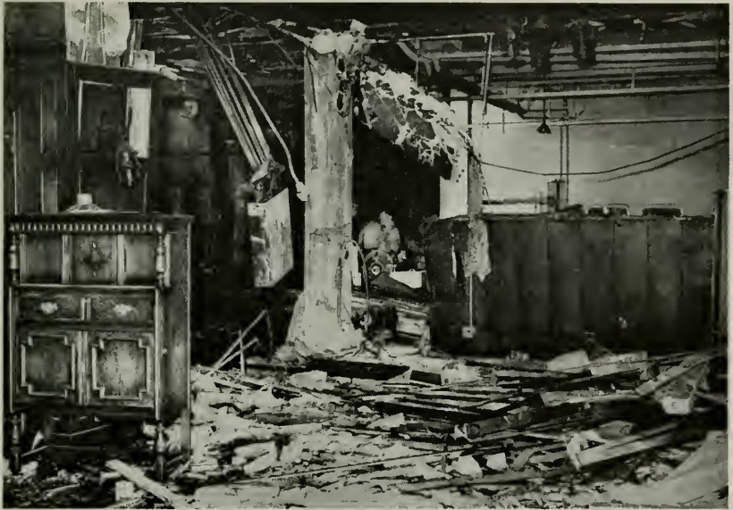
These ruins in a hotel grill-room resulted from an explosion of gas which had been generated in an oil-insulated transformer.
