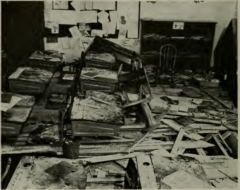
Figure 1—School room after air lift water system tank exploded.
