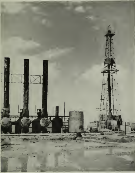
Derrick for the world's deepest well and three of the four boilers and the superheater which supplied steam for the drilling engine. The well, 15,004' deep, surpassed the former world's record by 2,218 feet.
