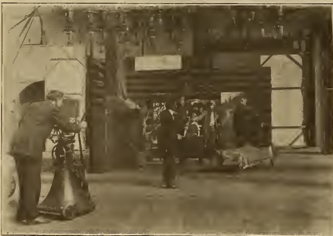
Producing an Interior, Edison Studio.
