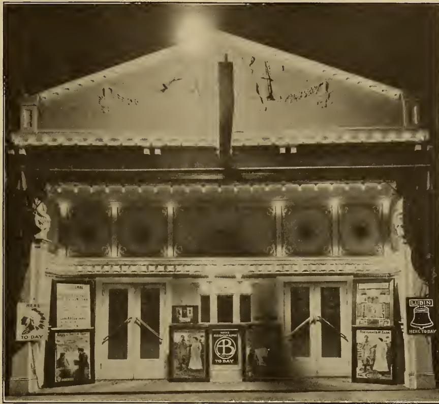
Grand Theater at The Dalles, Oregon. Two Hundred and Fifty Incandescent Lamps Blaze a Welcome.
