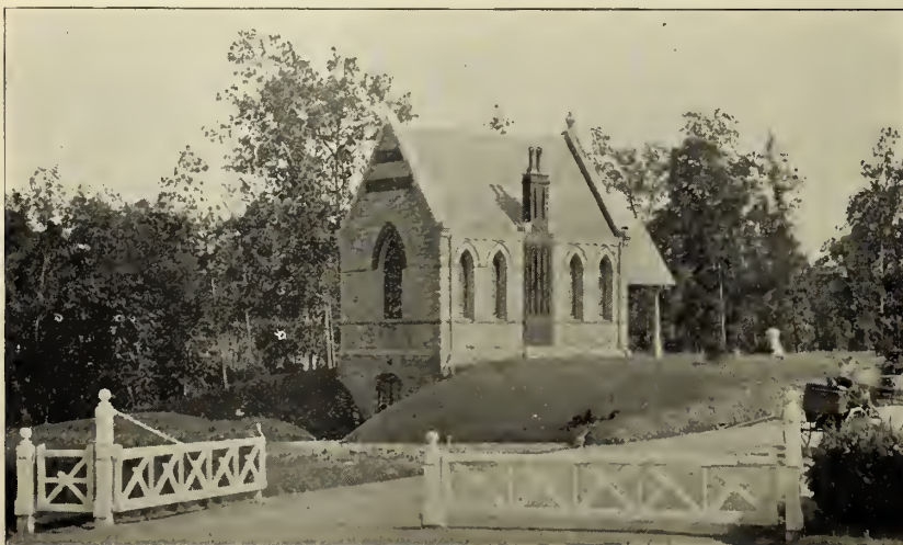
CHAPEL AND RECEIVING VAULT, RIVERSIDE CEMETERY, DEFIANCE, O.
