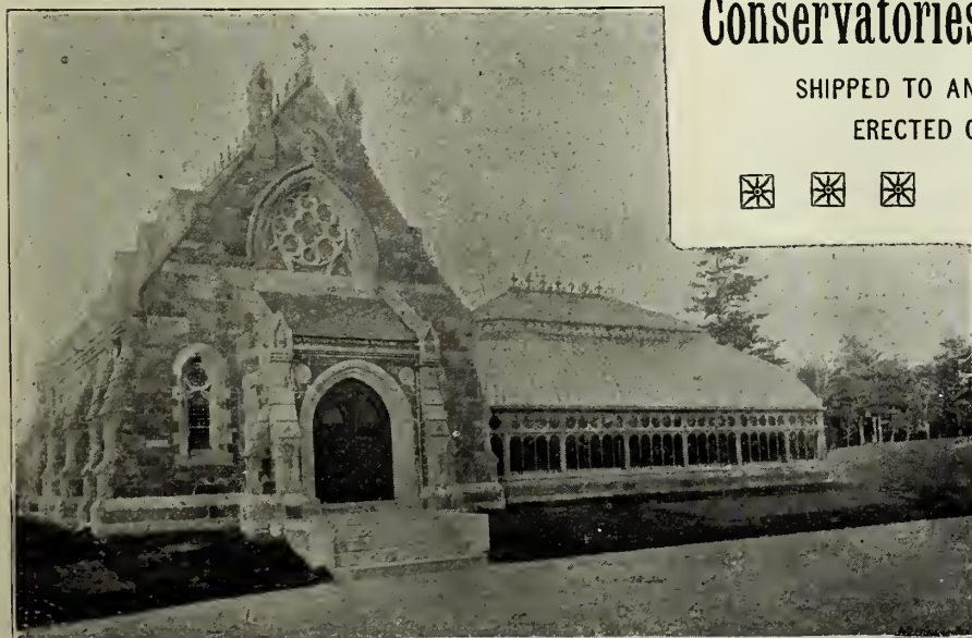
Conservatory in Newton Cemetery, Newtonville, Mass., designed and erected by Lord & Burnham Co
