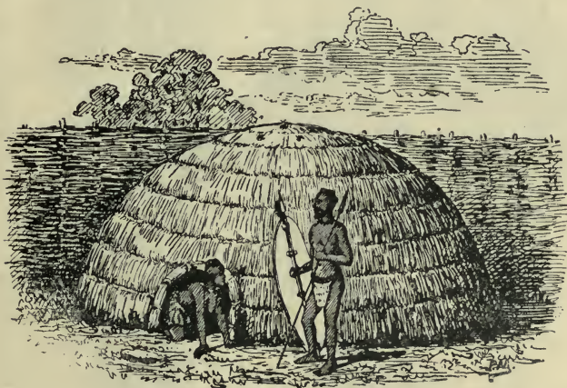
FIG. 41.—Hemispherical hut in straw of Zulu Kafirs. ( After Wood and other sources. )
