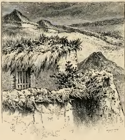
ENTRANCE TO THE HACIENDA, PEDREGAL.
