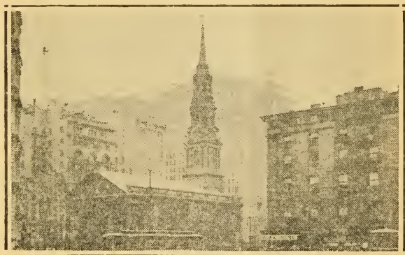
St. Paul's Church, Astor House, and Hudson Terminal Buildings, 1912.
