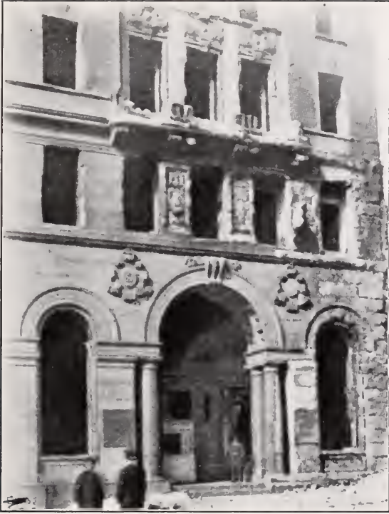
Sandstone front of the Maryland Trust Building at Baltimore Md., damaged by the fire. 1904
