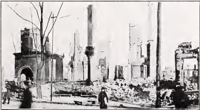
Fig. 2 Ruins of the Danforth City Library at Paterson N. J. 1902
