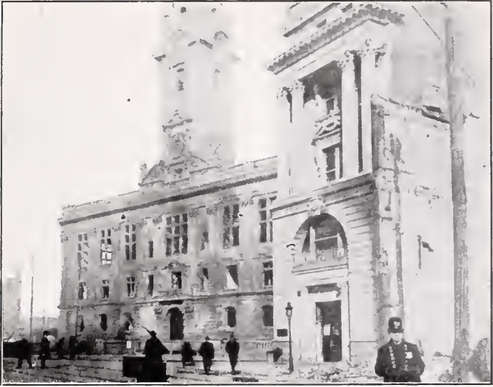
Fig. 1 Showing damage to granite in the City Hall at Paterson N. J. 1902
