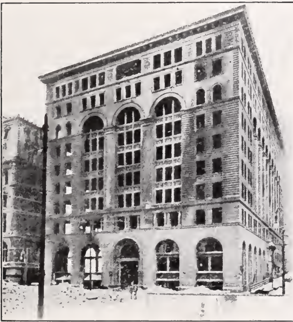
Equitable Building, Baltimore Md. The granite in this building was little damaged by the fire. 1904
