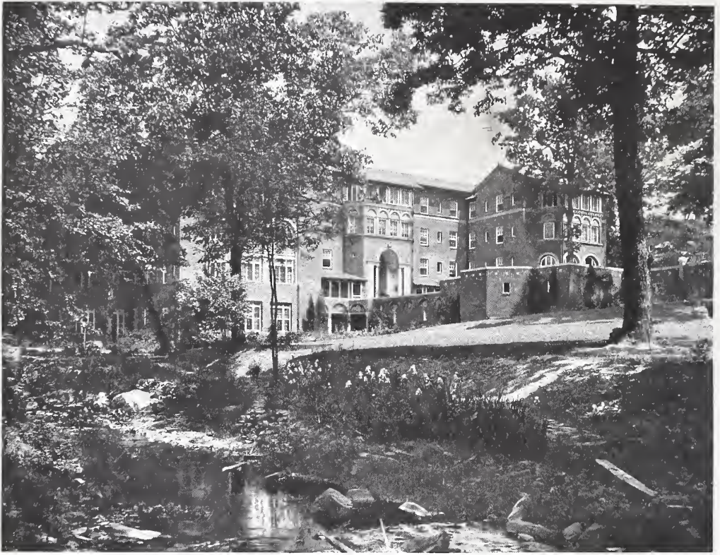
FIG. 66. TUSCANY APARTMENT HOUSE, BALTIMORE, MD. Clyde N. Friz, Architect.
