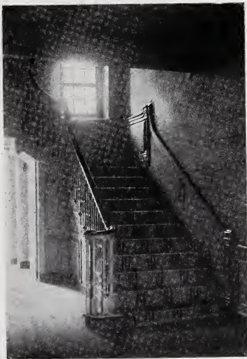
STAIRWAY IN KEEPER'S HOUSE, CHARMING FORGE.
