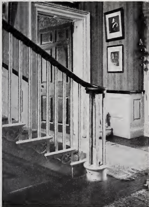
DETAIL OF STAIR BALUSTRADE, UPSALA, GERMANTOWN (1798)
