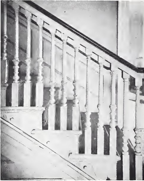
DETAIL OF STAIR BALUSTRADE, CLIVEDEN, GERMANTOWN (1763).
