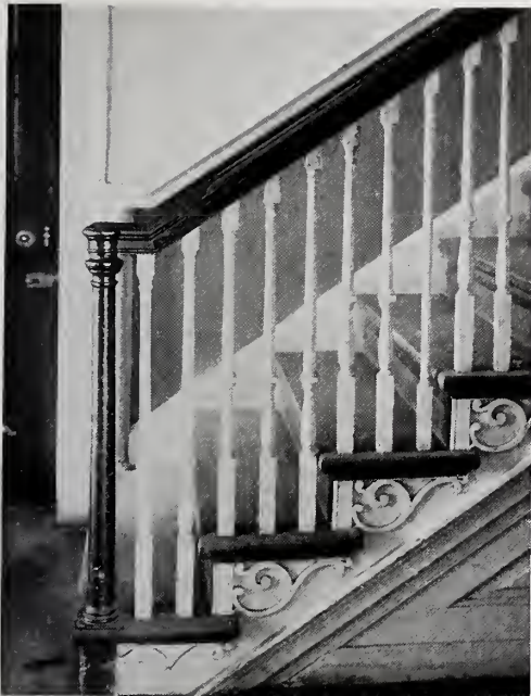
DETAIL OF STAIR BALUSTRADE, GOWEN HOUSE, MOUNT AIRY.
