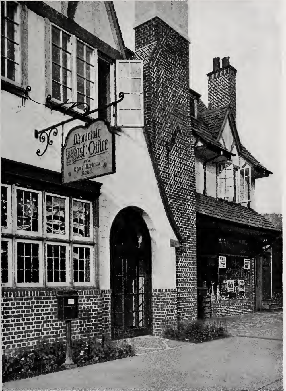
DETAIL OF POST OFFICE, UPPER MONTCLAIR, N. J. FRANCIS A. NELSON, ARCHITECT.
