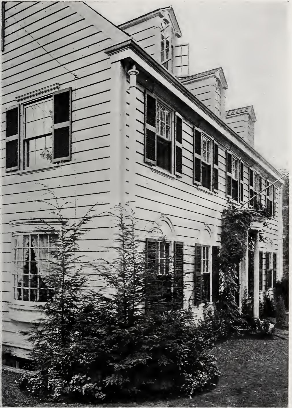
EAST END—RESIDENCE OF MISS E. S. CUSHING, WABAN, MASS. GRAND- GENT & ELWELL, ARCHITECTS.
