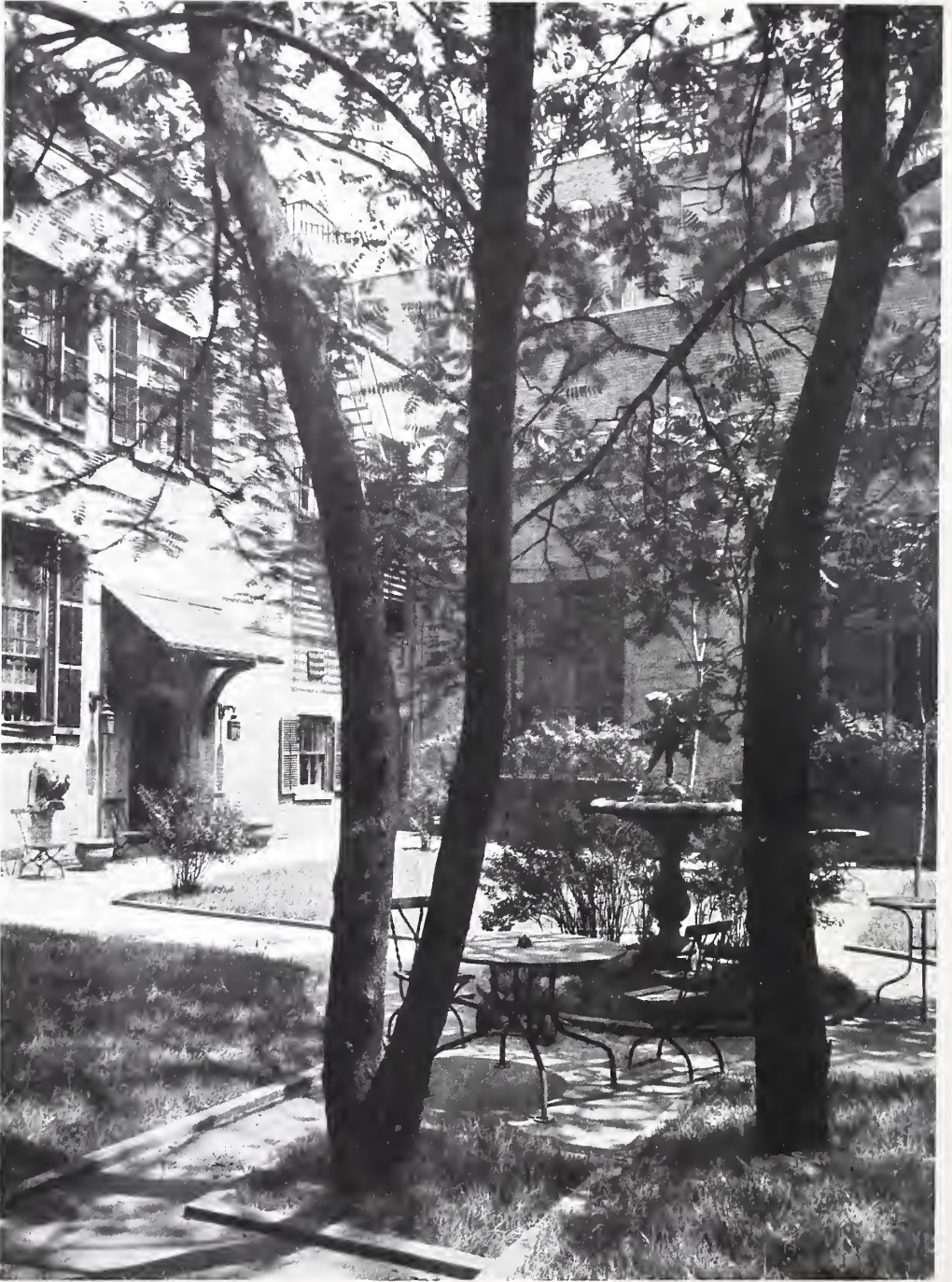
FIG. 11. ENTRANCE TO COURTYARD — "WESTOVER COURT," 206-214 WEST 44TH STREET AND 207-215 WEST 43RD STREET, NEW YORK. EVARTS TRACY, ARCHITECT.
