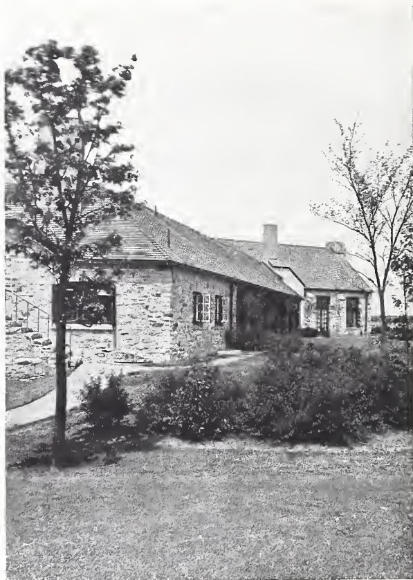
ENTRANCE TO MEN'S LOCKER ROOM, NORWOOD GOLF CLUB, LONG BRANCH, N. J. Harry Allan Jacobs, Architect.
