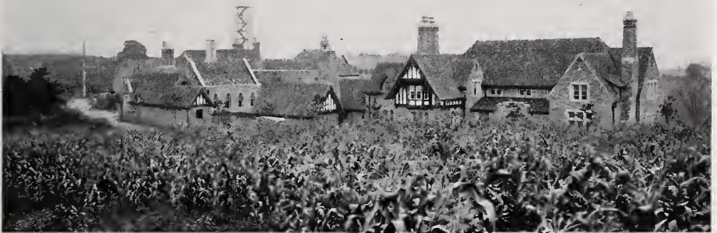
THE STEEL TOWER, A TEMPORARY OBSERVATION PLATFORM, MARKS THE SITE OF THE FUTURE CARSON MEMORIAL TOWER.
