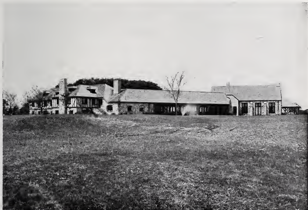
VIEW OVERLOOKING LINKS—NORWOOD GOLF CLUB, LONG BRANCH, N. J. Harry Allan Jacobs, Architect.
