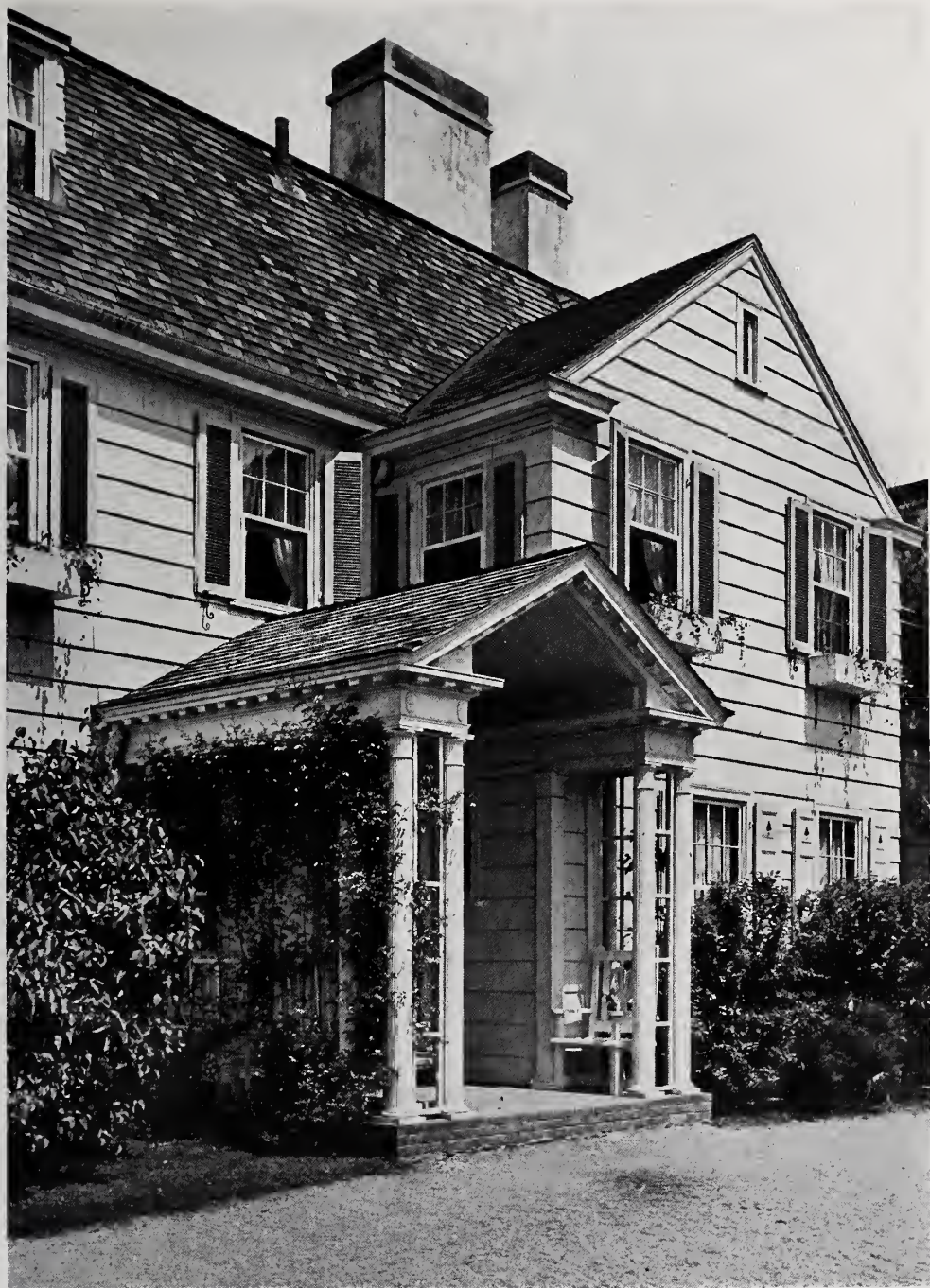
DETAIL OF HAAS HOUSE, MT. KISCO, N. Y. AYMAR EMBURY II, ARCHITECT.
