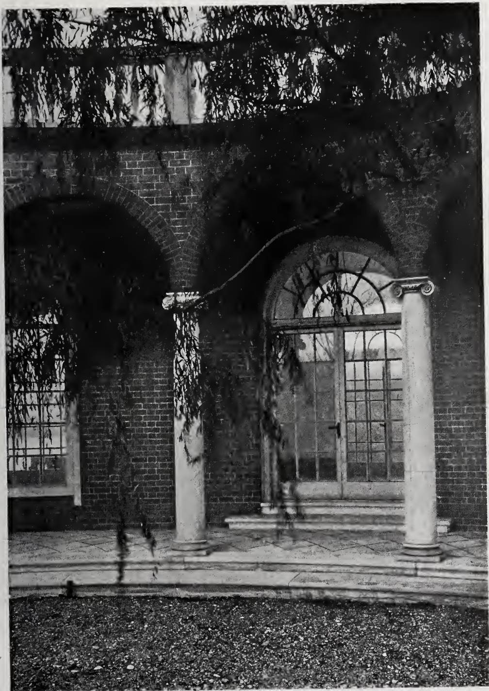
DETAIL OF CURVED PORCH—RESIDENCE OF LATHROP BROWN, ESQ., ST. JAMES, LONG ISLAND, N. Y. PEABODY, WILSON & BROWN, ARCHITECTS.
