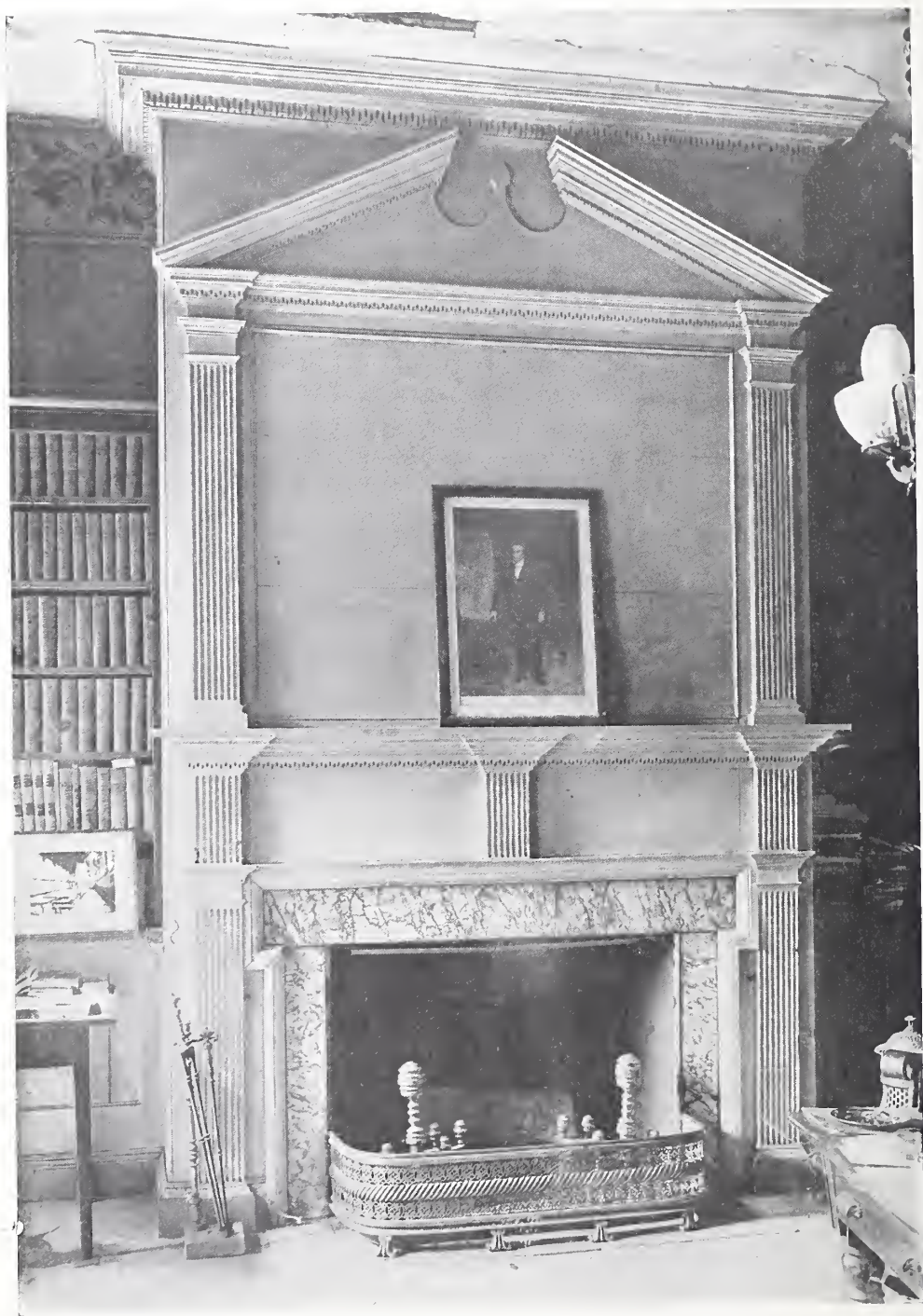
MANTELPiece ON FIRST FLOOR OF EPHRAIM BLAINE HOUSE, CARLISLE, PA.
