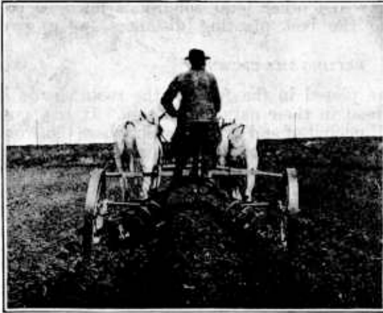
FIGURE 2.—A type of asparagus ridger used to a considerable extent in some asparagus-growing regions for renewing the ridges.
