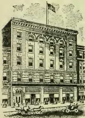
BOOK CONCERN BUILDING 5 AND 7 CITY HALL AVENUE SAN FRANCISCO
