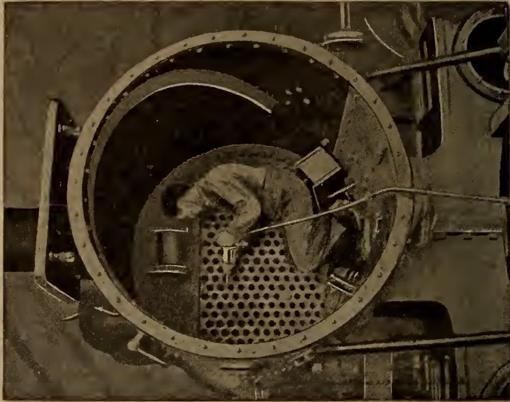
FIG. 3. Pneumatic Hammer Beading Flues—Will Bead 150 Locomotive Flues in One Hour.
