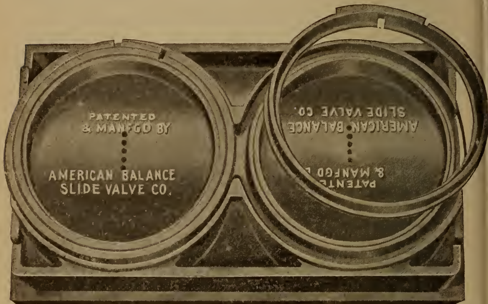
FIG. 3. Double Cone American Balance Valve.
