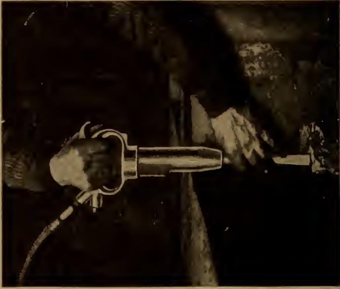
FIG. 2. Pneumatic Hammer Chipping Steel Casting.
