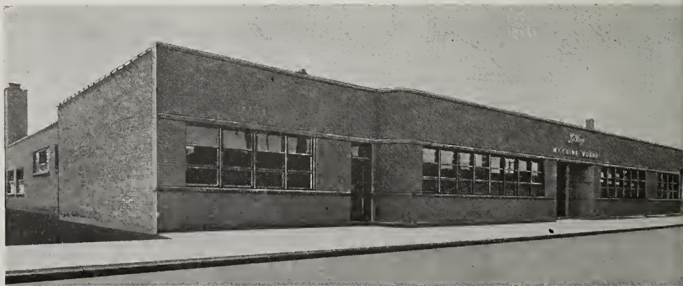
The new plant and home office building of the LaVezi Machine Works at 4635 W. Lake Street, Chicago. It was dedicated at an "open house" party attended by dealers, manufacturers and press.
