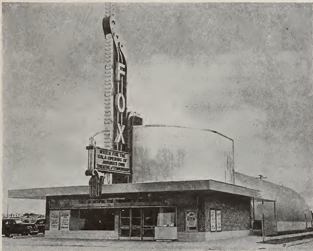
The Fox theatre in Aurora, Colo., is constructed of prefabricated sections behind a brick front structure.
