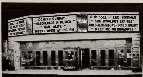
A legible arrangement of single-sized letters at the Tiffin in Chicago (above) and a layout combining large and small letters at the Sheridan in the same city, both displays representing new installations of Wagner window type panel silhouette letters.
