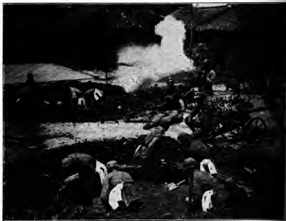
北之宅陸董在築趕之穴地空防旅九五二 Underground shelter being constructed for the defense against the air force. 去逐其將射仰兵士時防後師七十八襲來機敵 Enemy planes repulsed by our riflemen.
