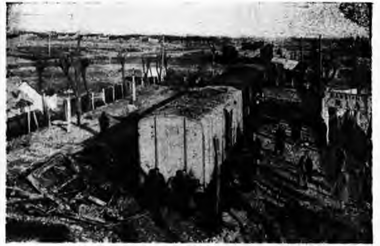
Wagons and Track at Nansiang Station Reduced to a Heap of Debris by Bombs.
