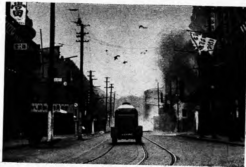
正在正北四川路鴻慶坊口 Burning Buildings in the Vicinity of Odean Theatre
