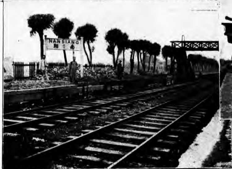
劇頗炸被站車翔南 The Nanziang Railway Station suffered great damage.
