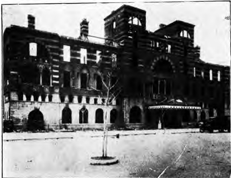
壁敗垣頽之後毀被站車火北 The North Railway Station Building after destruction by fire.
