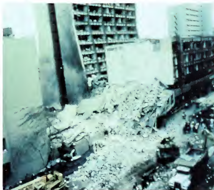
Fig. 24-2. (a) The bank building pictured was adjacent to the US embassy in Kenya before the terrorist bombing on August 7, 1998. (b) After the explosion, the same bank building (rear) has lost of most of the windows on the side closest to the explosion.
