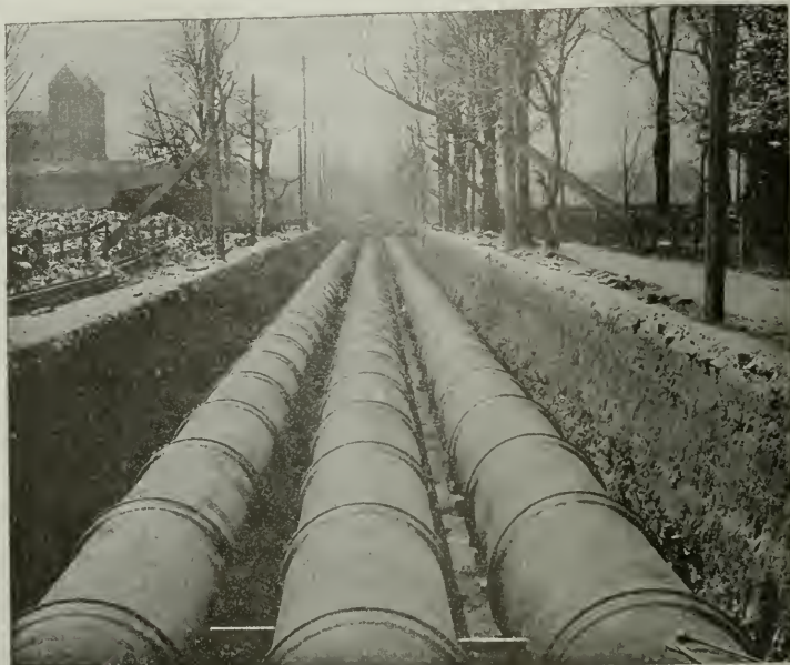
Three Lines of 60-inch Cast Iron Pipe
