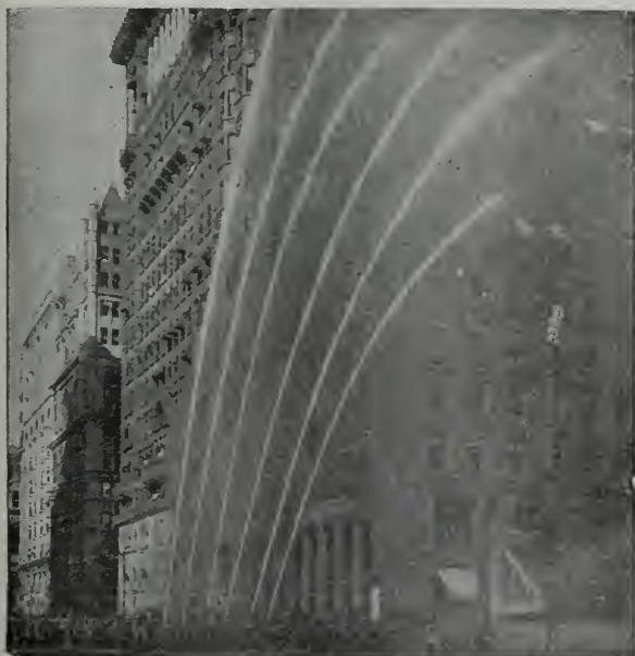
Six High Pressure Streams from One Stand
