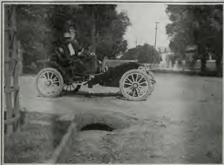
ONE OF THE MANY PART CIRCLE AMERICAN INGOT IRON CULVERTS INSTALLED IN THE CITY OF FRESNO, UNDER DIRECTION OF MR. C. P. JENSEN, CITY ENGINEER, THE MAN IN THE AUTOMOBILE
