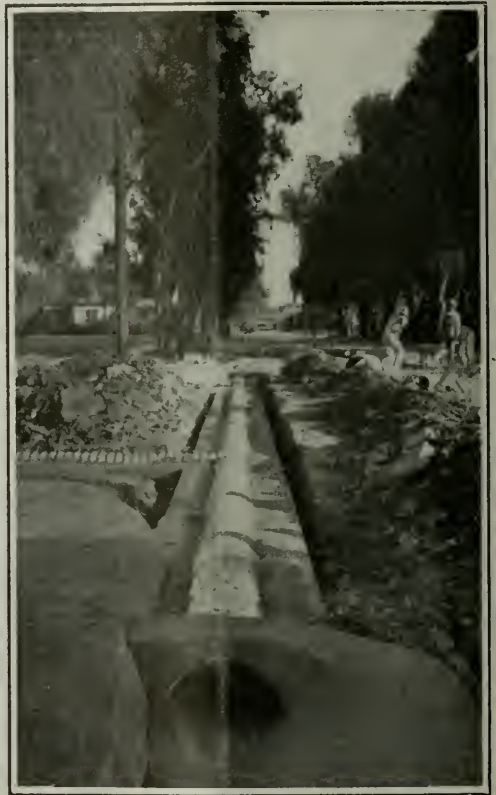
THESE PART CIRCLE AMERICAN INGOT IRON CULVERTS SHOWN AS BEING INSTALLED AT SIXTH AND LIME STREETS, RIVERSIDE, UNDER DIRECTION OF MR. A. P. CAMPBELL, CITY ENGINEER Size 14"x7", Main Culvert 68 Feet Long with Two Tees 17 ft. Each
