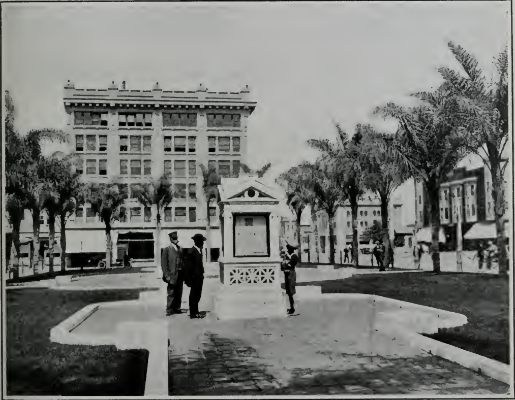
CLIMATIC KIOSK IN SAN DIEGO PLAZA
