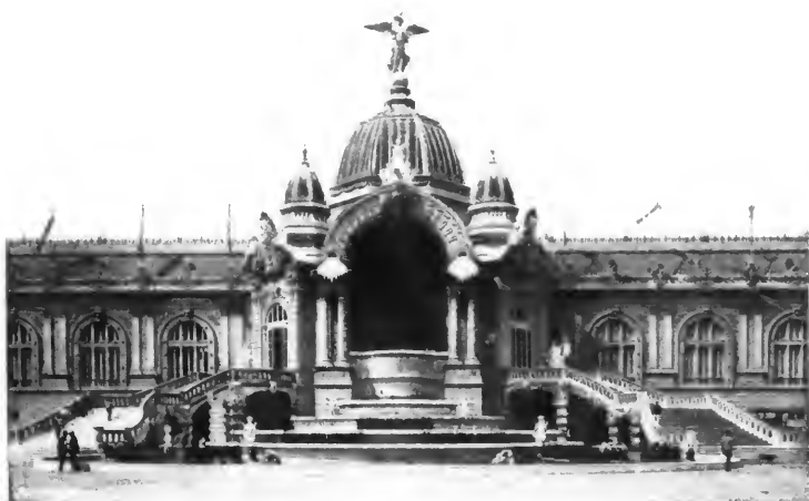
THE TEXTILE INDUSTRIES BUILDING.
