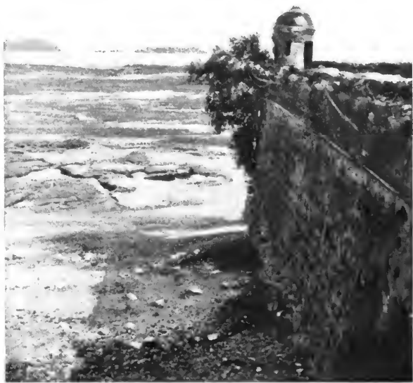
OLD SEA WALL AND WATCH TOWER OF THE CITY OF PANAMA.
