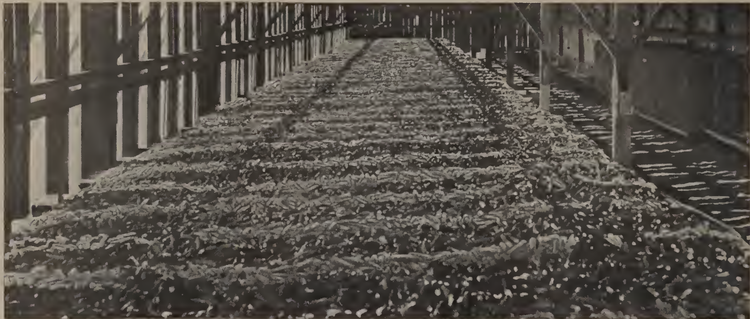
A Corn Drying Shed — Total Capacity 3,000 Bushels
