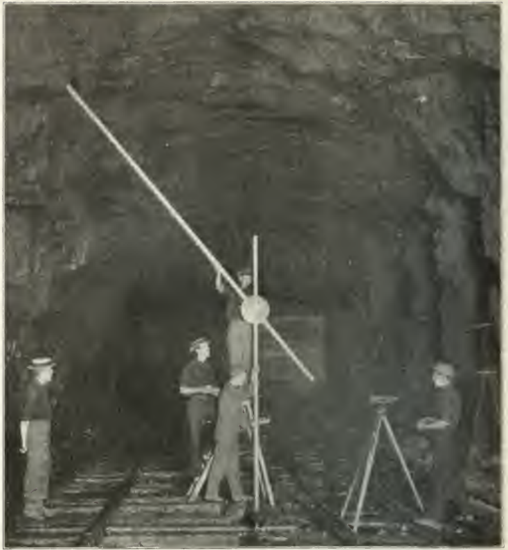
Tunnel Interior near Hackensack Portal, Showing Use of Cross Section Rod.
