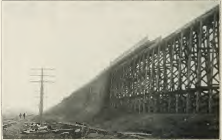
View Showing Fill, Temporary Trestle, and Old Main Line.
