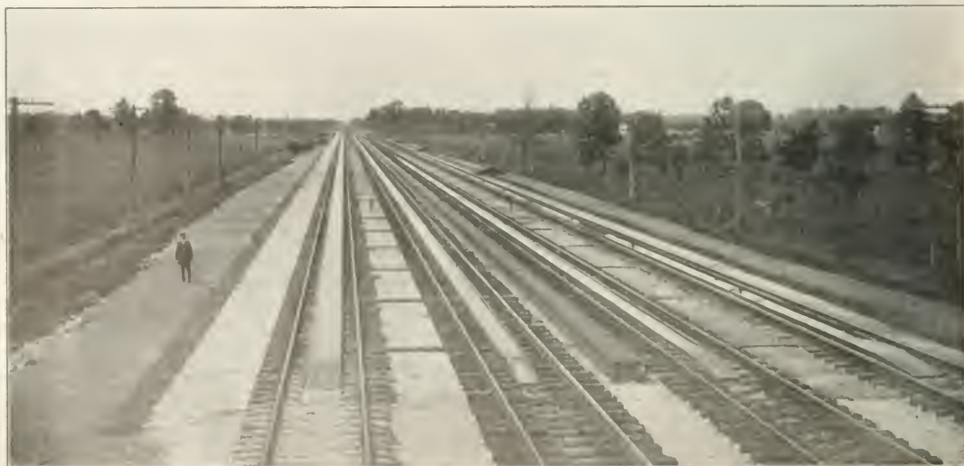
Fig. 5—Track Tanks at Springfield, Pa.; Lake Shore & Michigan Southern.
