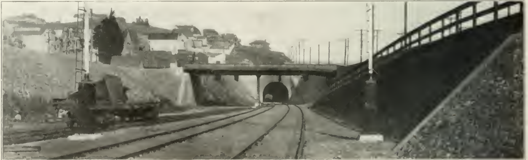
Tunnel 2; Bay Shore Cut-Off.
