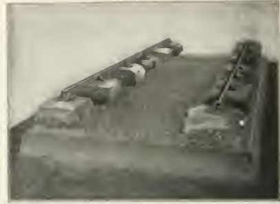
Fig. 2—Fishbelly Rails on Stone Ties; Stockton-Darlington Line, 1825.
