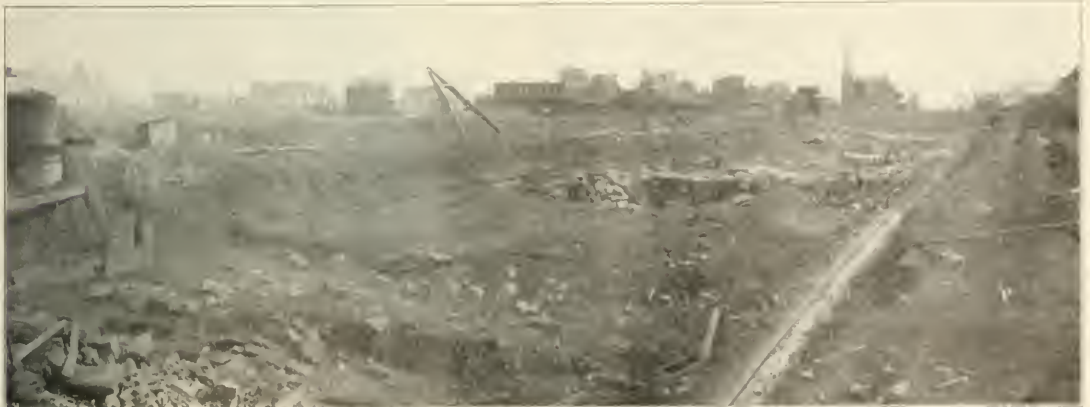
View of Open Cut from Hudson County Boulevard; Erie Terminal Improvements.
