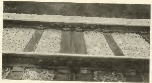
Fig. 40—Permanent Way with Rib Ties, Showing Joint Tie.
