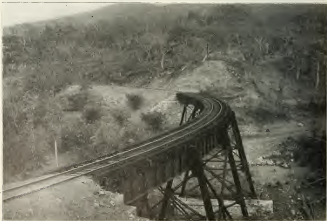
Callejon Viaduct; Guatemala Railroad.
