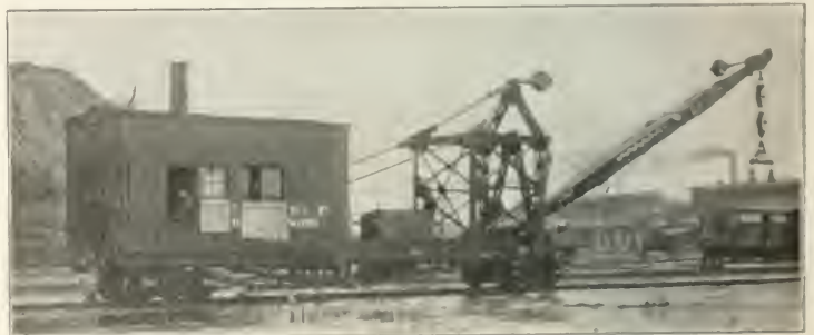
30-Ton Wooden Underframe Derrick Car; Chicago, Milwaukee & St. Paul.
