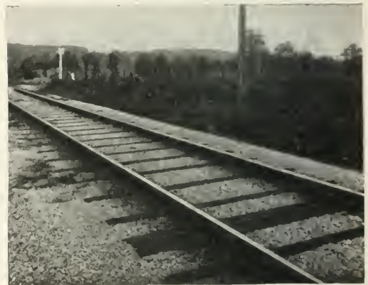
Fig. 41—Permanent Way with Rib Ties.
