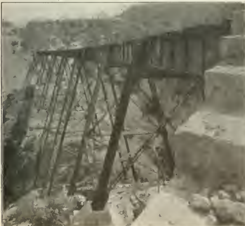
Azacuaquilla Viaduct; Guatemala Railroad.
