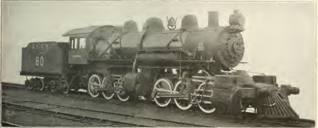
Mallet Articulated Compound Locomotive; Central Railroad of Brazil.
