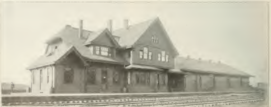
Combination Freight and Passenger Station and Division Offices; Corinth, Miss.
