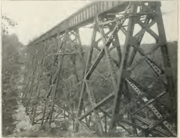
Brush Creek Viaduct; View of Structure.
