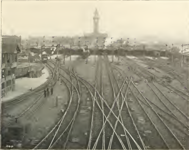
Fig. 1—General View of Hoboken Yard Looking East from Signal Bridge No. 5.
