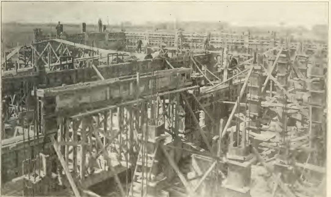
Forms for Erection of Main Building; Galesburg Timber Preserving Plant.
