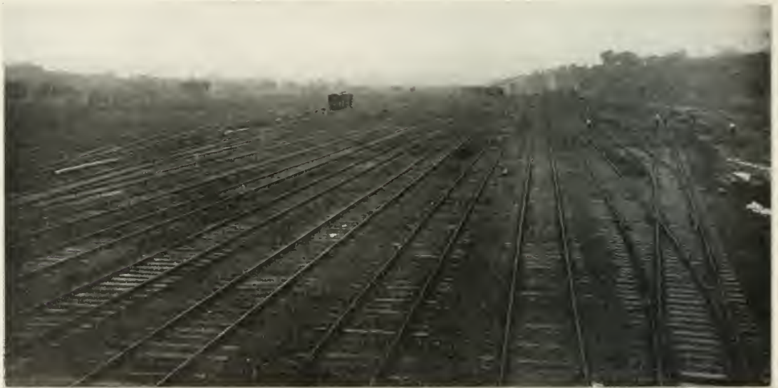
New Eastbound Classification Yard at Brunswick, Maryland; Baltimore & Ohio.
