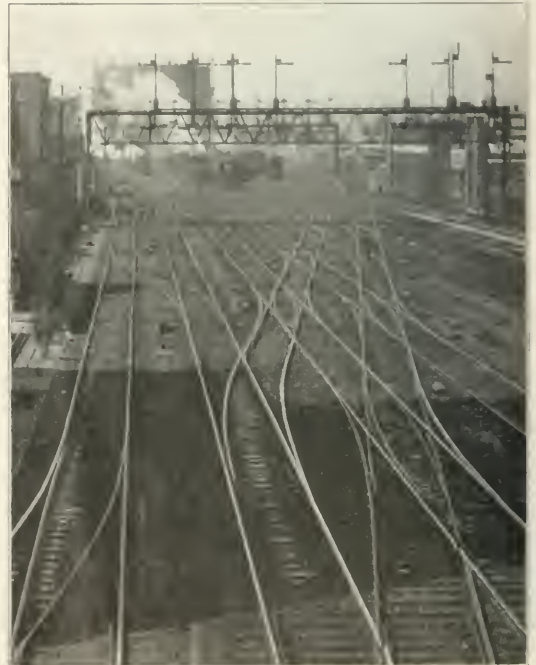
Fig. 3—Nine Tracks on Viaduct Leading to Broad Street Station, Pennsylvania Railroad, Philadelphia.
