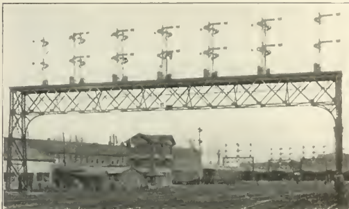
Fig. 2—Signal Bridge No. 5.
