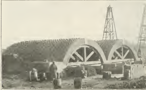
Bridge Arches Under Construction North of Soochow.
