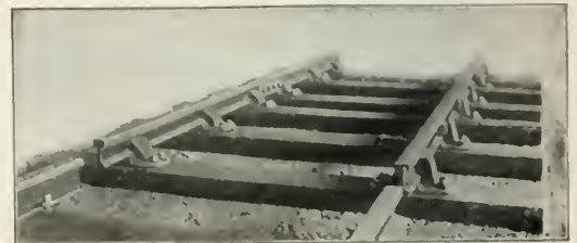
Fig. 20—Heavy Rails and Heavy Chairs on Oak Ties; Midland Railway, 1896.
