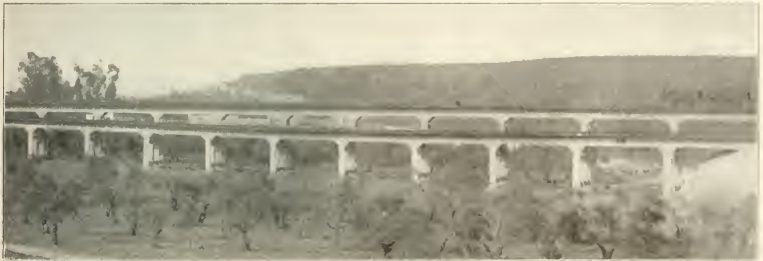
Section of Two Reinforced Concrete Viaducts Leading to Wharf of the Spanish Cala Iron Company at Seville.
