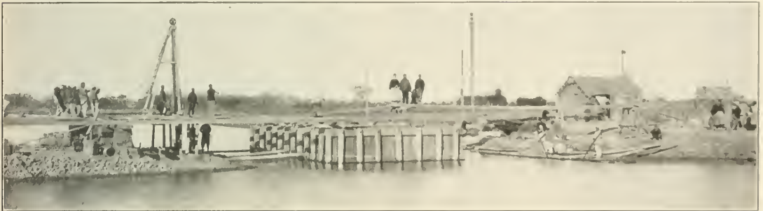
Building a Cofferdam; Shanghai-Nanking Railroad.
