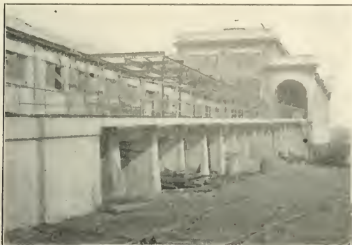
Side View of Trestle and Approach.
