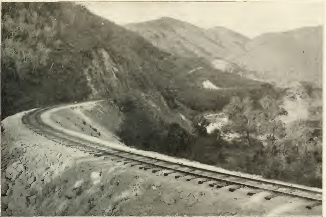
Trapich Fill; Mountain Section of Guatemala Railroad.
