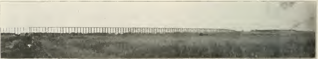
Temporary Trestle Nearly Five Miles Long; Northern Pacific Grade Revision.
