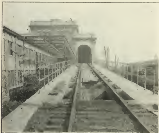
Trestle and Approach, Looking toward Power House.
