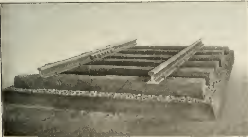
Fig. 13—Close Tie Spacing and Heavy Rails; Pennsylvania Railroad, 1895.
