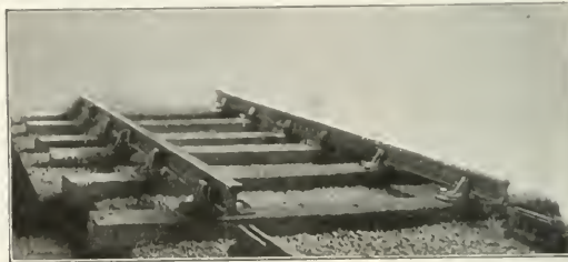
Fig. 18—Heavy Cast Iron Chairs on Fir Ties; Minden-Bückeberg Line, 1893-1903.
