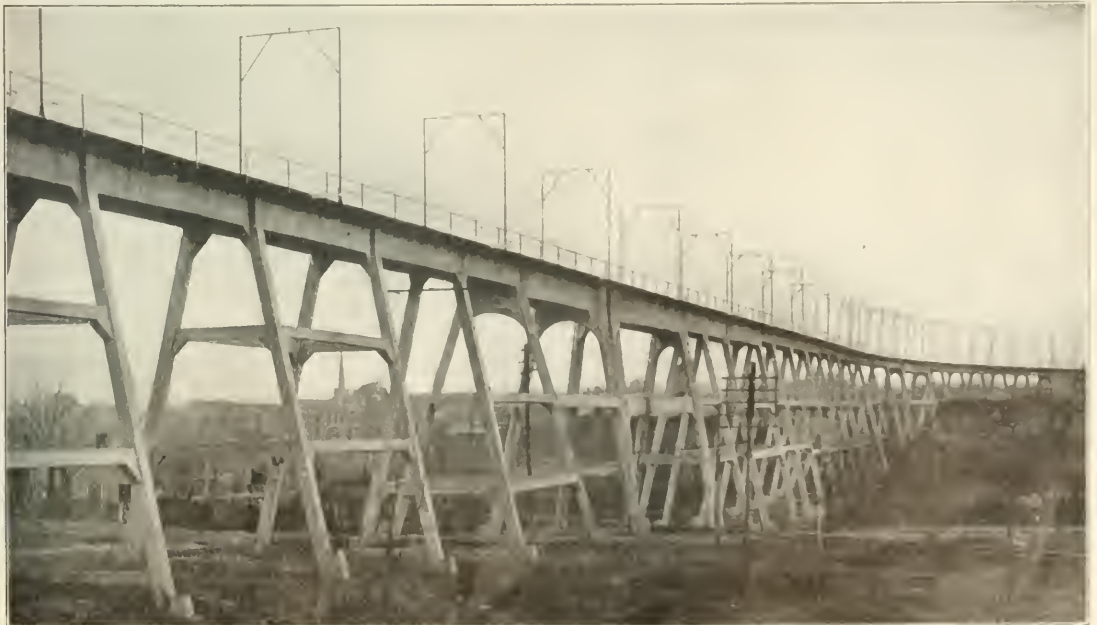
Reinforced Concrete Viaduct; Richmond & Chesapeake Bay Railway.
