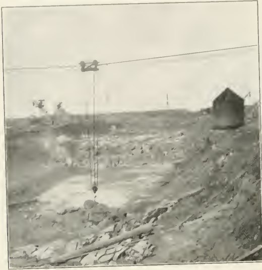
Cable Conveyors for Handling Excavated Material. Location of present tunnel shown by ventilator.
