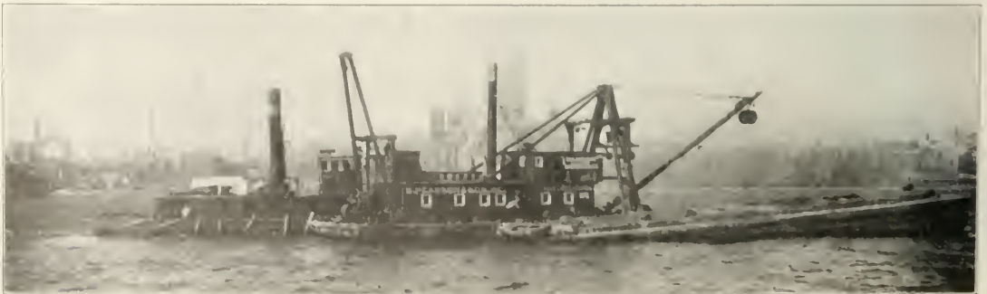
Floating Equipment—Dredge, Tug and Scow.
