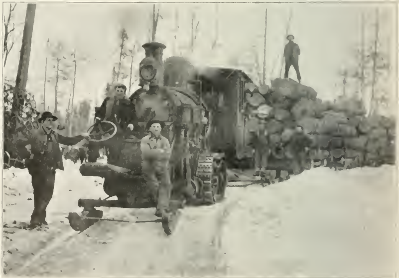
Locomotive Sled for Hauling Logs on Ice Roads.
