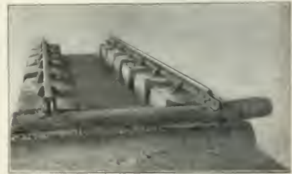
Fig. 4—Chair Rails on Stone Ties; Bavarian Railroads, about 1850.
