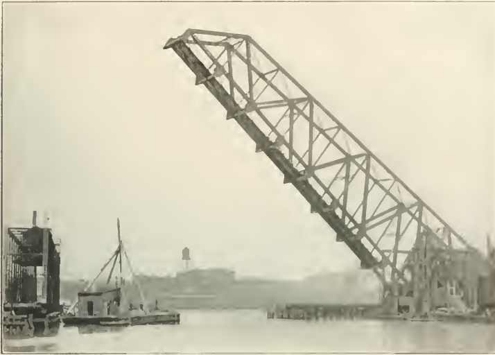
Side View of 230-ft. Scherzer Bridge in Cleveland, Under Construction.
