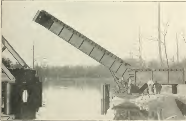
Strauss Bascule Bridge, Underneath Counterweight Type; St. Louis, Iron Mountain & Southern.
