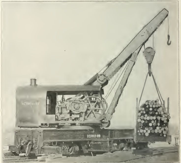
Steam Wrecking Crane; Shaw Electric Crane Company.
