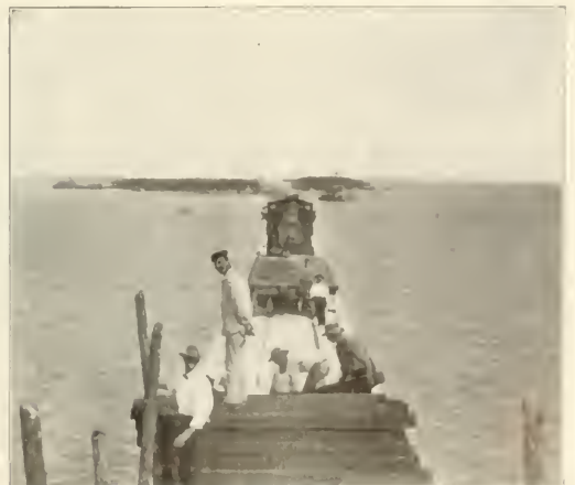
Work Train on Ocean Viaduct.
