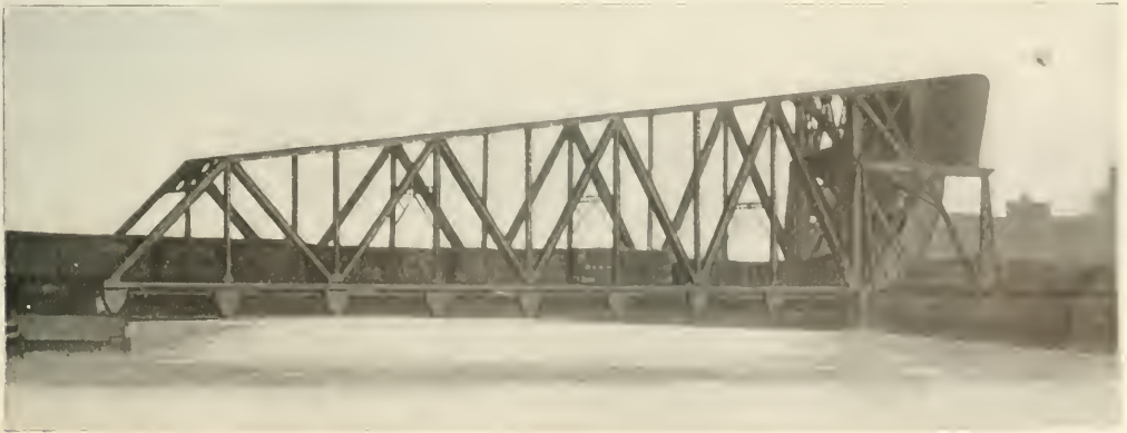
Scherzer Bridge in Closed Position.
