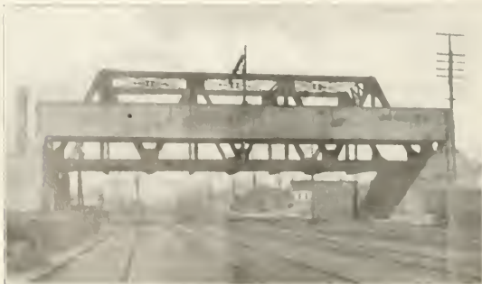
Chicago Junction Railway and Elevated Railroad Bridges Over Lake Shore and Rock Island Tracks.
