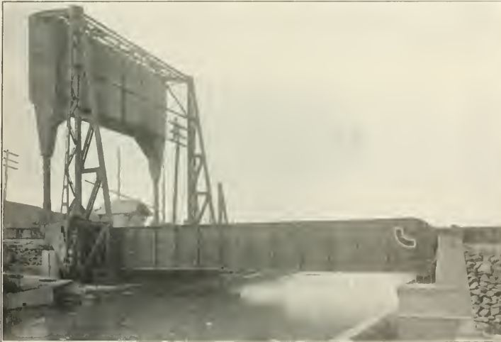
Strauss Bascule Bridge, Overhead Counterweight Type; Staten Island Rapid Transit.
