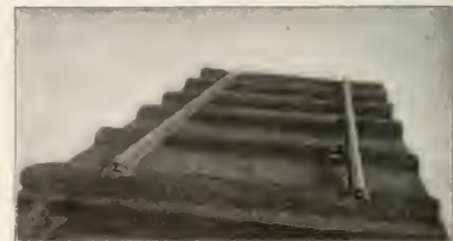
Fig. 5—Broad-Flange Rails on Wooden Ties; Leipzig-Dresden Line, 1838.
