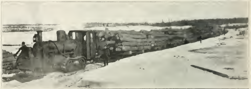
Traction Engine for Ice Roads Hauling String of Log Sleds.
