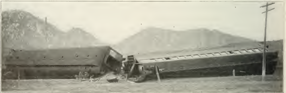
Derailment of a Passenger Train by Wind Near Marshall, Colorado.
