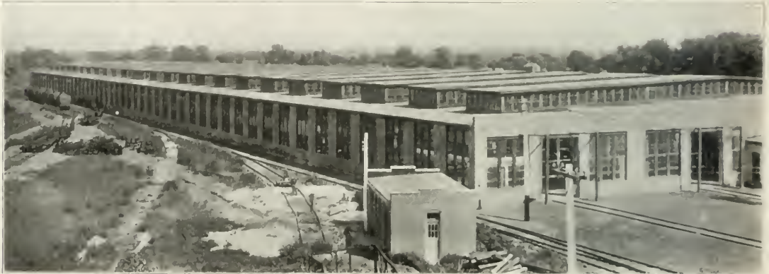
New Freight Car Repair Shop at Topeka; Atchison, Topeka & Santa Fe.
