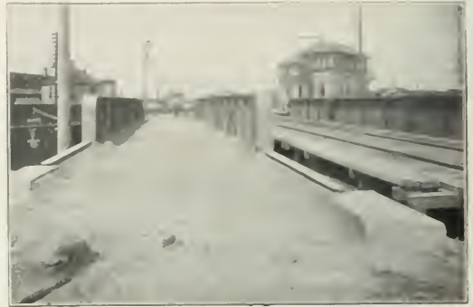
Junction Avenue Bridge of the Wabash, Detroit, Mich.
