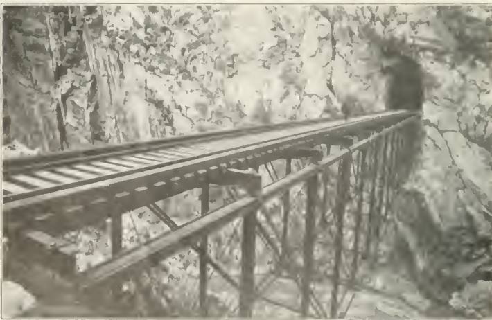
Infernillo Bridge and Tunnel 32, Elevation 10,920 ft.; Peruvian Central.
