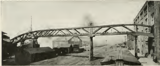
Overhead Carrier Between Warehouse and Dock.
