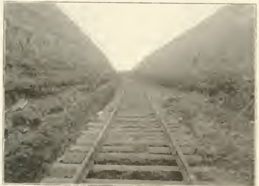
Chub Hill Cut; Alabama Western Railroad.
