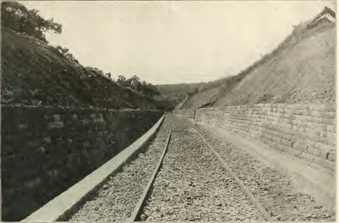
Retaining Walls and Road Bed.
