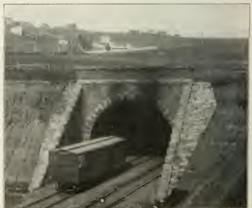
Tunnel 5; Bay Shore Cut-Off.
