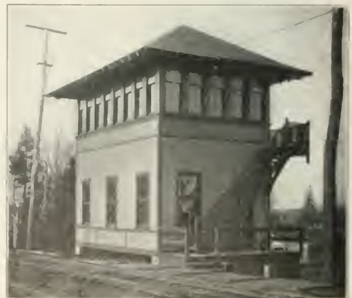
Fig. 3—Signal Cabin, Vernon, Conn.
