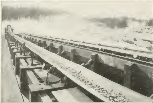
Conveyors over Storage Bins.
