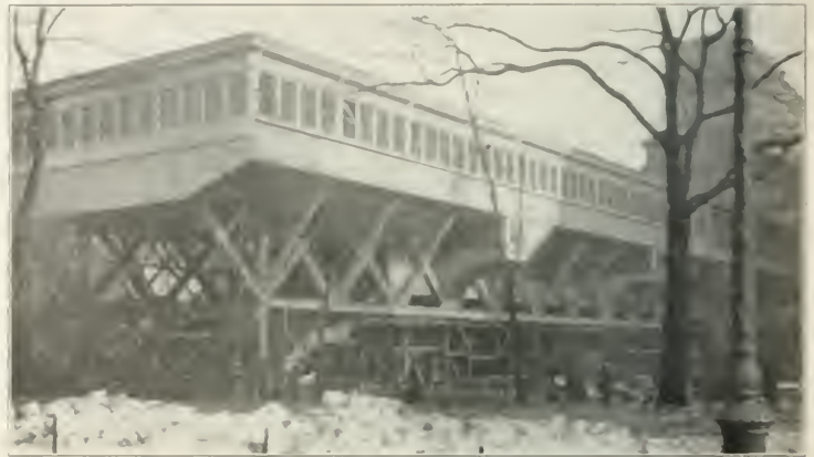
New Extension of Manhattan Terminal of Brooklyn Bridge.
