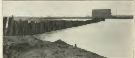
View of Dike Before Tops of Piles Were Cut Off.
