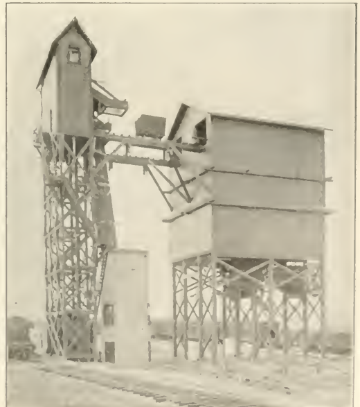
Coaling Plant at Vaughn, N. Mex.; Belen Cut-Off.
