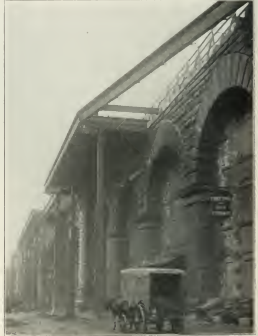
Widening of Manhattan Approach.
