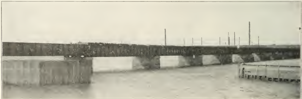
Raritan River Bridge; New Deck Girders.
