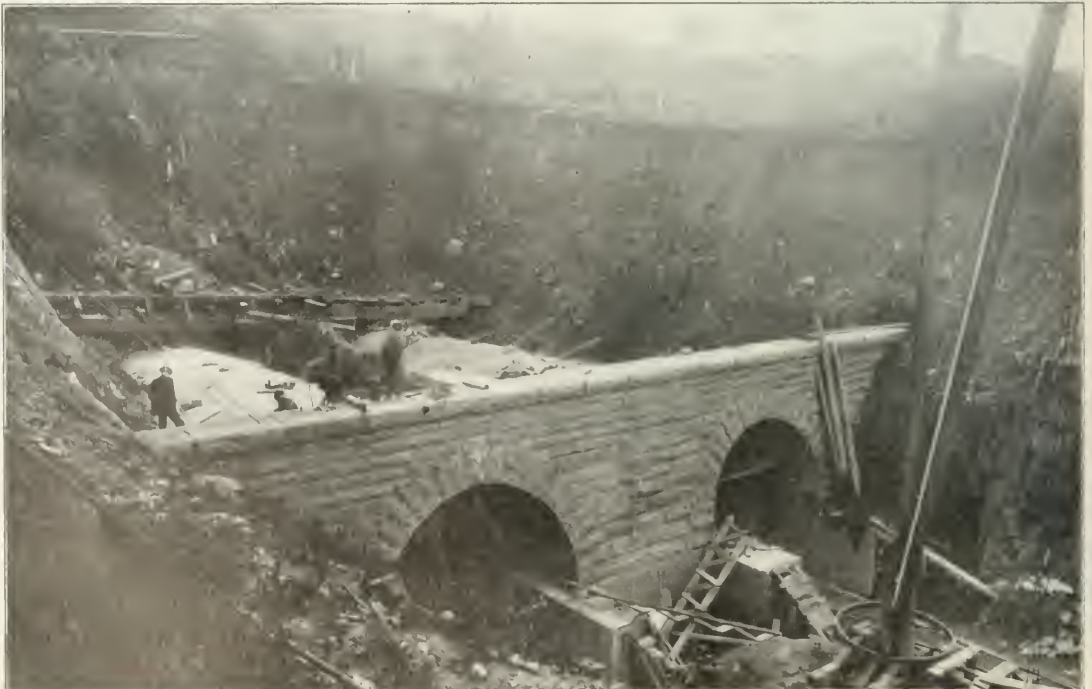
Hackensack Portal of Bergen Hill Tunnels, Looking East and Showing Arches of Cut-and-Cover Section; Pennsylvania Railroad.
