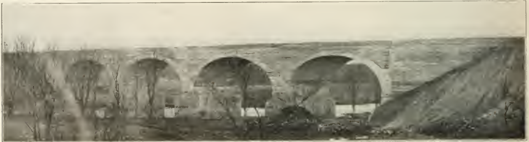
Reinforced Concrete Bridge over the Sangamon River; Wabash Railroad.
