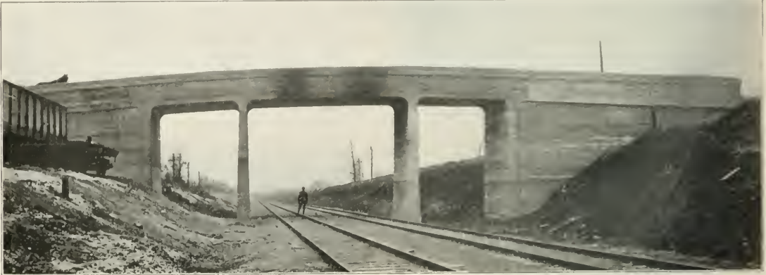
Overgrade Crossing near Seelyville, Ind.; Vandalla Railroad.
