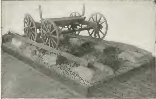
Fig. 1—Cast Iron Rails on Stone Blocks at Merthyr Tydfil, Wales, 1804.
