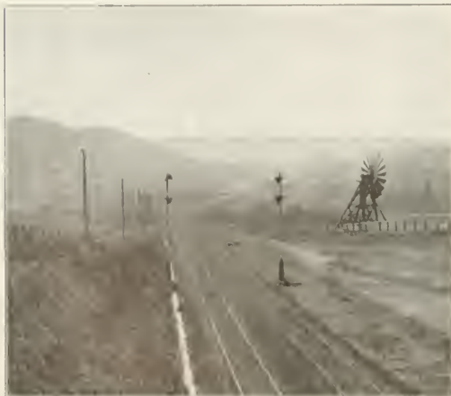
Track from Tunnel 4; Bay Shore Cut-Off.
