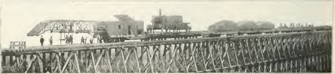
Hurley Track-Laying Machine on the Chicago, Cincinnati & Louisville.
