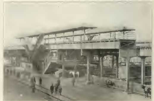
Elevated Station in Stock Yards; Chicago Junction.
