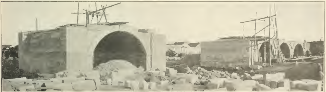
Bridge Arches Under Construction South of Soochow.
