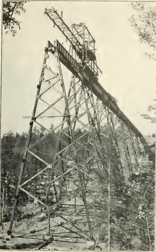
Brush Creek Viaduct, Showing Traveler.
