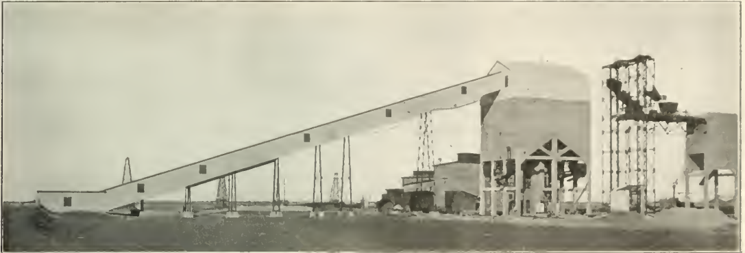
Coaling and Cinder Plant at Clovis, N. Mex., on Belen Cut-Off of the Atchison, Topeka & Santa Fe.
