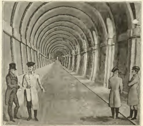
Western Archway of Tunnel, Lighted by Gas.
