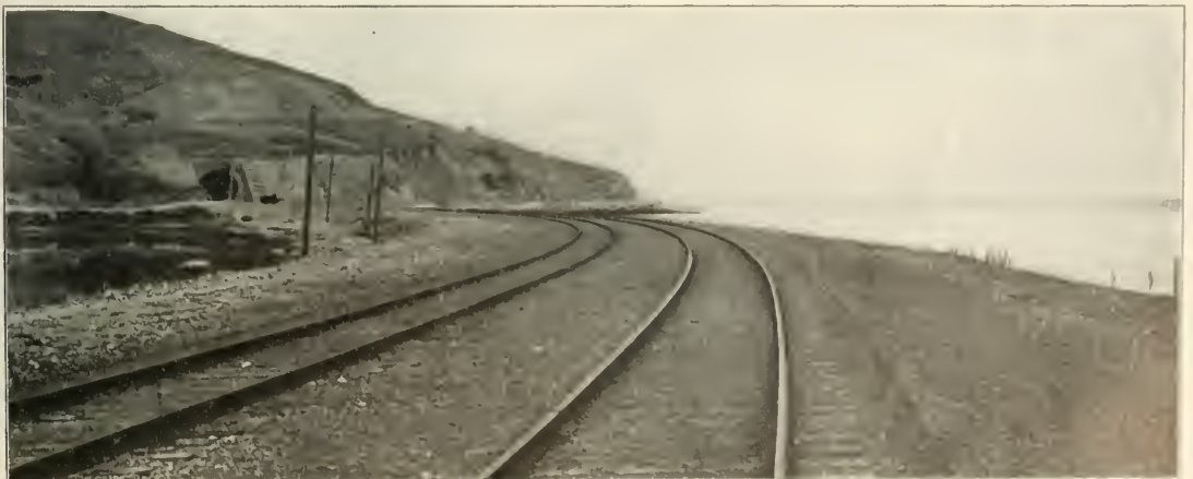
Tracks and Tunnel 6; Bay Shore Cut-Off.
