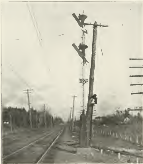
Fig. 1—Special Semaphore for East Hartford-Vernon Line.
