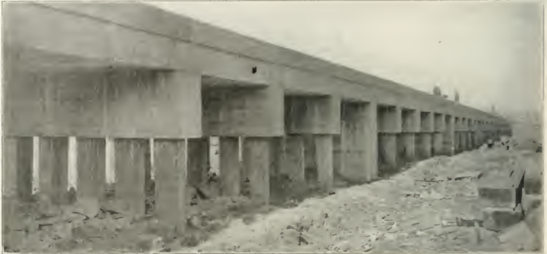
Reinforced Concrete Trestle Approach to Salt River Bridge.
