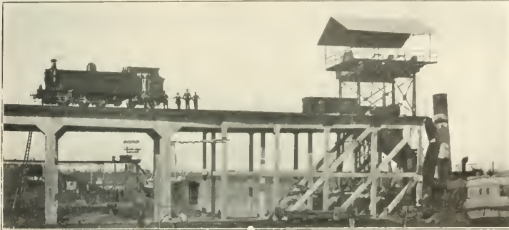
Reinforced Concrete Wharf With Car Dumper at Seville, Spain. Second wharf and viaduct in left background.
