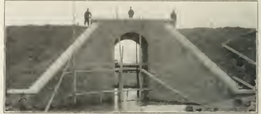
Small Bridge Near Soochow.
