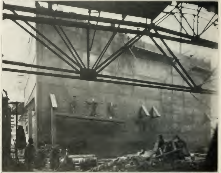
One of the Caissons at Long Island City.
