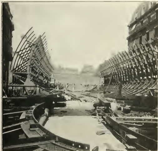
The Large Central Caisson Being Mounted.
