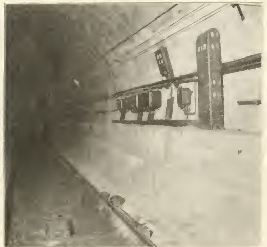
Fig. 7—Signal No. 312 and Accessories.
