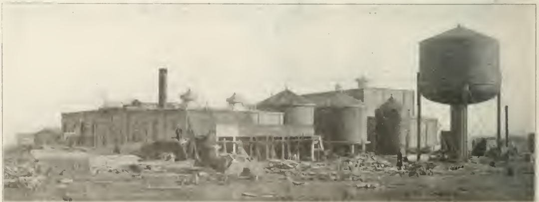
New Timber Preserving Plant at Galesburg, Ill.; Chicago, Burlington & Quincy.
