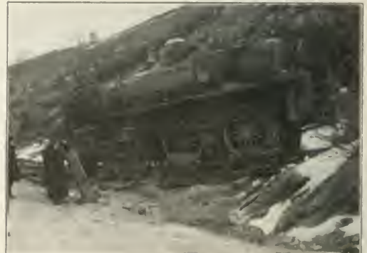
Locomotive at Foot of Plane after Having Been Pulled Along Highway. Telegraph Pole Marked "X" Shows Where Derailment Occurred.
