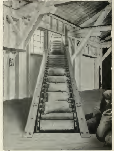
Dock End of Overhead Carrier.
