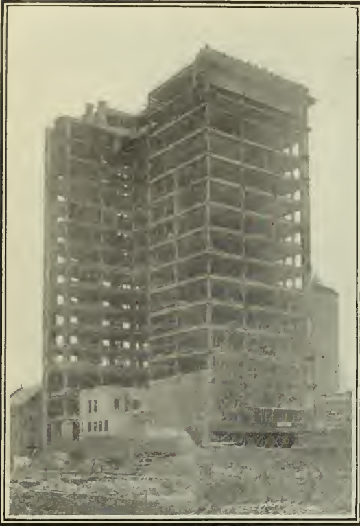
THE SKELETON OF A FIRE-SWEPT BUILDING, FROM WHICH THE EXTERIOR WALLS WERE TORN AWAY.
