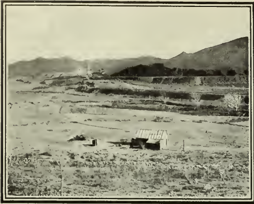
HIGH-LINE CANAL OF THE TRUCKEE-CARSON PROJECT.
