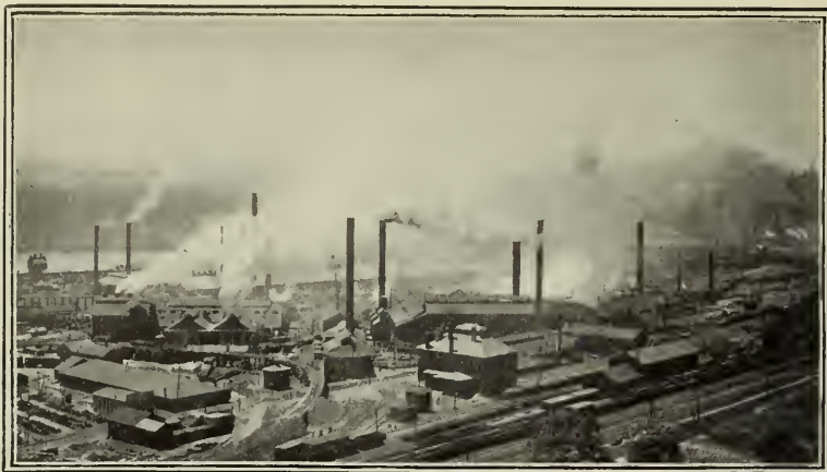
THE EDGAR THOMSON STEEL WORKS.
