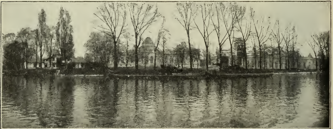
THE EXHIBITION BUILDINGS AT LIÈGE.
