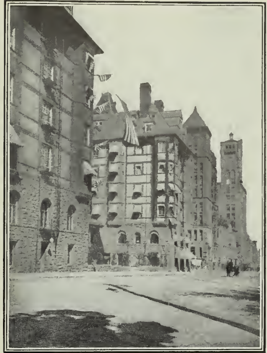
SIXTH STREET, PORTLAND, SHOWING OFFICE BUILDINGS.
