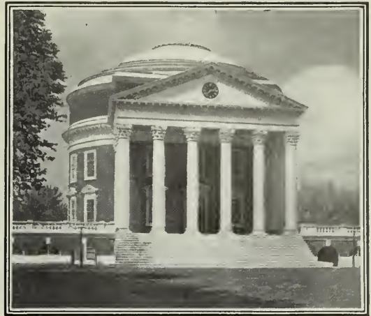
THE ROTUNDA, AS REBUILT AFTER THE FIRE OF 1895.
