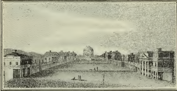
THE BUILDINGS OF THE UNIVERSITY OF VIRGINIA, AS ERECTED IN ACCORDANCE WITH JEFFERSON'S PLANS.
