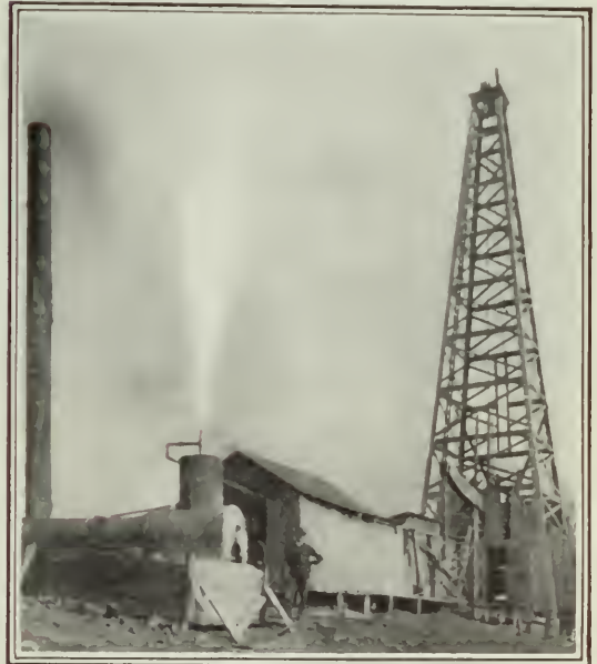
DRILLING A GAS WELL.
