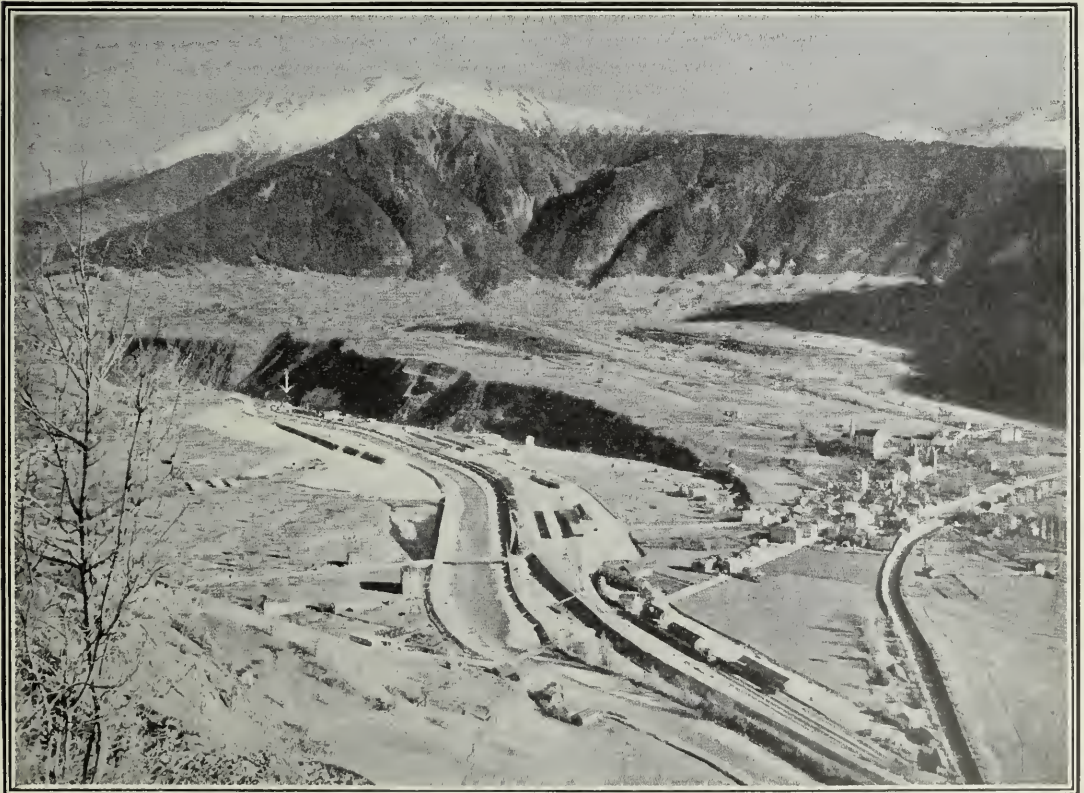
WHERE THE TUNNEL ENTERS THE SIMPLON RANGE ON THE SWISS SIDE.
