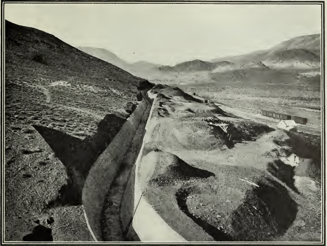
THE CEMENT-LINED CANAL OF THE TRUCKEE-CARSON PROJECT.
