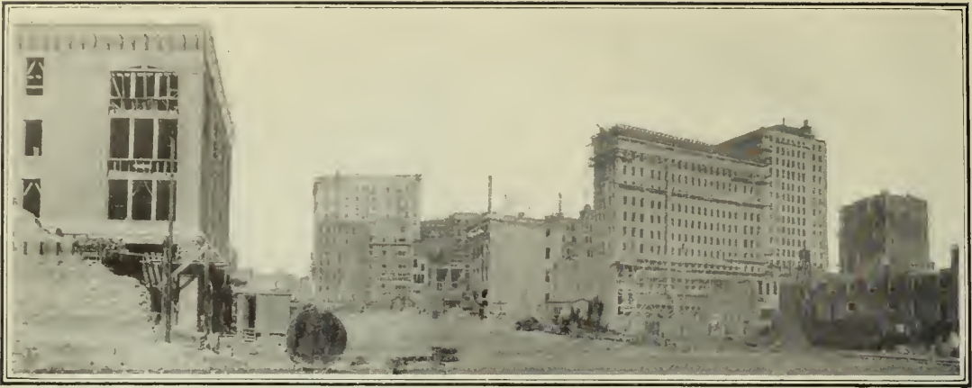
A VIEW OF THE CENTER OF THE BURNED DISTRICT, SHOWING ONE OF THE NEWLY WIDENED STREETS, NEW OFFICE AND STORE BUILDINGS, AND FIREPROOF BUILDING BEING REPAIRED.*
