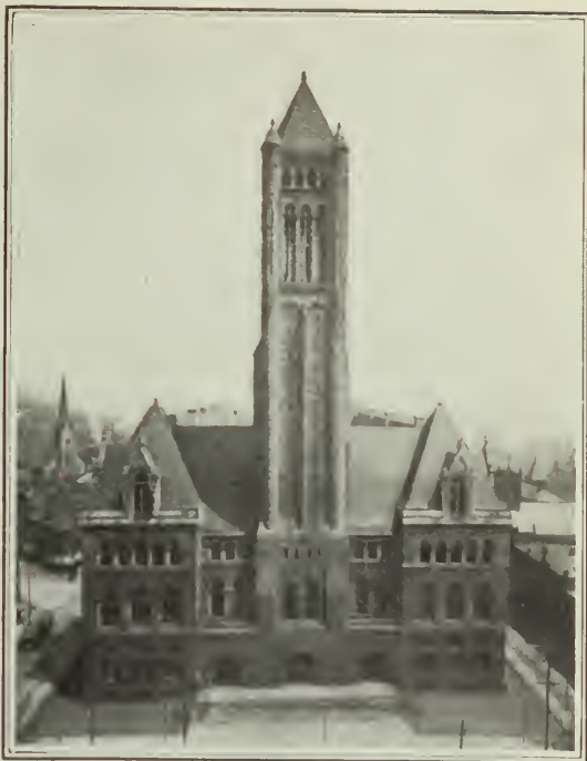
THE ALLEGHENY COUNTY COURTHOUSE.
