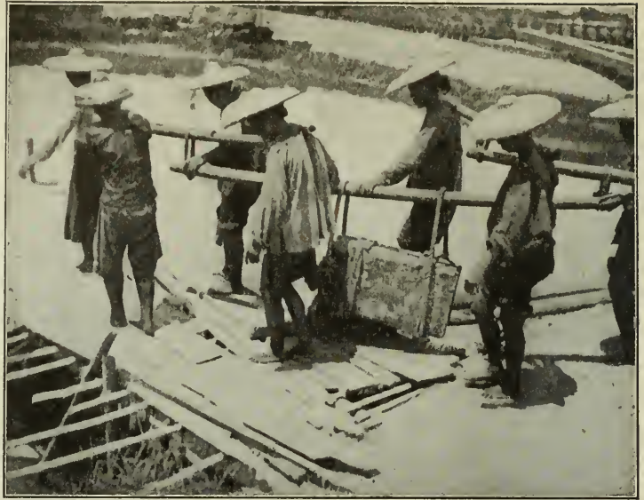
CHINESE METHODS OF MULTIPLE LEVERS IN CARRYING HEAVY LOADS.
