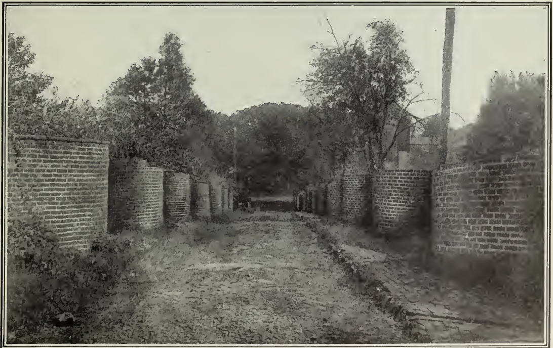
SERPENTINE WALLS (OF SINGLE-BRICK THICKNESS) PLANNED BY THOMAS JEFFERSON.
