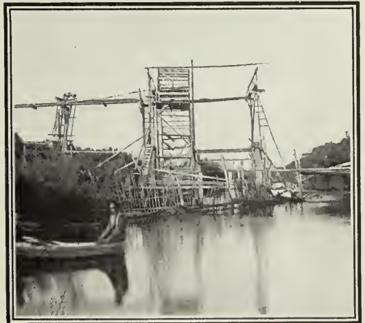
A PIONEER'S IRRIGATION PLANT.
