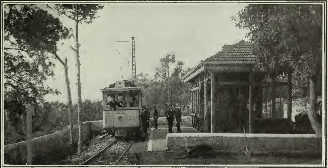
ELECTRIC CAR AND STATION ON ADHESION SECTION OF MOUNT VESUVIUS RAILWAY.
