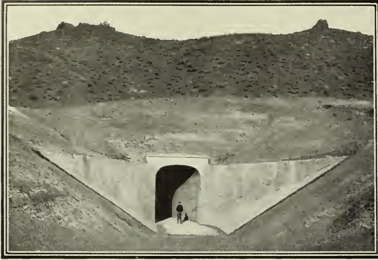
ONE OF THE NUMEROUS GOVERNMENT TUNNELS IN NEVADA.
