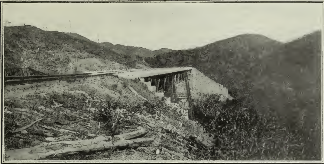
BRIDGE IN CHIVELA PASS, ON THE TEHUANTEPEC RAILWAY.
