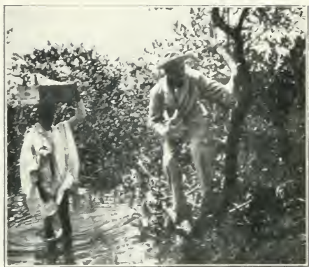
THE ROADS IN THE RAINY SEASON ARE OFTEN FLOODED.
